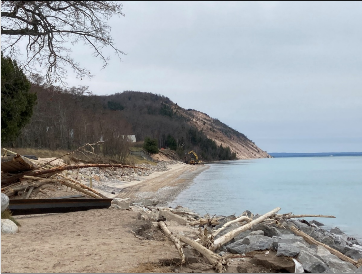
Figure 1: Revetment Construction Conditions (11/24/2020)
