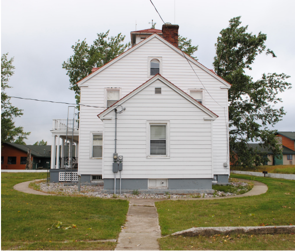
Pedestrian walks arranged symmetrically around Station Dwelling (HS-18) remain from the period of significance (source: Mundus Bishop, 2019)
