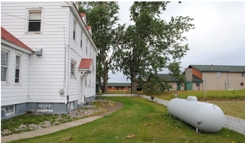
Contributing small scale features at Station Dwelling (HS-18) include a concrete wall. The propane tank, grill, and picnic table are non-contributing (source: Mundus Bishop, 2019).
