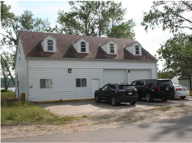
Equipment Building (source: Mundus Bishop, 2019).
