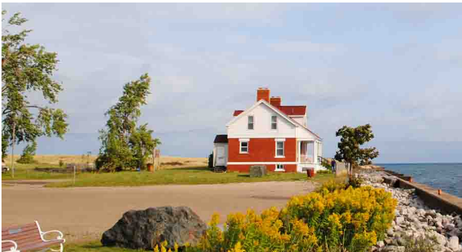
The orientation of Harbor of Refuge Dwelling (HS-20) to the navigational channel remains similar to the period of significance. A fence parallel to West Pier obscures views to the water (source: Mundus Bishop, 2019).
