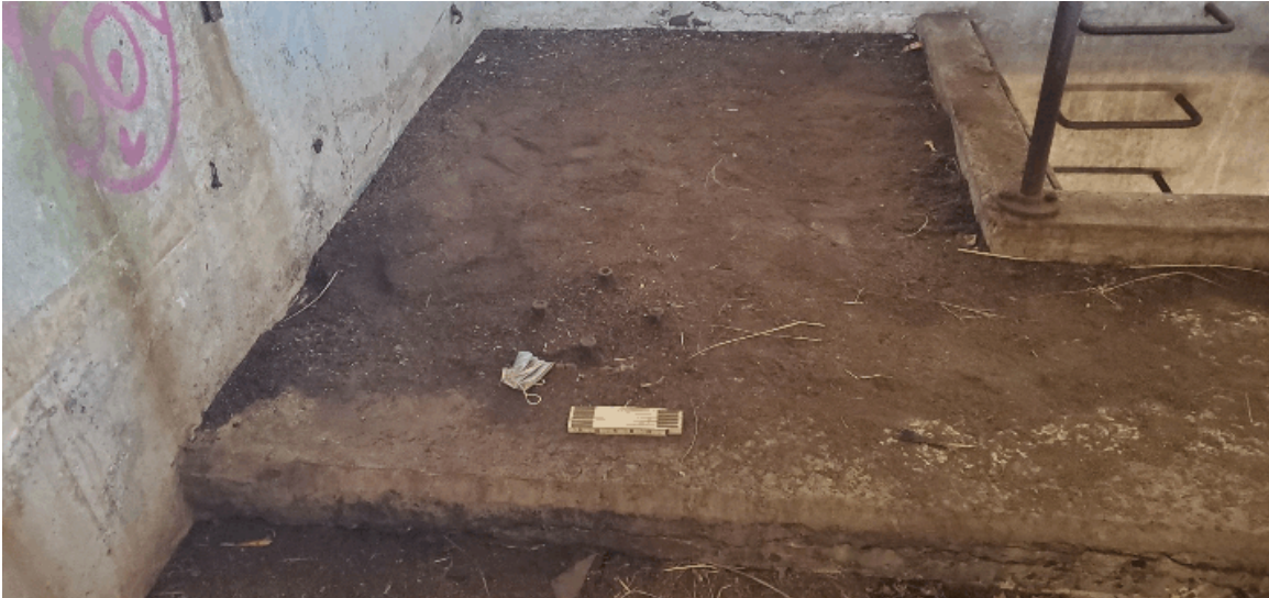
Figure 40 Interior, Miller Field Fire Control Tower, Fourth Level Showing Azimuth Instrument Base Connection (Four Bolts Above Rule), Facing Northwest (Attenborough 2022).
