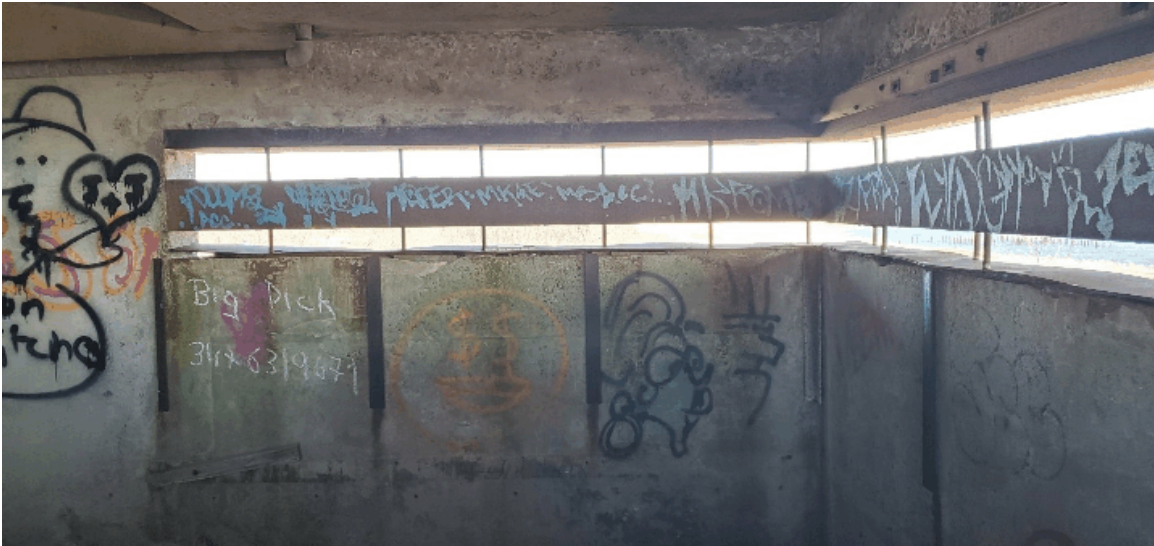
Figure 41 Interior, Miller Field Fire Control Tower, Fifth Level Instrument Observation Slits, Facing Northeast (Attenborough 2022).
