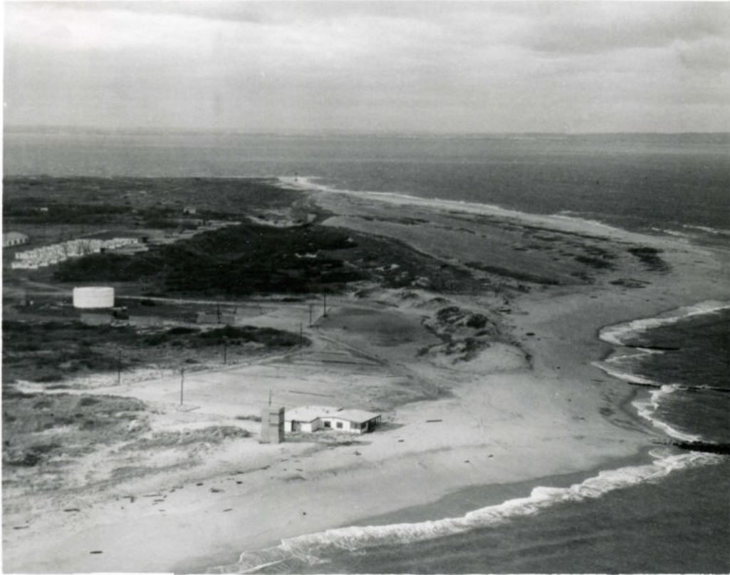
Figure 45 Image Showing Fire Control Tower at North Beach, Sandy Hook, New Jersey in 1960. Source: NPS GATE. Courtesy of Shawn Welch of AGFA.
