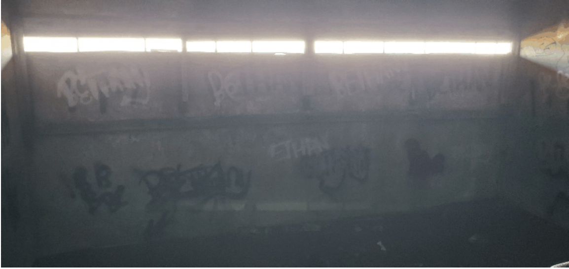
Figure 39 Interior, Miller Field Fire Control Tower, Third Level Showing Single Observation Slit, Facing Southeast (Attenborough 2022).
