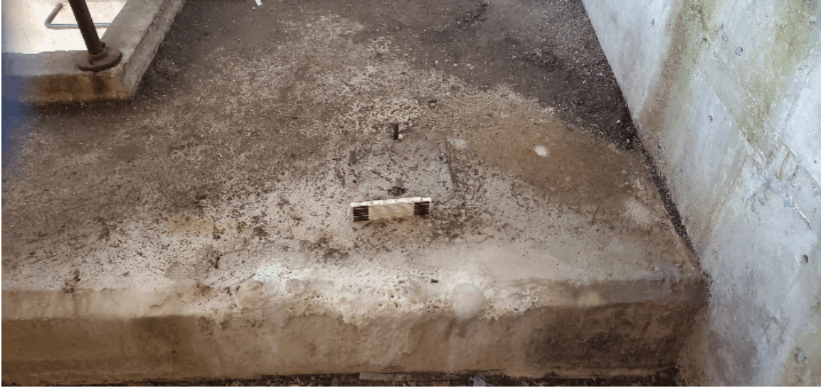
Figure 43 Interior, Miller Field Fire Control Tower, Fifth Level Showing DPF Instrument Base Connection, Facing Northwest (Attenborough 2022).
