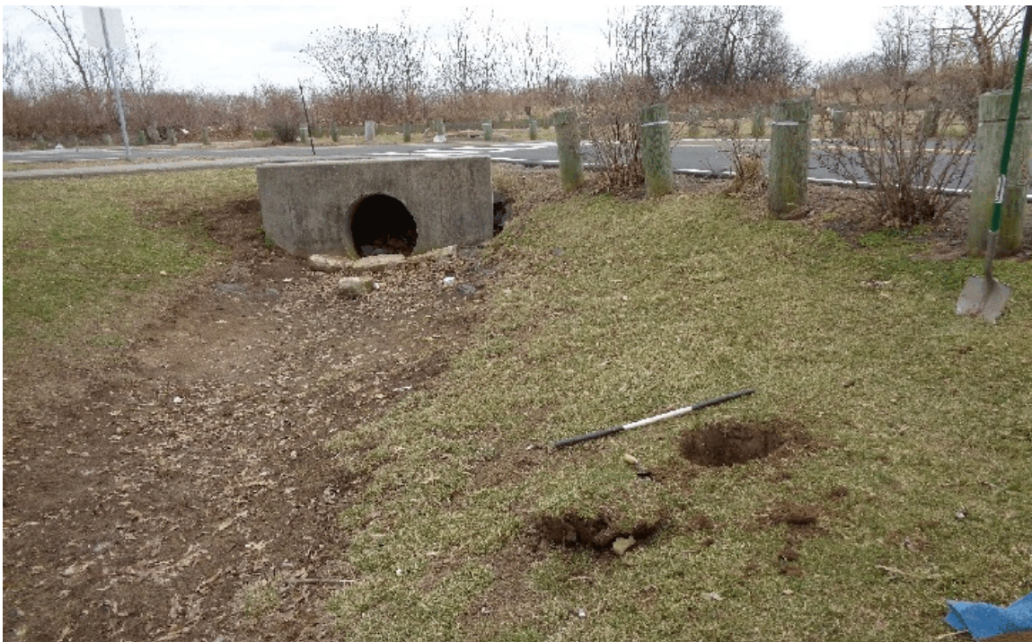
Figure 11 View of the culvert, drainage ditch and STP E20, facing east (Image 0145: March 7, 2022).
