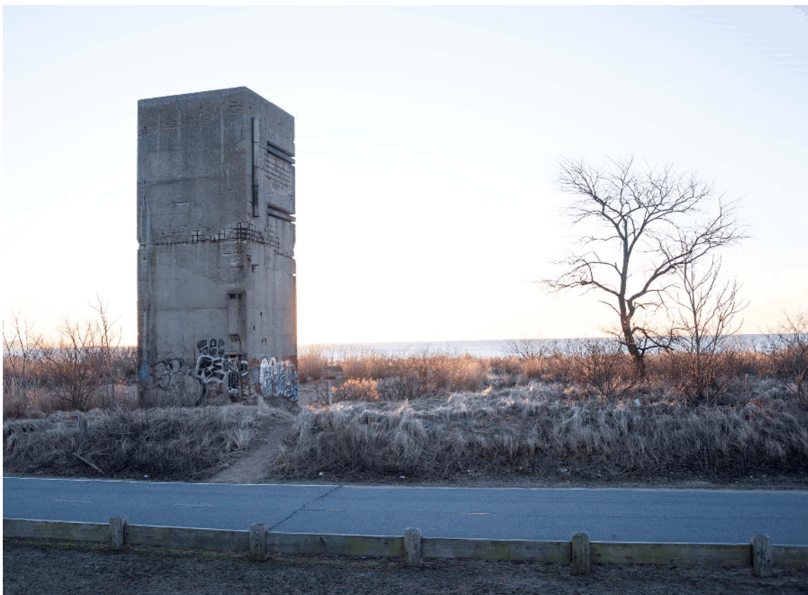
Figure 33 Miller Field Fire Control Tower, Northwest and Southwest Façades, Facing East (Attenborough 2022).
