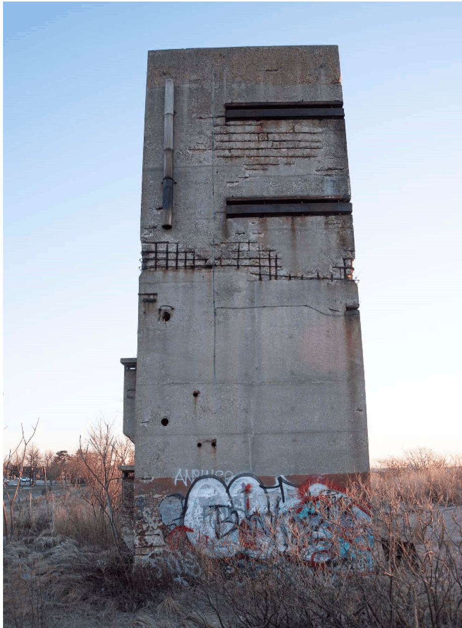
Figure 36 Miller Field Fire Control Tower, Southwest Façade, Facing Northeast (Attenborough 2022).
