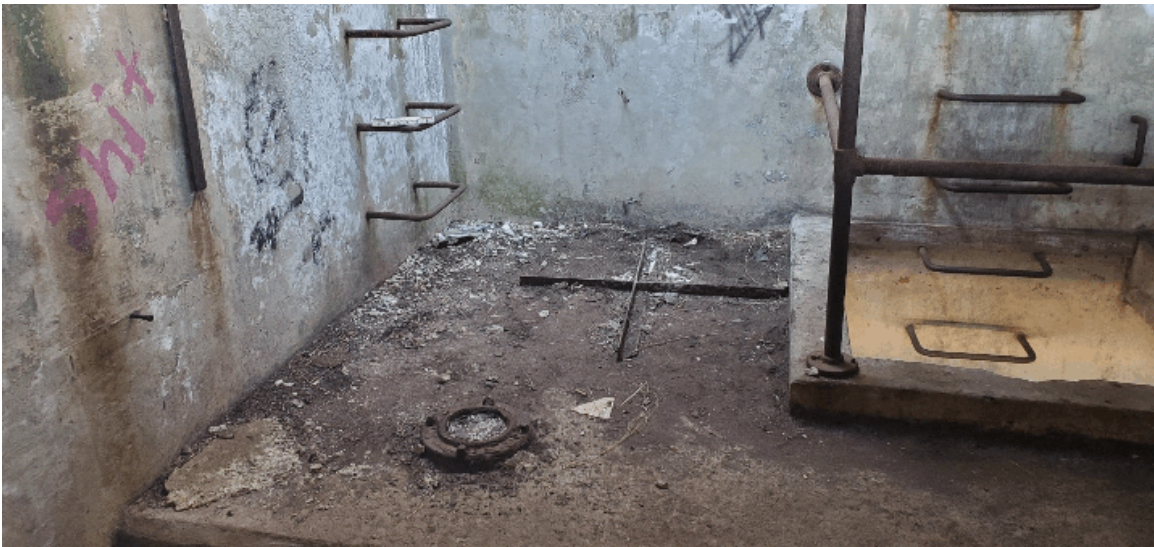
Figure 42 Interior, Miller Field Fire Control Tower, Fifth Level Showing Azimuth Instrument Base Connection (Circular Object, Lower Left), Facing Northwest (Attenborough 2022).
