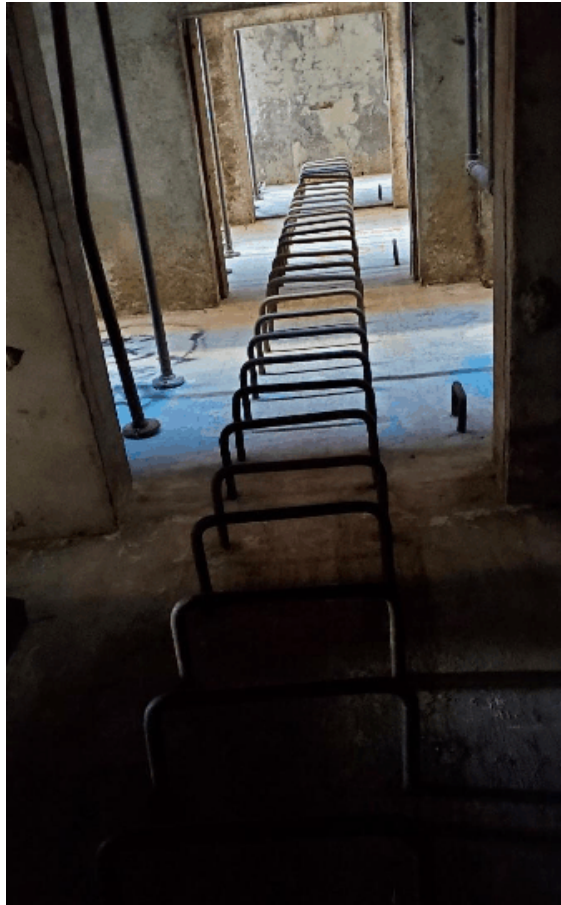
Figure 38 Interior, Miller Field Fire Control Tower, View of Ladder, Facing Northwest (Attenborough 2022).
