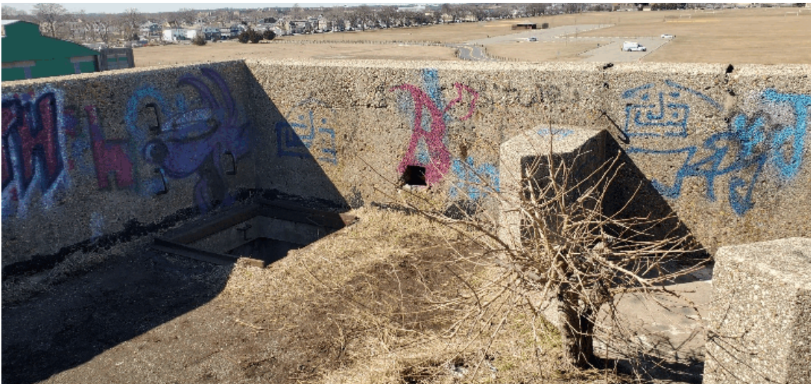
Figure 44 Miller Field Fire Control Tower, Parapet Level, Facing West (Attenborough 2022).
