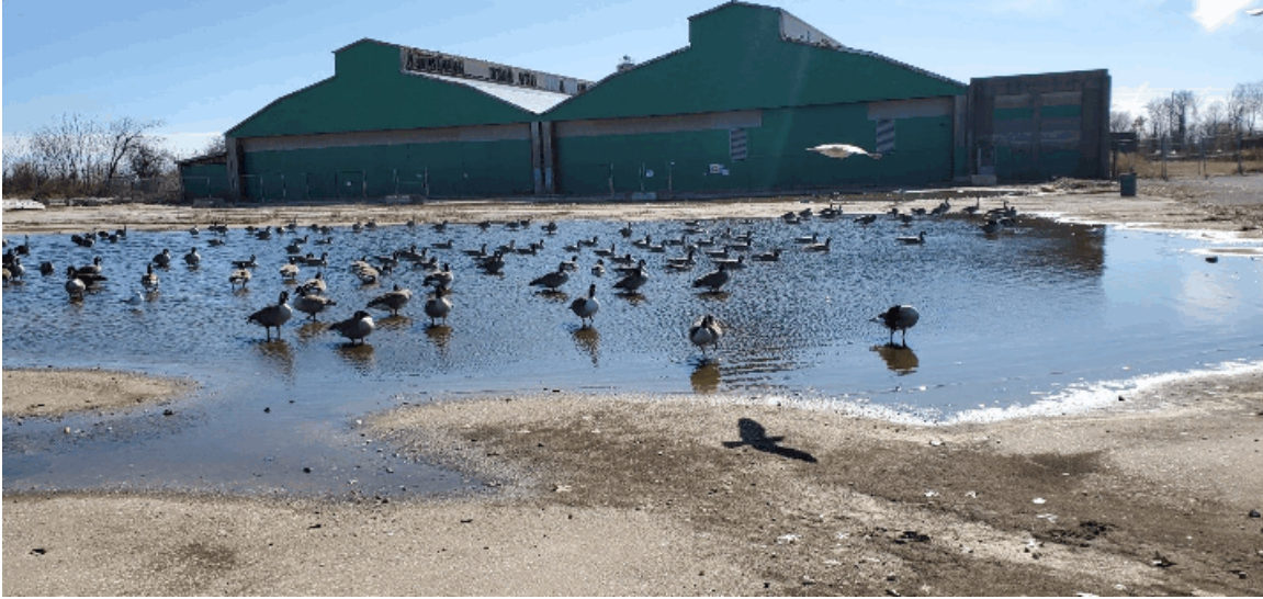
Figure 18 Concrete Apron and Seaplane Hangar 38, Facing Southwest (Stone 2022).
