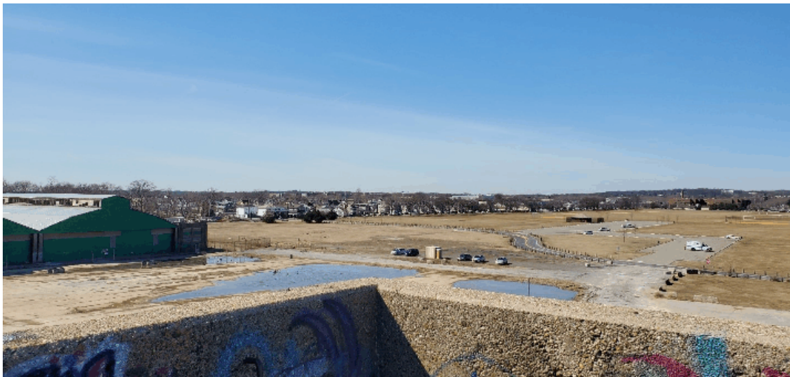
Figure 31 Concrete Apron and Seaplane Hangar 38 From Fire Control Tower, Facing West (Attenborough 2022).
