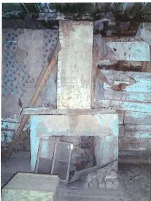
Fireplace in Room 102
