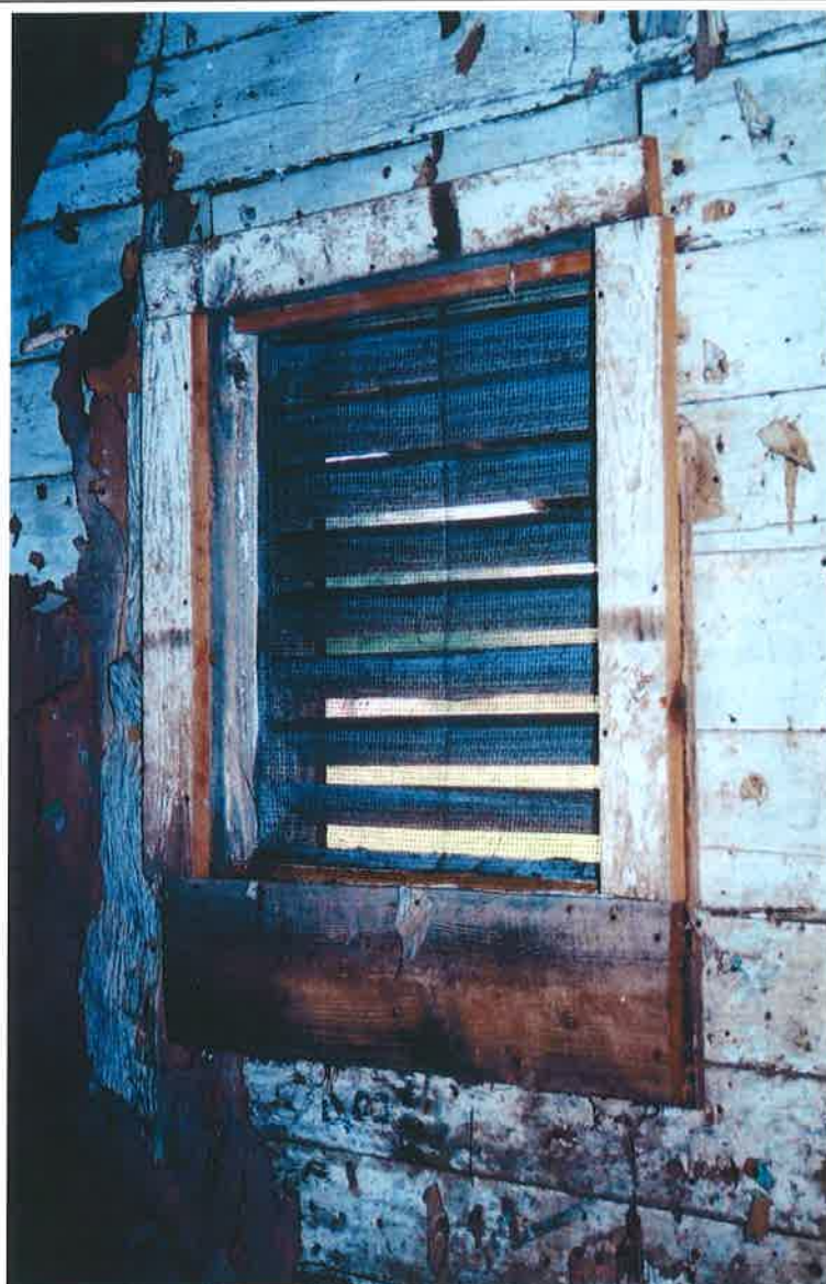
Image 84: Oakland Plantation. South Tenant Cabin, Room 103, 2002. Window surround on east wall.
