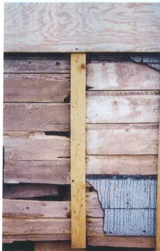
Detail of north exterior siding
