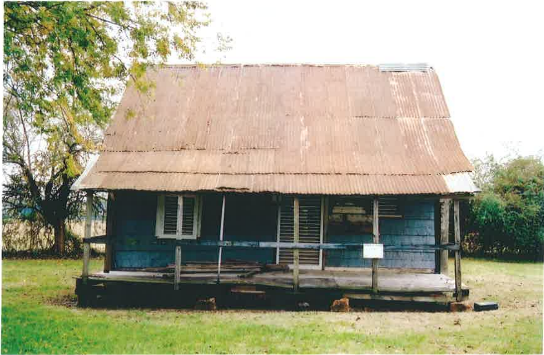
Image 66: Oakland Plantation. South Tenant Cabin, east elevation, 2002.
