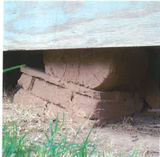
Foundation pier, main building
