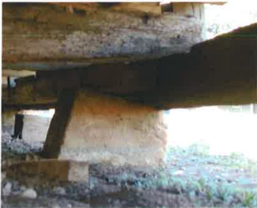
Beam at front gallery
