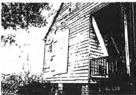
11-21. West elevation of the Main House showing the stabilized window complete.
