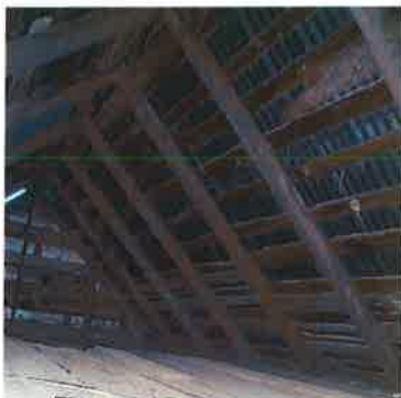
Roof framing over main building
