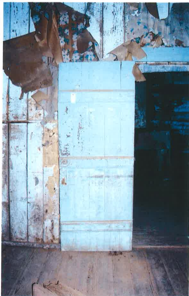
Image 78: Oakland Plantation. South Tenant Cabin, Room 102, south wall, 2002. Door D2.
