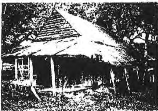
3-35. The Cook's House. Northeast elevation prior to stabilization work.
