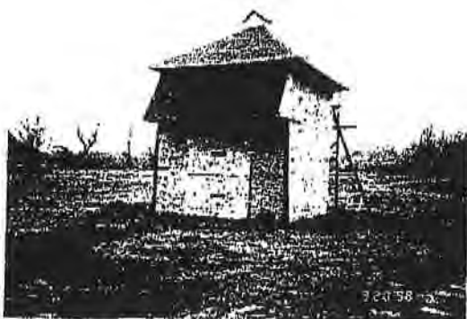
13-6. Complete West Pigeoneer. Notice asphalt, venting, and temp double doors.
