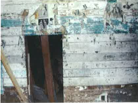
Detail of west wall of Room 103
