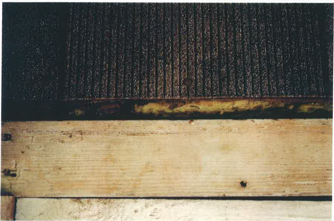
Image 74: Oakland Plantation. South Tenant Cabin, east elevation, 2002. Bousillage preserved behind sheathing and asphalt paper.
