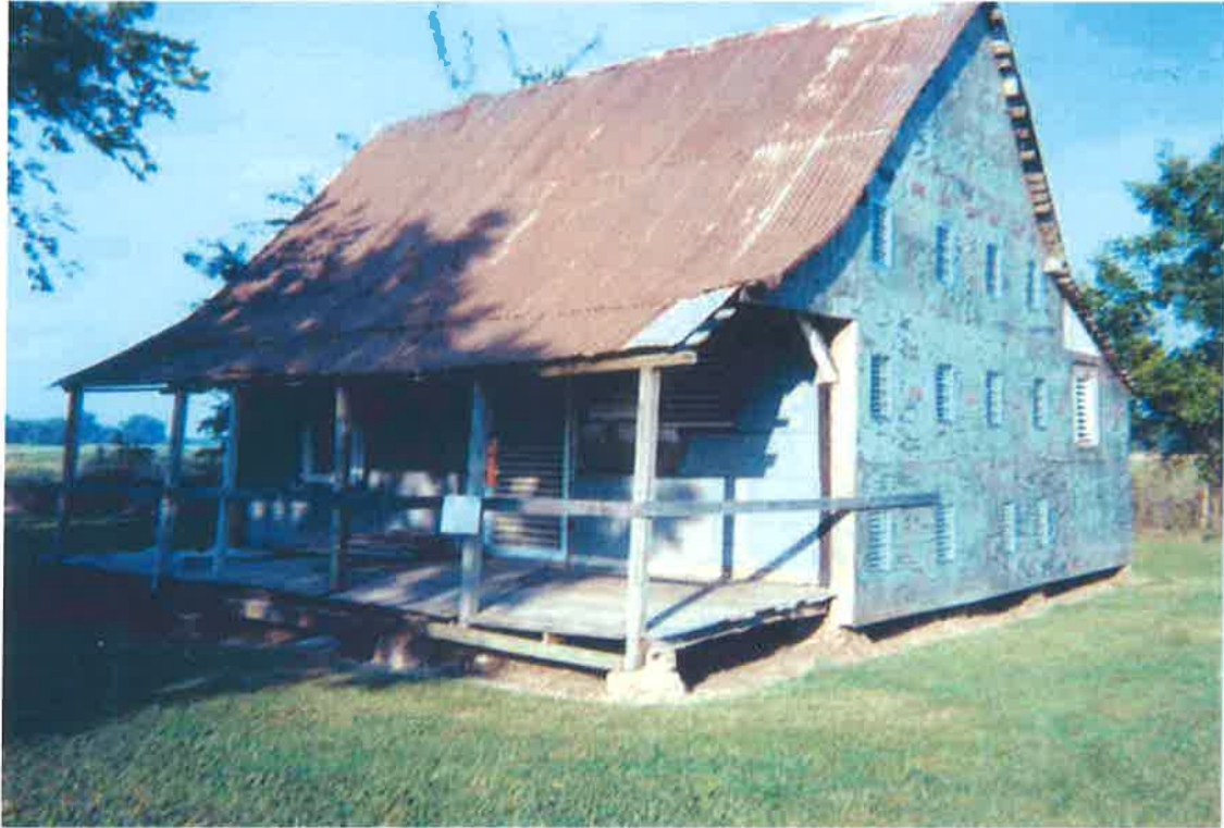
South Tenant Cabin, Cane River Creole National Historical Park, 2003
