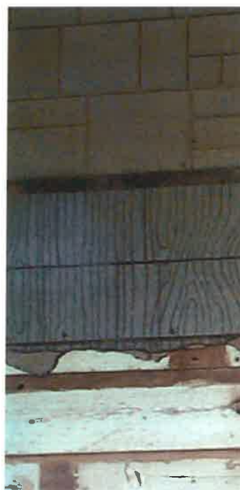
Detail of asphalt siding on the east elevation
