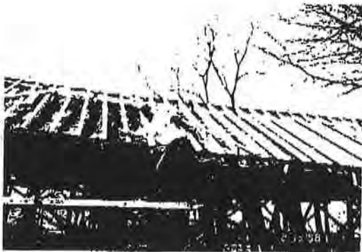
7-5. The Wagon Shed, south slope of roof during structural stabilization work.
