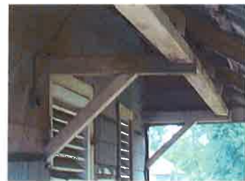
Detail of original east gallery roof framing
