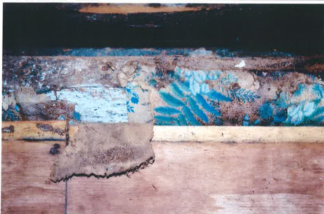
Image 88: Oakland Plantation. South Tenant Cabin, Room 104, 2002. Remnants of one of the wallpapers and earlier whitewashed framing under the plywood sheathing.
