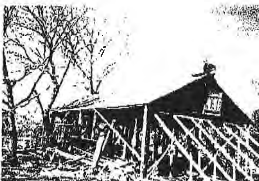
10-10. The Wagon Shed. Asphalt roof cover on south slope almost complete.
