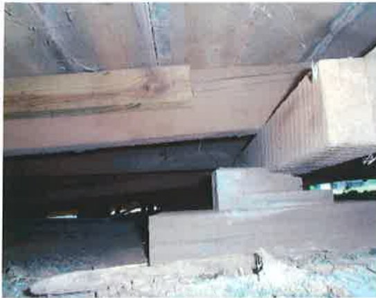
Wood shoring under building
