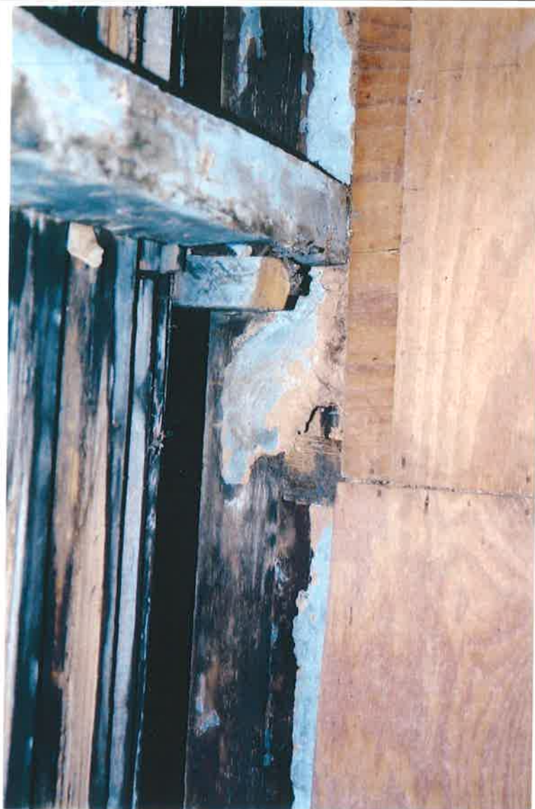
Image 68: Oakland Plantation. South Tenant Cabin, Room 104, east wall, 2002. The original bousillage walls can be seen behind the protective plywood sheathing.
