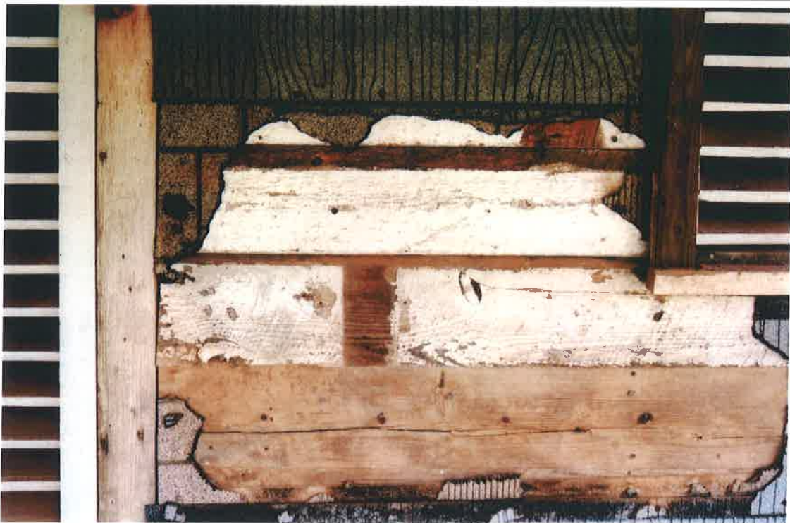
Image 86: Oakland Plantation. South Tenant Cabin, east elevation, 2002. Recycled board-and-batten sheathing under asphalt paper (and over bousillage ).
