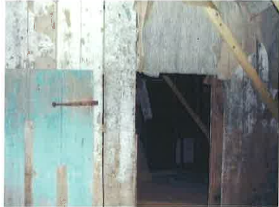
Detail of south wall of Room 102
