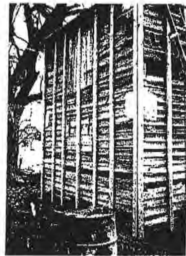
5-3. The East Pigeoneer during installation of the studs.
