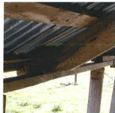
Detail of extended front gallery framing
