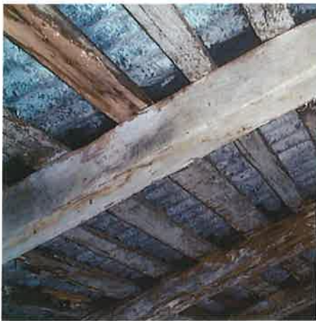
Rear gallery roof framing
