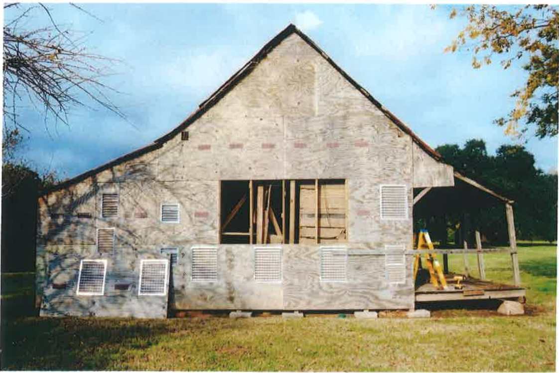
Image 67: Oakland Plantation. South Tenant Cabin, south elevation, 2002.
