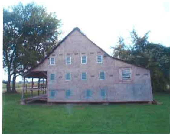
South Tenant Cabin, north elevation
