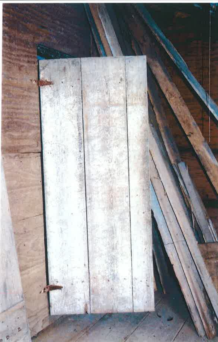
Image 80: Oakland Plantation. South Tenant Cabin, Room 104, 2002. Door D3.
