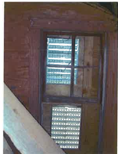
Interior of Window B
