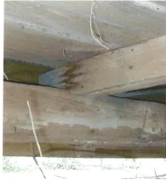
Rear gallery floor framing
