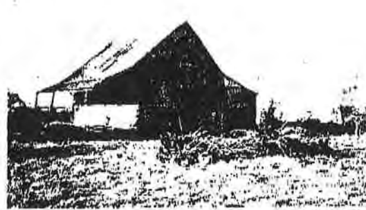
9-24. South Slave Quarter's, north elevation wall complete. Note poison ivy on ground.
