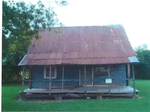
South Tenant Cabin, east elevation
