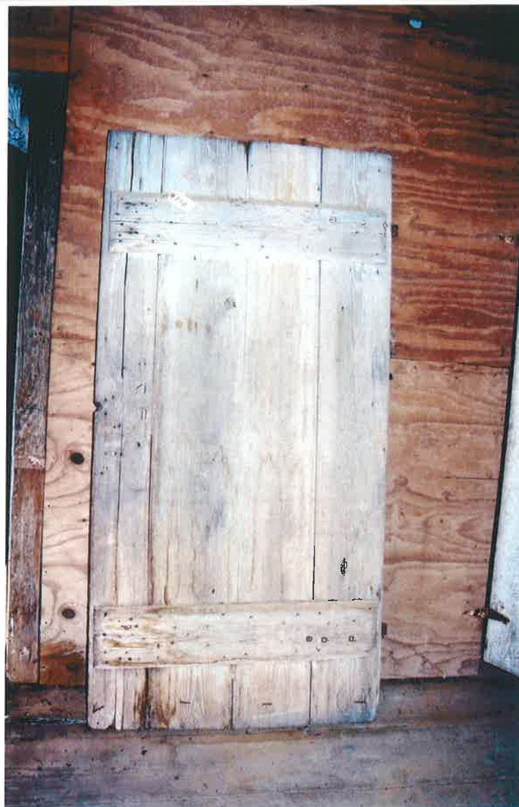
Image 81: Oakland Plantation. South Tenant Cabin, Room 104, 2002. Door D4.
