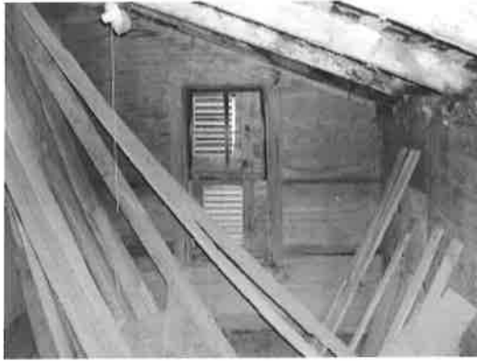
South wall in Room 104
