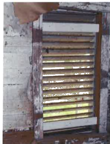
Exterior of Window E
