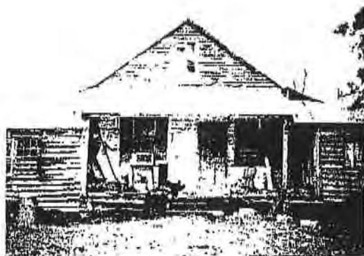
1-35. West elevation of the Store/Post Office prior to work. Note decayed porch deck.
