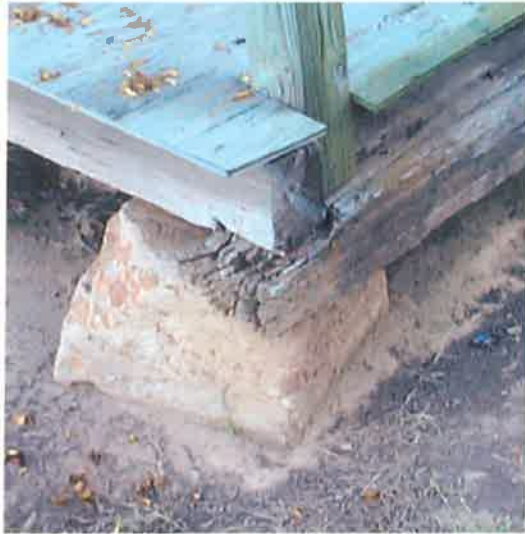
Foundation pier, front gallery
