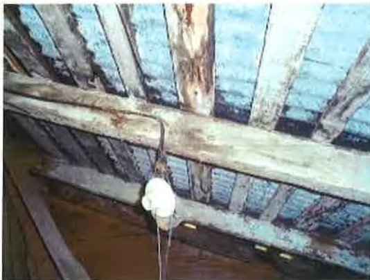
Detail of exposed roof and light fixture in Room 104
