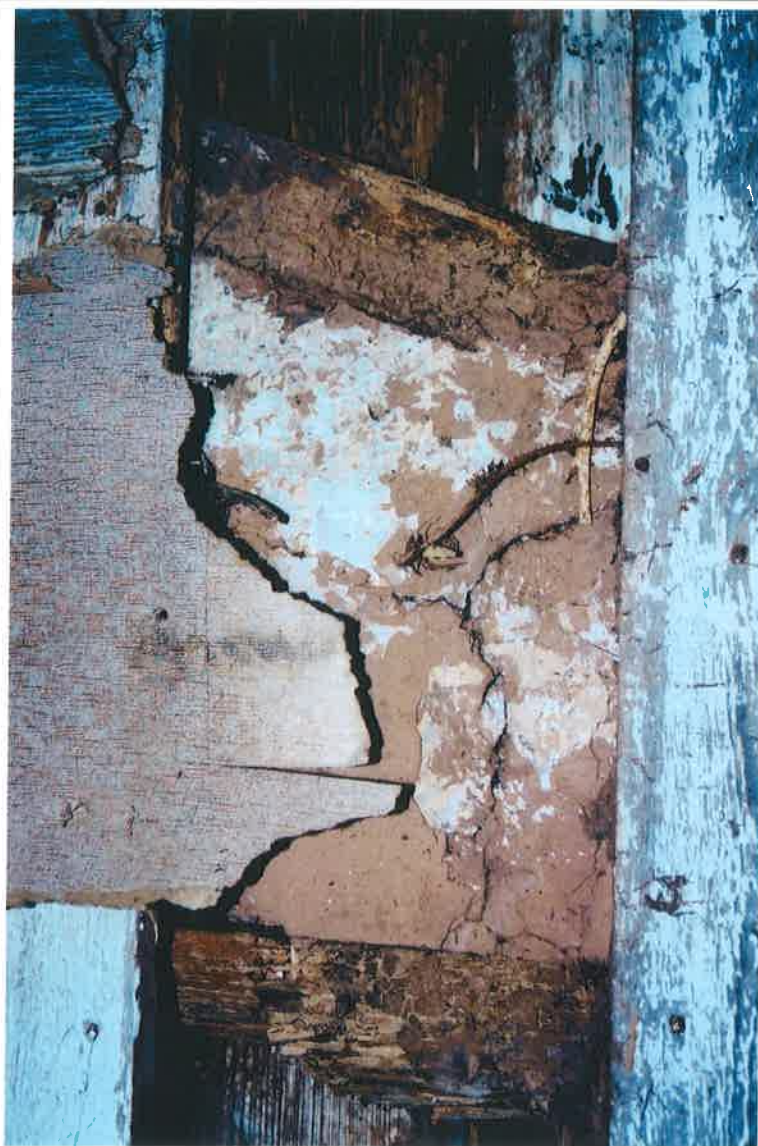
Image 72: Oakland Plantation. South Tenant Cabin, Room 102, north wall, 2002. The original whitewashed bousillage behind the sheathing and wallpaper.
