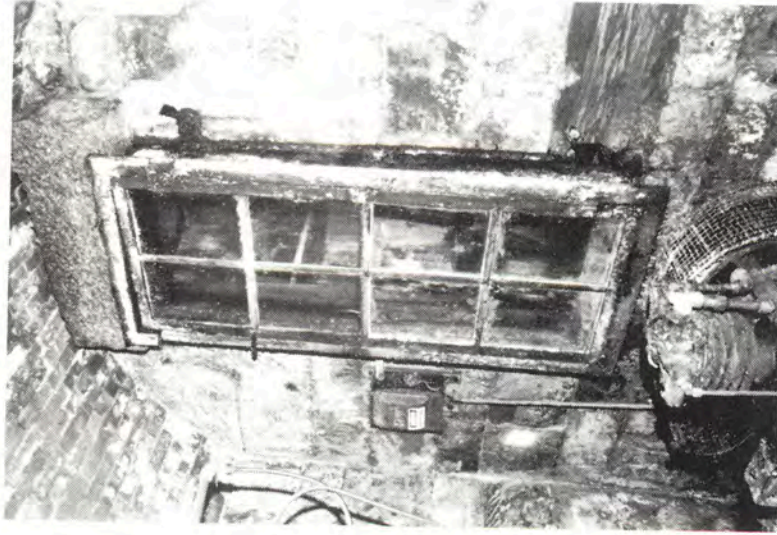
RIGHT: Photo 3-33 View of window in access corridor behind northwest magazine that lacks finish stonework. FAR RIGHT: Photo 3-34 View of window in a typical corridor behind magazine with finished stonework.
