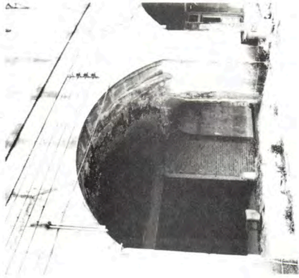
Photo 3-9 View looking southeast toward one of the bricked-in channel front casemates and vaulted brick and stone parade gallery.
