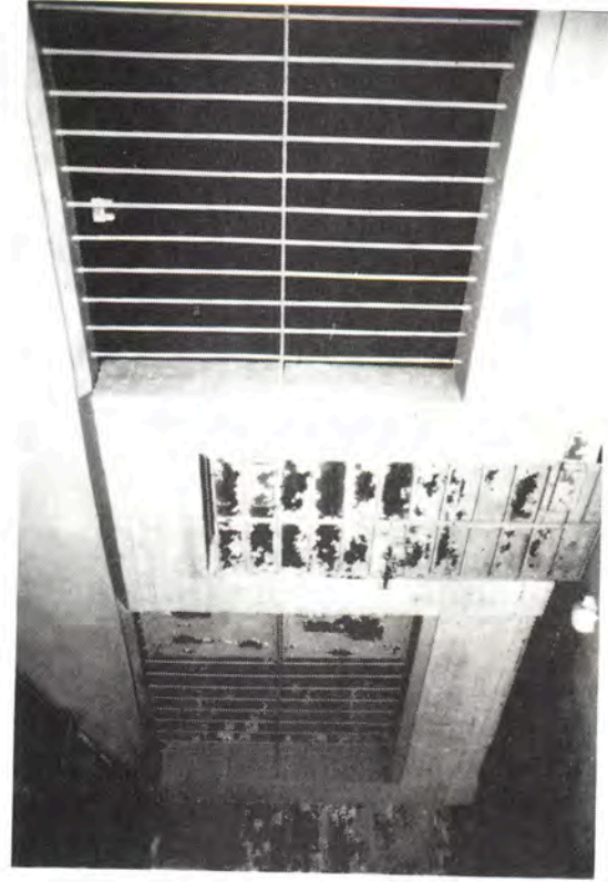
Photo 3-35 Typical holding cell on south side of second floor.
