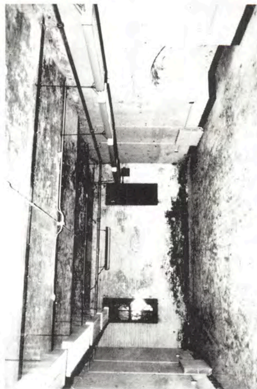
Photo 3-28 View looking north into typical north casemate; loop holes have windows and frames.
