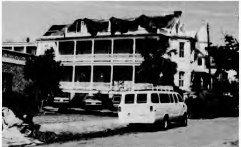
The immediate reaction to roof damage was to throw up plastic or canvas tarps to cover destroyed areas and to help prevent further interior damage.
