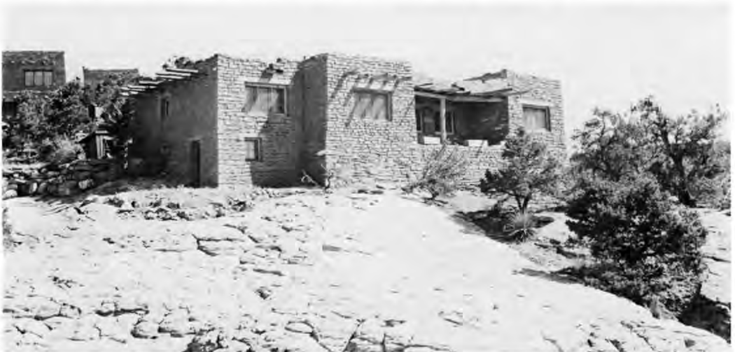
Headquarters building, Mesa Verde National Park, AZ, constructed between 1920 - 1930. Photo courtesy Mesa Verde NP. (Watch for more on Mesa Verde's early architecture in a future CRM.)
