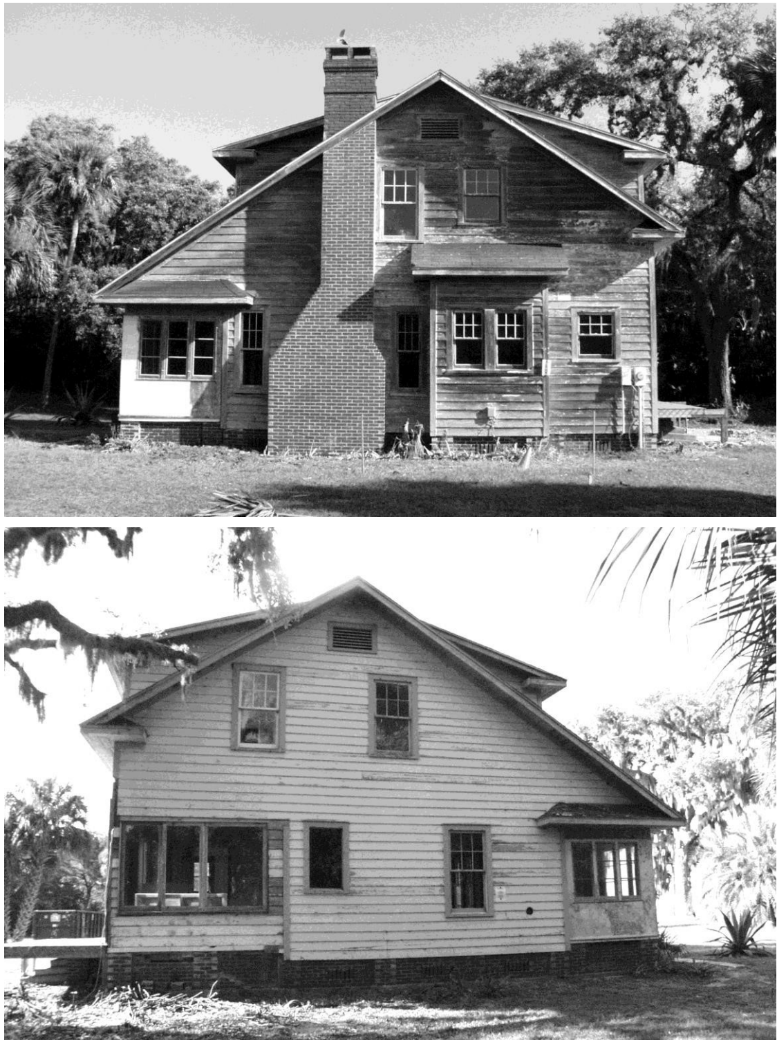
Figure 5 Top, view of south side of house; bottom, view of north side of house. (NPS-SERO-CRS, 2002)
