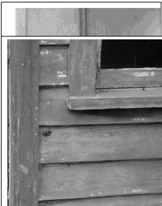
Figure 12 View of typical siding and trim. (NPS-SERO-CRS, 2002)
