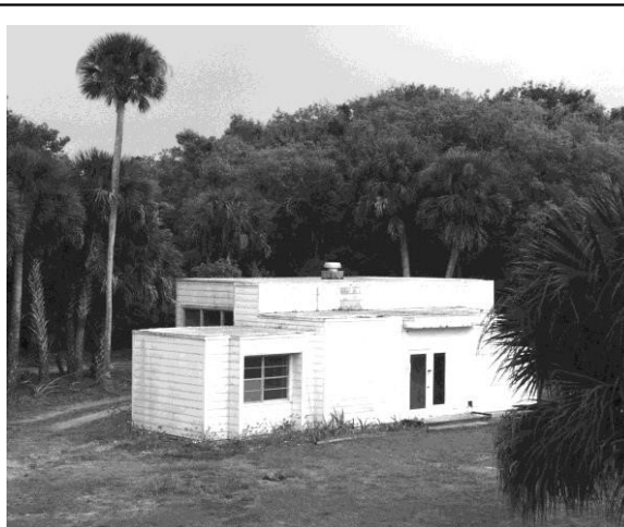
Figure 31 View to southeast of Guest House/Studio from second floor of main house. (NPS-SERO-CRS, 2002)
