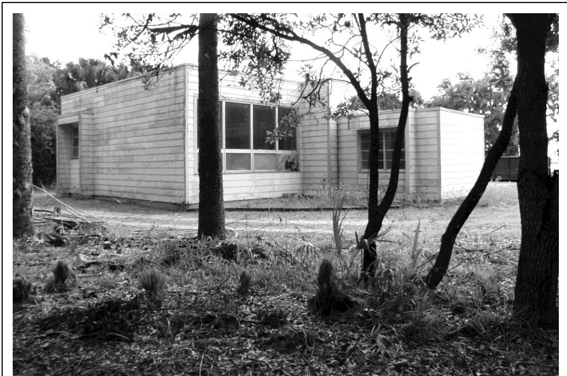
Figure 33 View to southwest of Guest House/Studio. (NPS-SERO-CRS, 2002)
