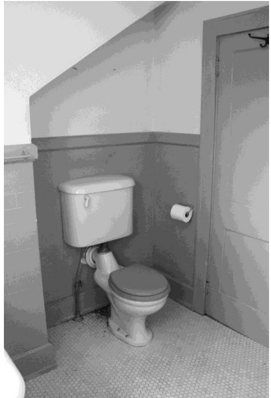
Figure 25 View to southwest in bathroom. (NPS-SERO-CRS, 2002)
