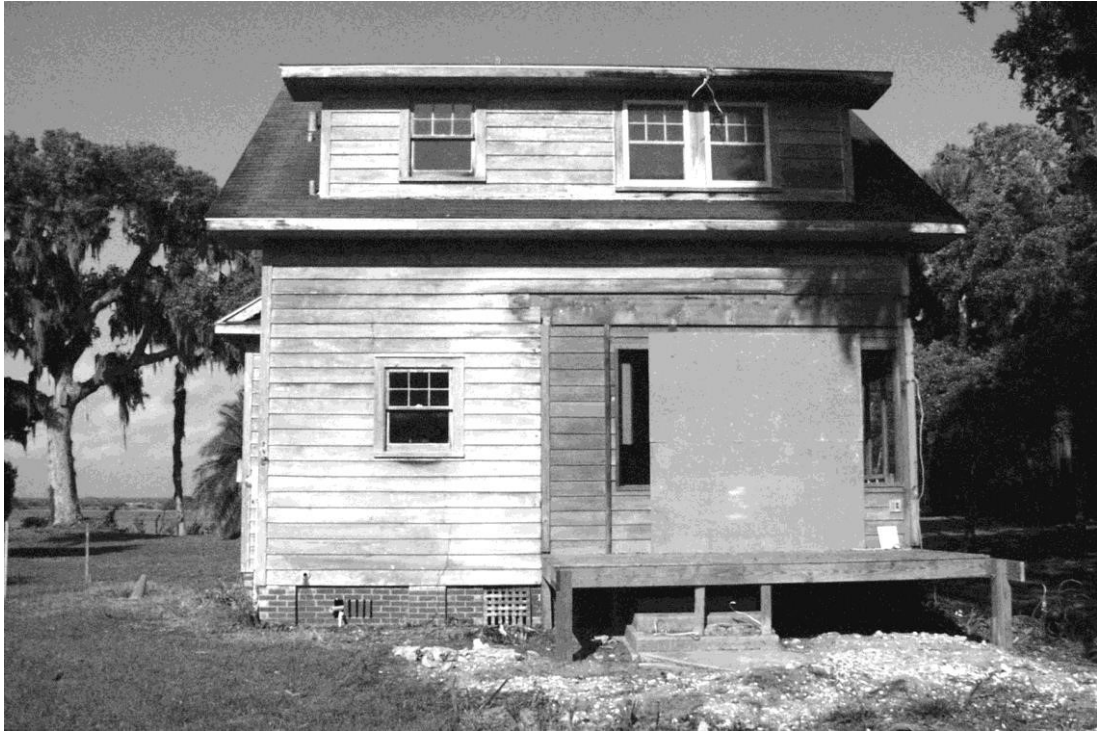
Figure 6 View of rear (east) side of house. The modern deck, which has been partially dismantled, was built over the original brick-and-concrete steps and stoop at the back door. (NPS-SERO-CRS, 2002)
