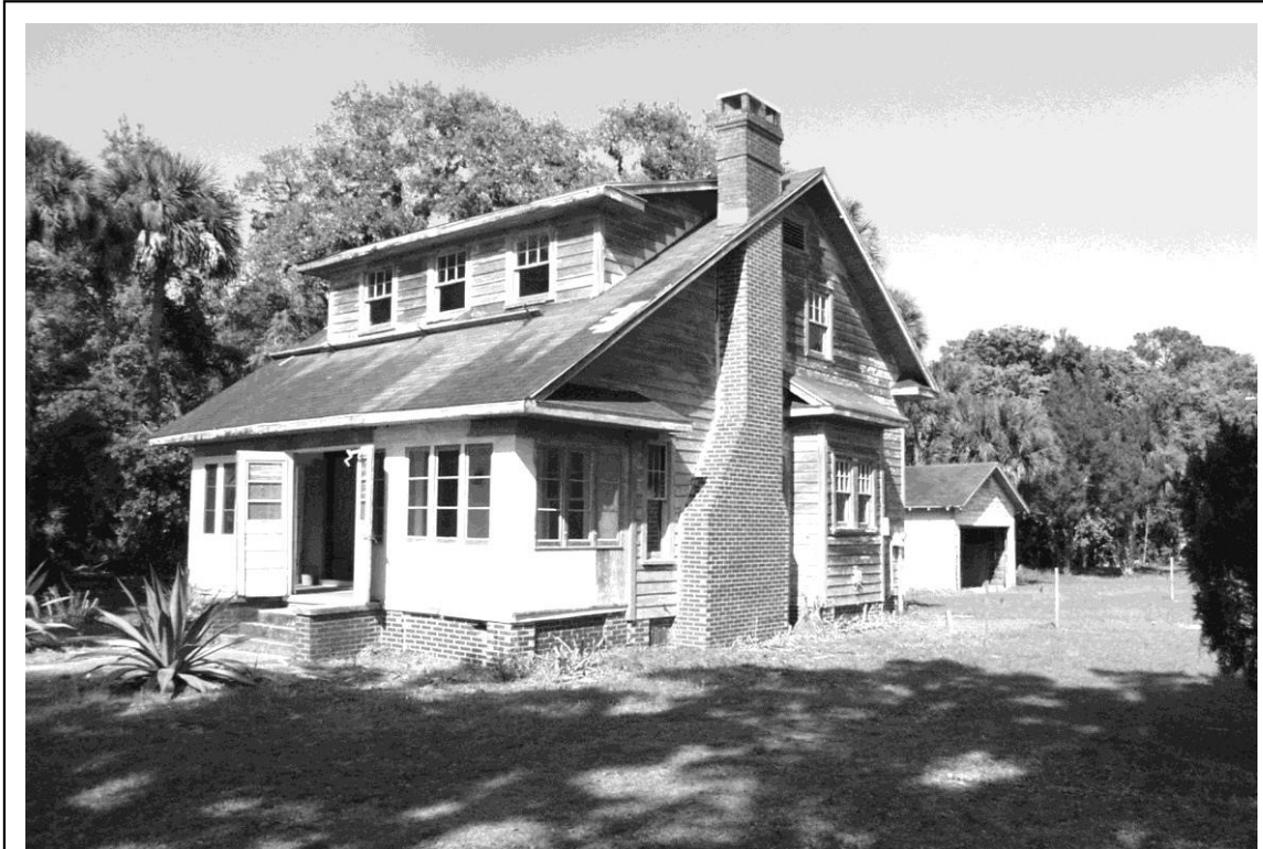
Figure 4 View to northeast of Leeper House. (NPS-SERO-CRS, 2002)
