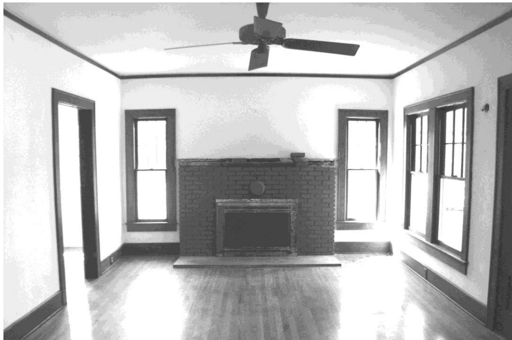
Figure 14 Top, view to north of living room (101). Bottom, view to south of living room. Except for missing sconces and mantle shelf, this room is in excellent condition. (NPS-SERO-CRS, 2002)
