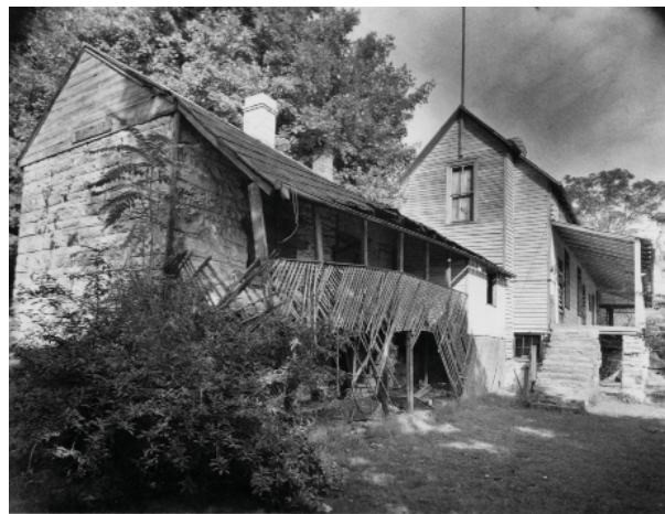
Figure 49. Photograph taken in 1956 showing the south end of the house and east elevation of the connector and dairy before the restoration. (CHCH Collection)
