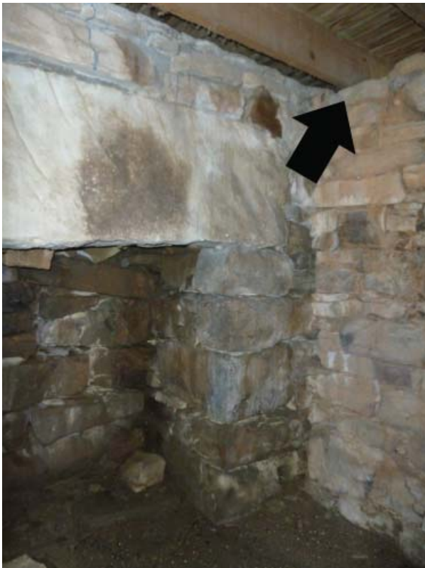
Figure 97. Northeast oblique of firebox in Room 006. Note porch joists extend across the east foundation wall.
