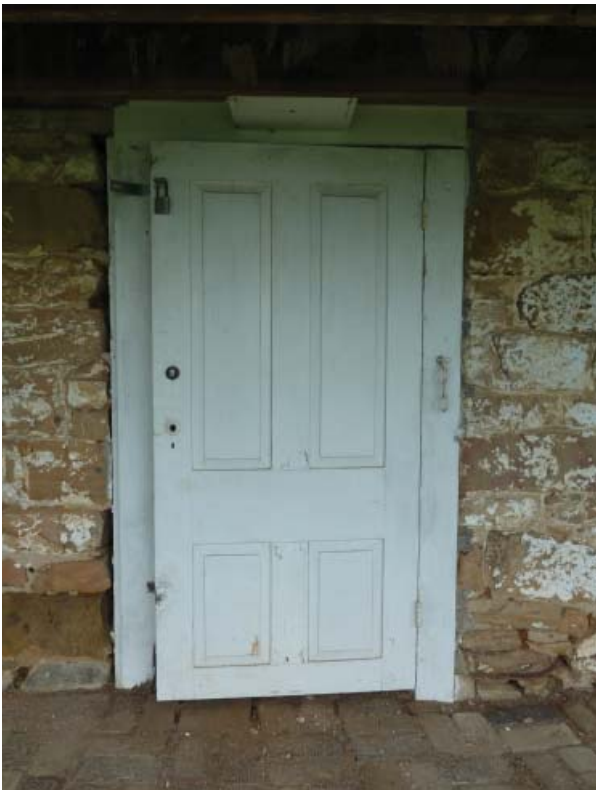
Figure 85. South doorway to the North Room (Room 001).
