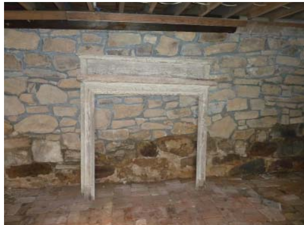
Figure 99. Stored fireplace mantel, North Room (Room 001).
