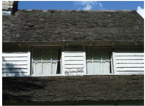
Figure 82. Typical second-floor sliding-sash window.
