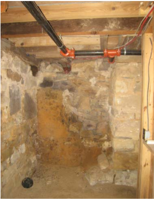
Figure 108. North wall of the Southwest Room (Room 003D). The west part (left) dates to 1866. The east part (right) dates to 1856.
