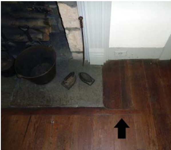
Figure 117. Modified hearth trim board, perhaps reused from the 1856 house, indicates a wider hearth.
