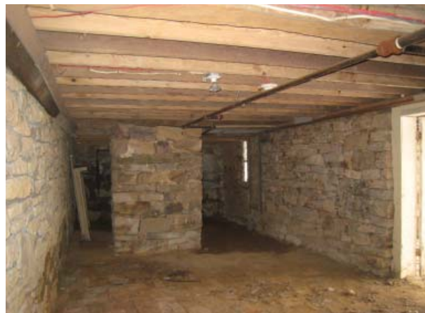
Figure 95. Northeast oblique view of the North Room (Room 001).
