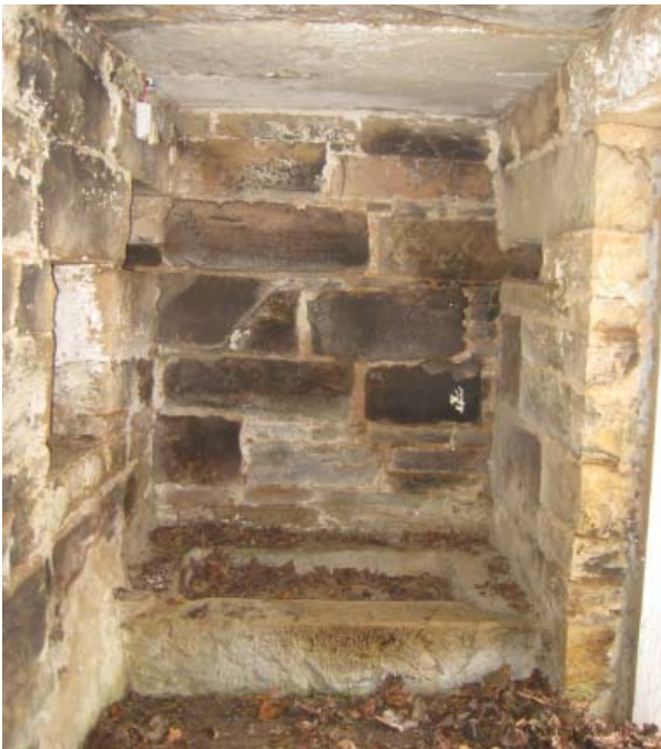
Figure 150. Stone basin along the north wall of the Dairy at basement level.
