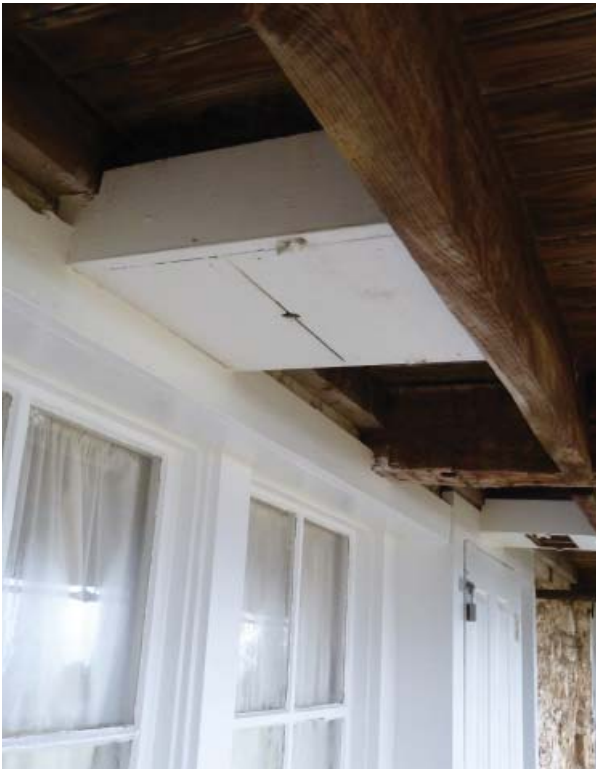
Figure 75. Light box above basement-level doorways.
