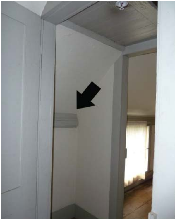
Figure 135. Window track continues from the Central Bedroom (Room 203) behind plaster walls through the passageway into the South Bedroom (Room 204).
