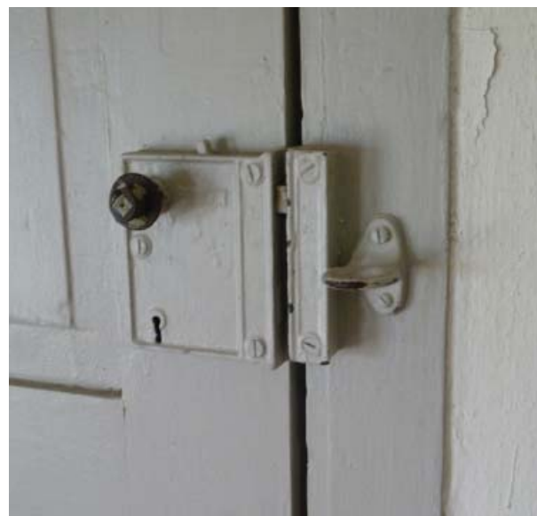
Figure 131. Rim lock and ring on south door of Central Bedroom (Room 203).
