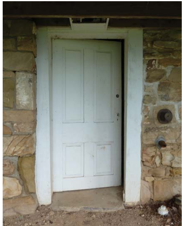
Figure 87. Entrance to the Utility Room (Room 003C).
