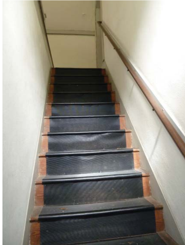
Figure 114. Staircase in Room 102.
