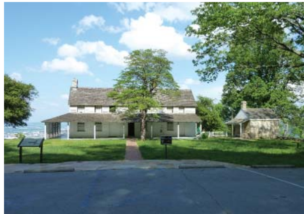
Figure 60. West elevation of the House.
