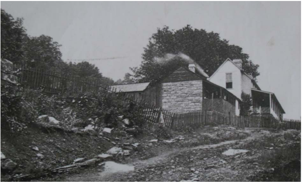
Figure 26. Photograph dated 1897. Note smoke emitting from the north chimney of the connector. (CHCH Collection)
