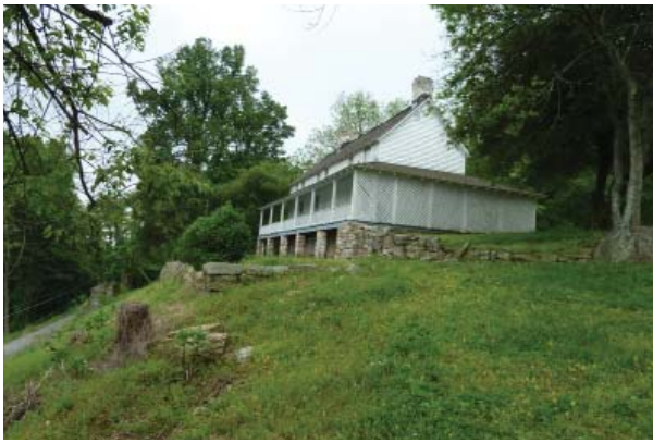
Figure 58. East side of house with drop-off to Cravens Terrace Road below.
