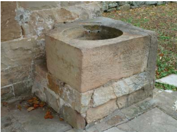
Figure 149. Water basin on front porch of the Dairy.
