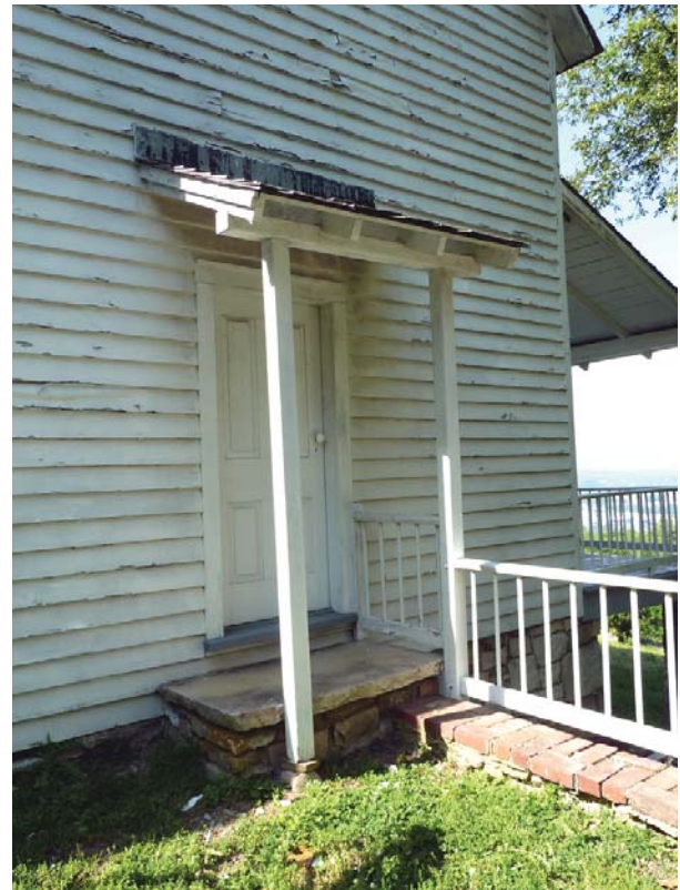
Figure 91. Side Entrance Porch on south elevation.
