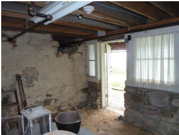
Figure 101. Northeast oblique of the Middle Room (Room 002).
