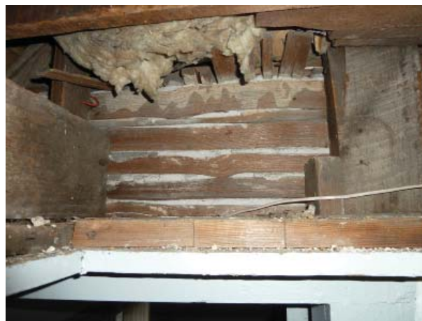
Figure 68. Riven lath and salvaged lumber for framing as seen at the ceiling hatch of the South Bedroom (Room 204).
