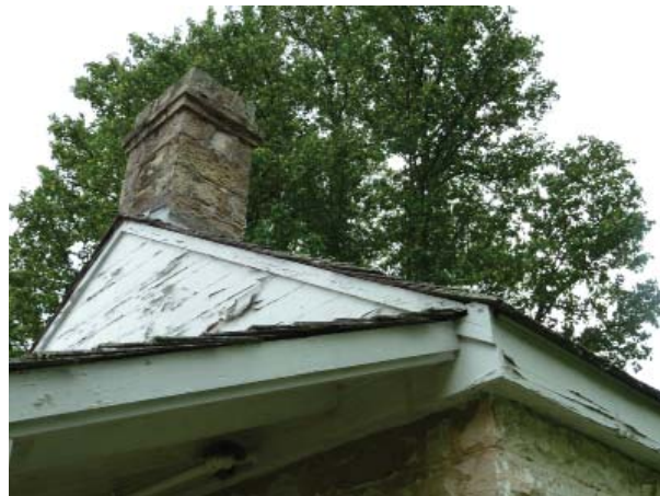
Figure 141. Dairy gable, cornice, and porch roof.
