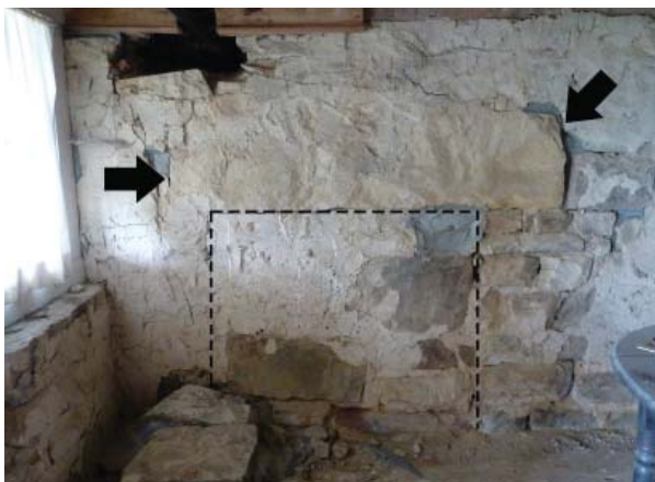
Figure 102. Filled-in fireplace on south wall of the Middle Room (Room 002), originally the south exterior wall of the 1856 House. Note the large stone lintel.
