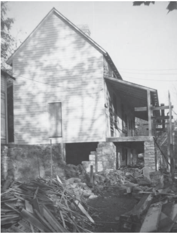
Figure 50. Photograph of south elevation taken while the project was underway. Demolition debris is stacked in the lower yard. (CHCH Collection)
