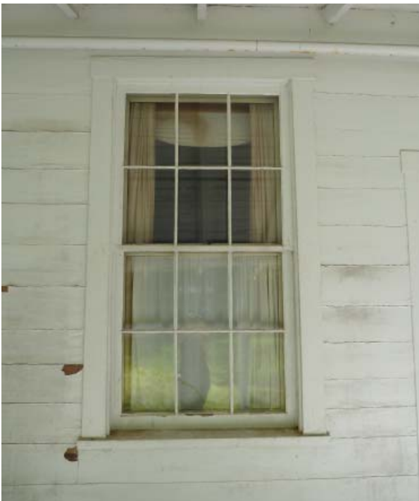
Figure 81. Typical first-floor double-hung window.
