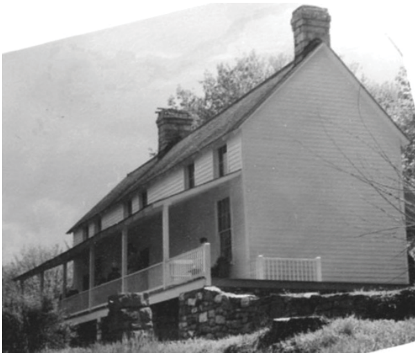
Figure 42. Photograph of north elevation taken 4/21/1957 during the open house celebrating the restoration. The north porch has been replaced by an open deck with railing protecting a stair opening, and the flush siding has been replaced by weatherboards. (Burton Jones, photographer; CPL Photograph Collection)
