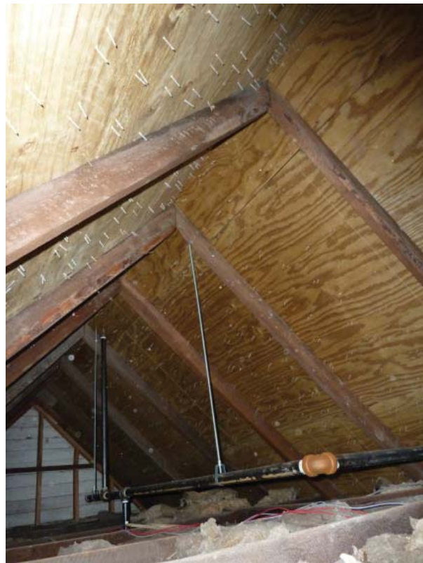
Figure 73. Roof rafters (1866) and modern plywood decking.
