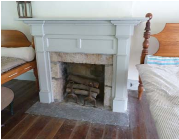
Figure 125. Fireplace and early mantel on the north wall of the North Bedroom (Room 201).
