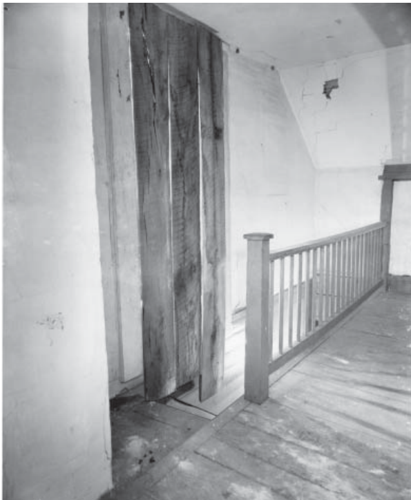
Figure 44. Photograph taken in 1956 looking southwest towards the stair of the south stair tower as it reached the second-floor south room. The two-over-two south window is boarded over. (CHCH Collection)
