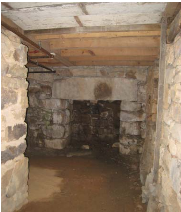
Figure 98. Fireplace on north exterior wall of the 1856 House, now North Room (Room 001).
