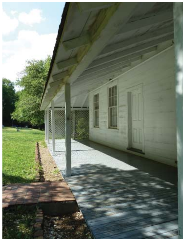
Figure 89. Porch on west elevation.
