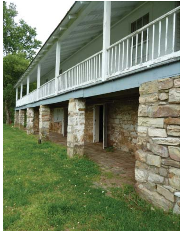
Figure 65. East porch foundation piers.
