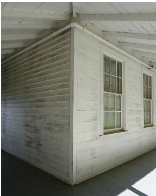
Figure 67. Northwest oblique with 1956-57 weatherboard on north wall and 1866 flush siding on west wall.
