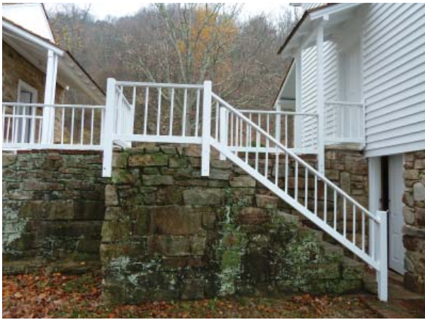
Figure 93. East elevation of stairs from basement to yard between the House and Dairy.
