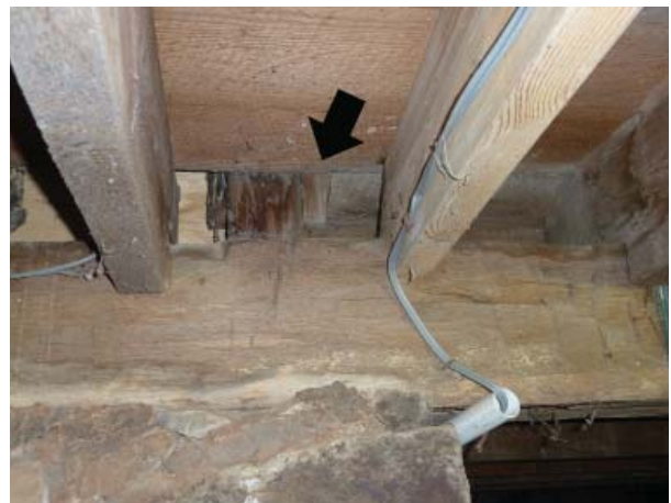
Figure 71. 1866 2" by 4" wall stud (arrow) and notched 1866 and 1956-57 floor joists at west wall sill, Room 003D.
