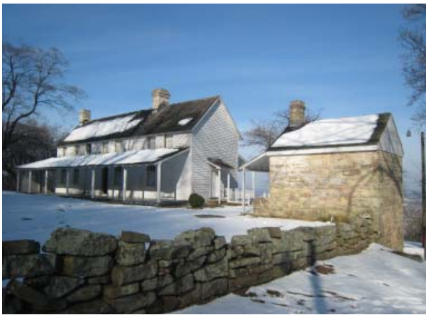
Figure 138. Southwest oblique of the House and Dairy.
