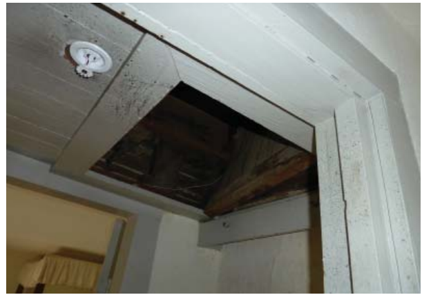
Figure 136. Attic hatch in the passageway of the South Bedroom (Room 204).
