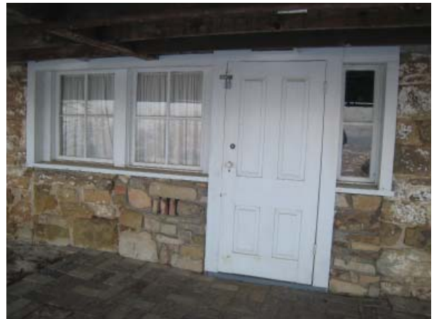
Figure 86. Windows and door at Room 002.
