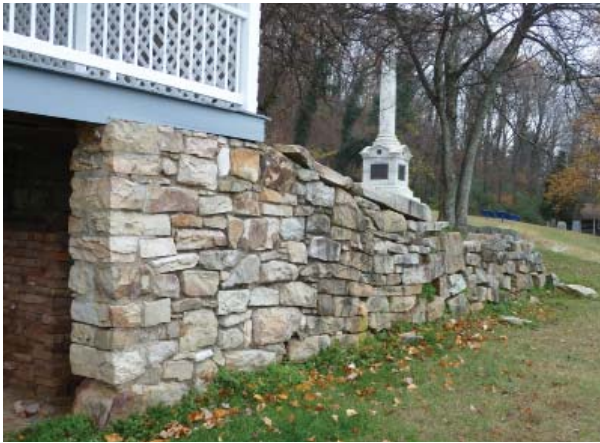
Figure 66. Extension of stone foundation wall north of the House.
