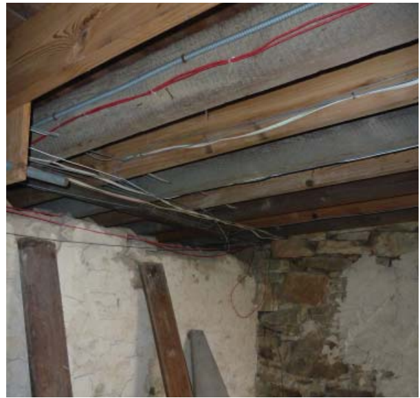
Figure 70. Alternating 1866 floor joists and 1956-57 joists.
