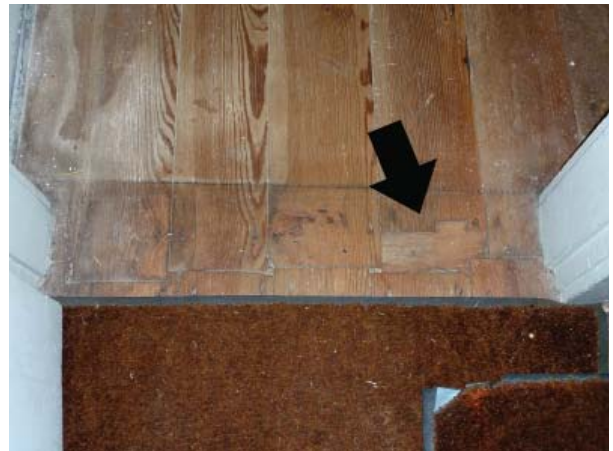
Figure 113. Seam in flooring at the south doorway. Note the patch possibly for a wall stud.
