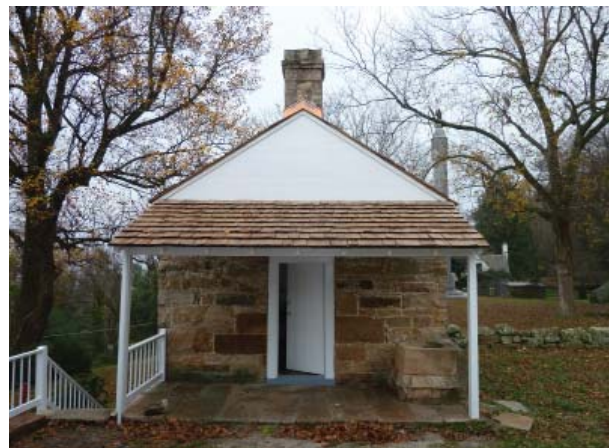
Figure 137. Front (north) elevation of the Dairy.
