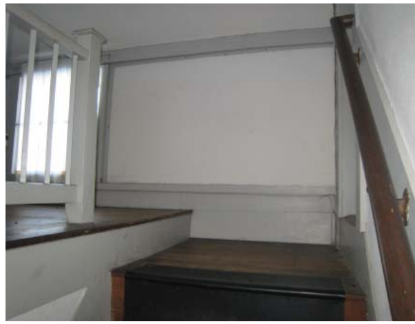
Figure 126. Top landing in Upper Stair Hall (Room 202) looking east.
