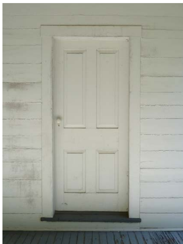
Figure 84. Typical four-panel exterior door.
