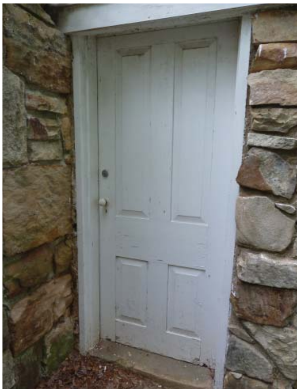
Figure 88. Entrance to the Hall (Room 003C).
