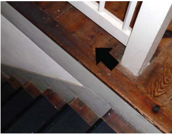
Figure 123. Floor patch for door frame of early board wall.
