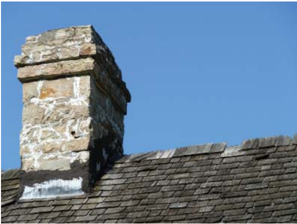
Figure 80. Central stone chimney.
