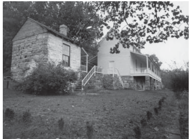
Figure 51. Photograph from the southeast taken in 1957 after the restoration, showing removal of the connector, its porch, and the stone staircase to the house porch. Visible are the two replacement staircases ascending to the upper terrace. (CPL Photograph Collection)
