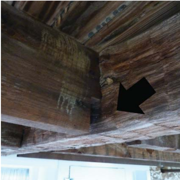
Figure 72. Lap joint of hatcheted girder and joist typical at the east porch.
