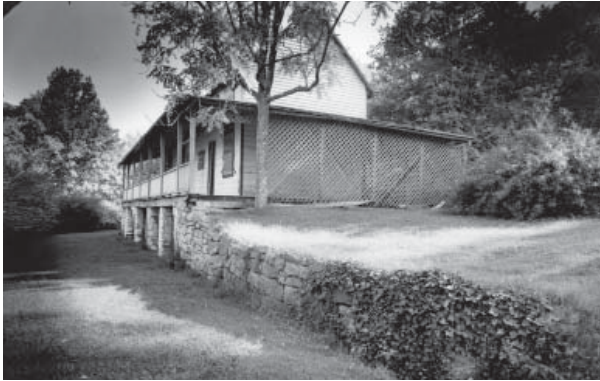
Figure 41. Photograph of north elevation taken in 1956 before the restoration. Flush siding can be seen beneath the latticed north porch. (CHCH Collection)
