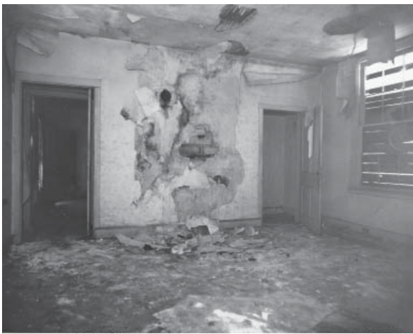
Figure 47. Photograph of "dining room" taken in 1956 before the restoration, showing evidence of the former firebox and mantelpiece. (CHCH Acc 212, Folder 28A)
