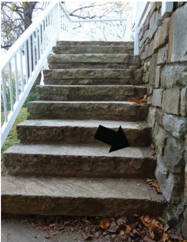
Figure 94. Reused original steps with 6" infill stones on the interior (west) side.
