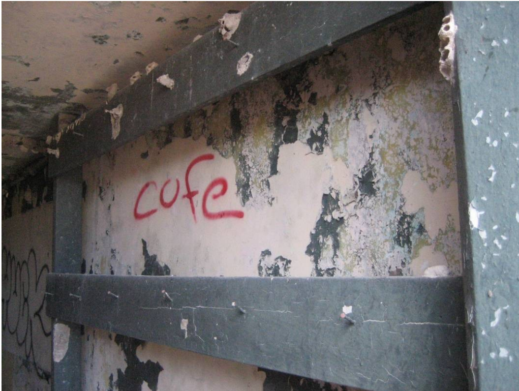
Fire-control Bunker C: Intact green paint on wood rack inside bunker.
