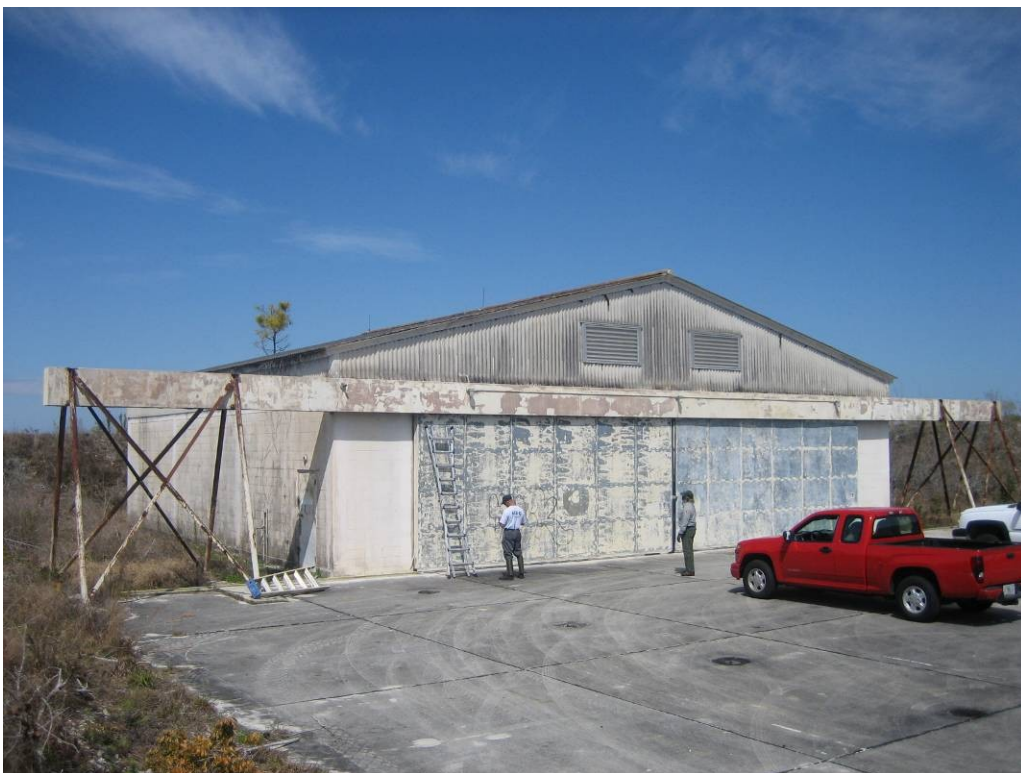
Missile Barn C: Intact beige paint on exterior barn door.
