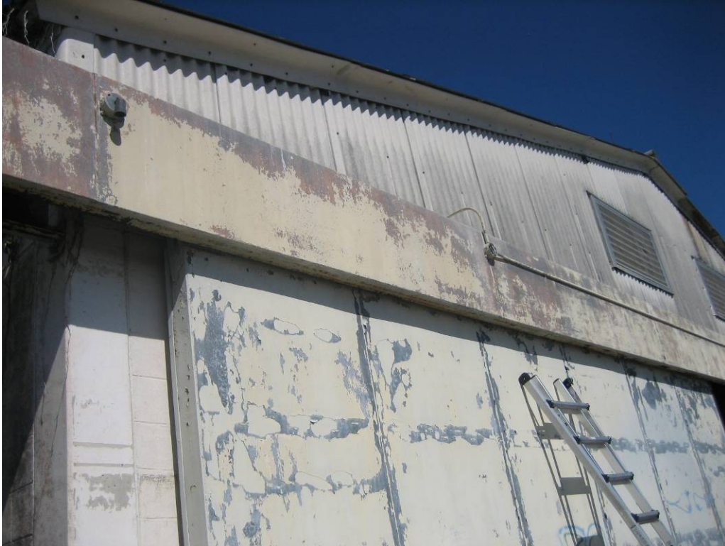
Missile Barn A: Intact pink paint on metal rail beam on barn door.
