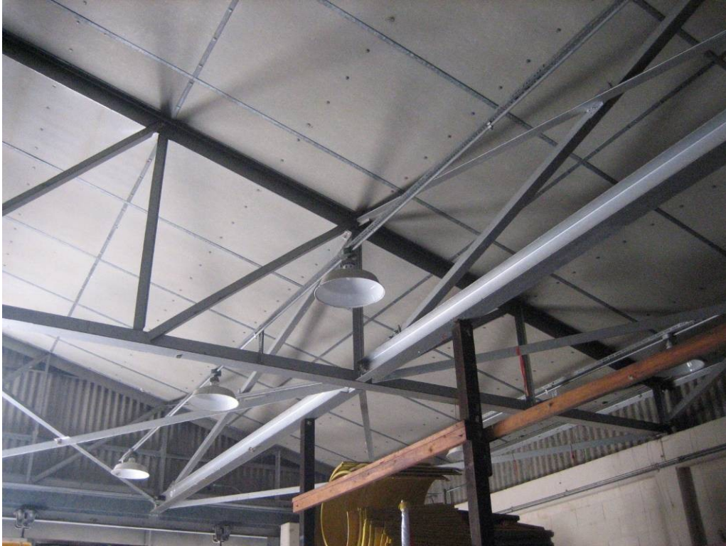
Missile Barn A: Intact gray paint on interior metal beams.
