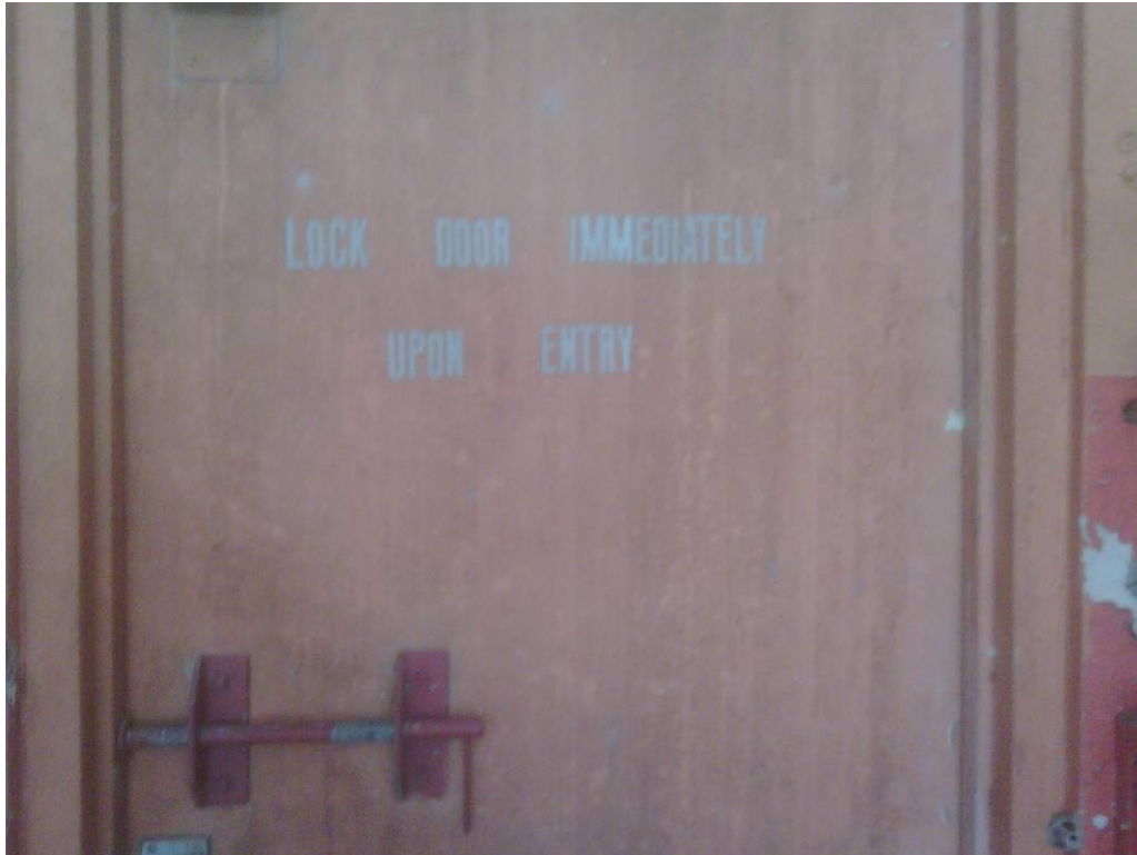
Missile Barn C: Intact orange paint on interior metal exit door.
