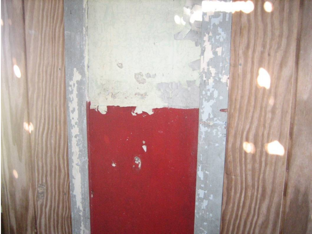
Sign/Generator Building 190A: Intact red paint on concrete block wall.
