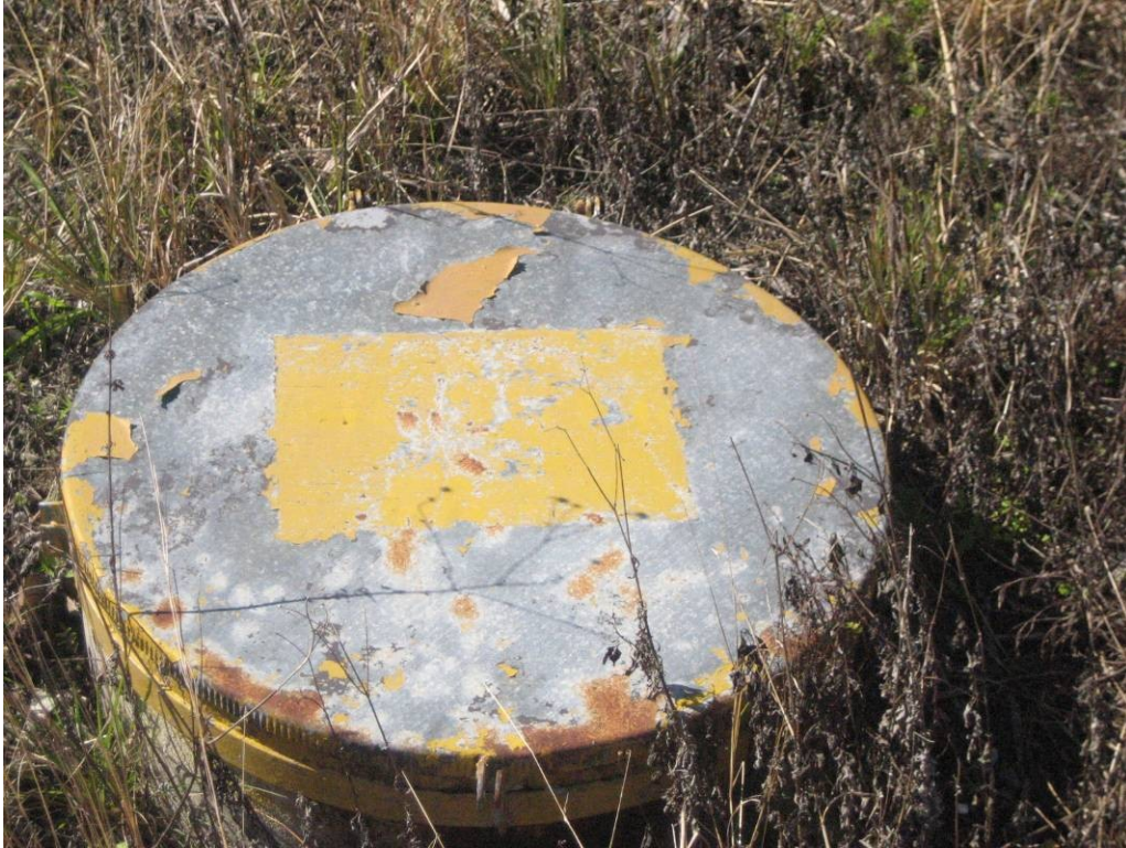
Missile Barn B: Intact yellow paint on manhole cover near bunker.
