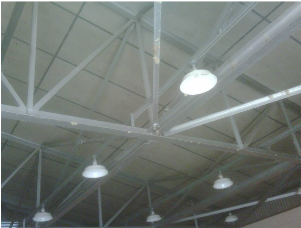
Missile Barn C: Intact gray paint on interior metal support beams.
