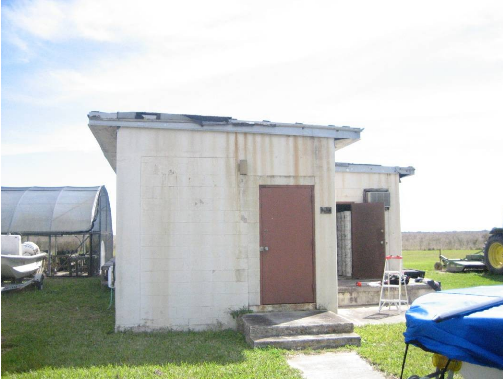
190B Building: Intact beige paint on exterior concrete block walls.
