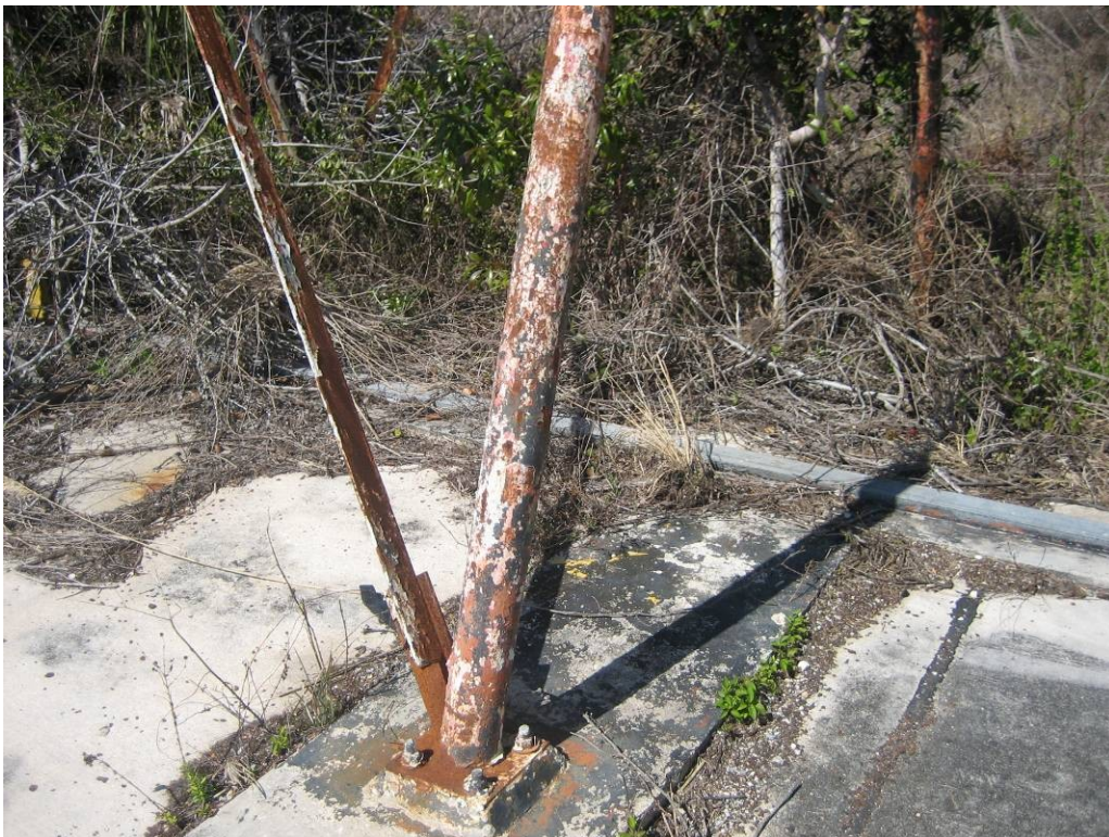
Missile Barn A: Intact pink paint on supports for rail beam on barn door.
