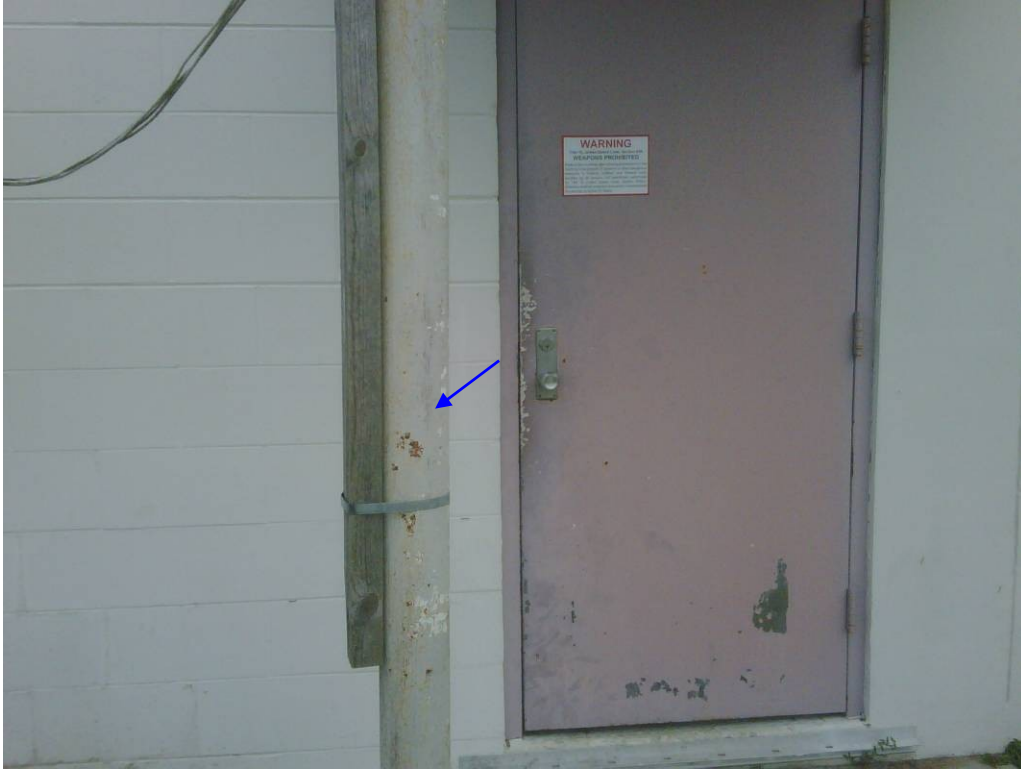
Administration Building: Beige paint on exterior metal column.
