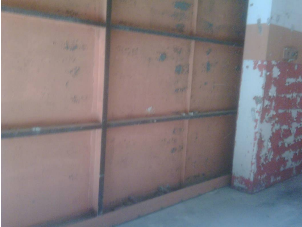
Missile Barn C: Intact orange and black paint on interior of barn door.
