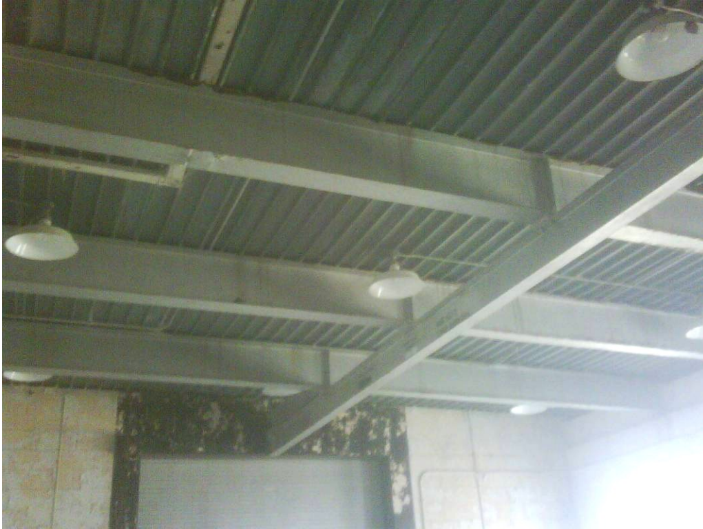
Missile Assembly Building: Intact gray paint on metal support beams.
