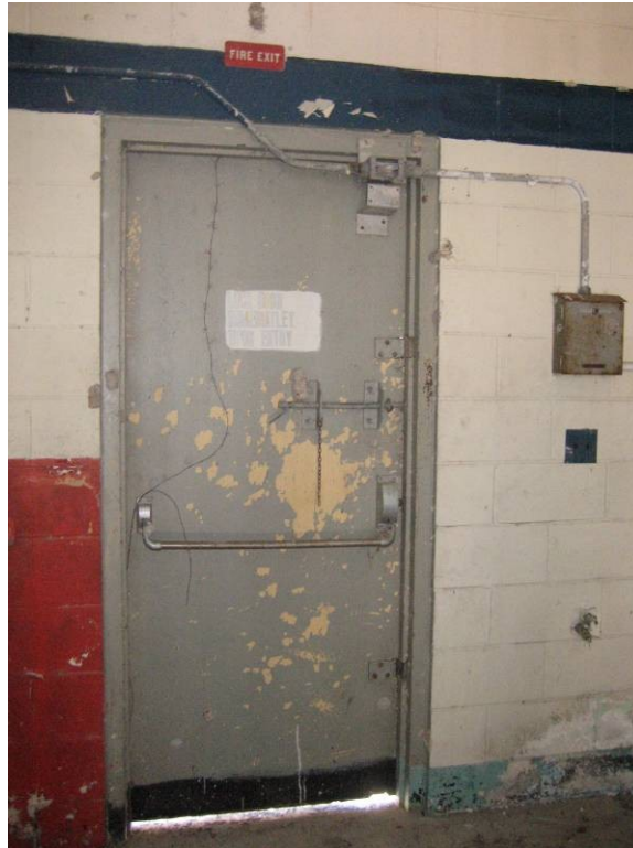
Missile Barn A: Chalking gray paint on interior metal exit door.
