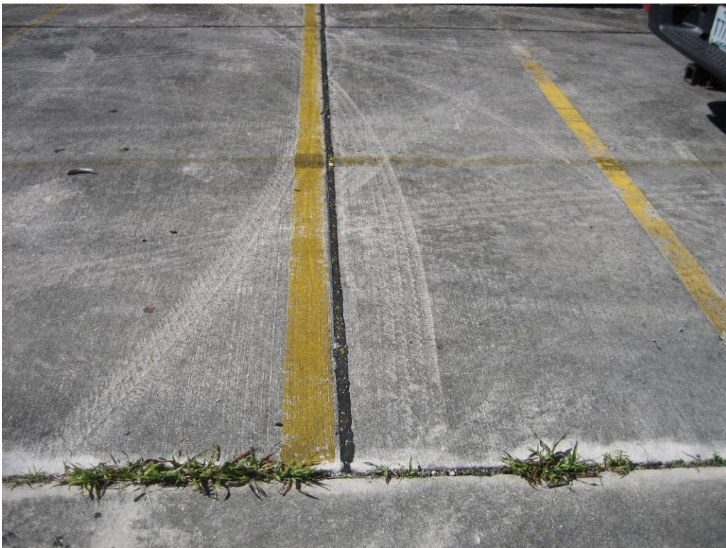
Missile Barn A: Intact yellow paint on exterior concrete slab.
