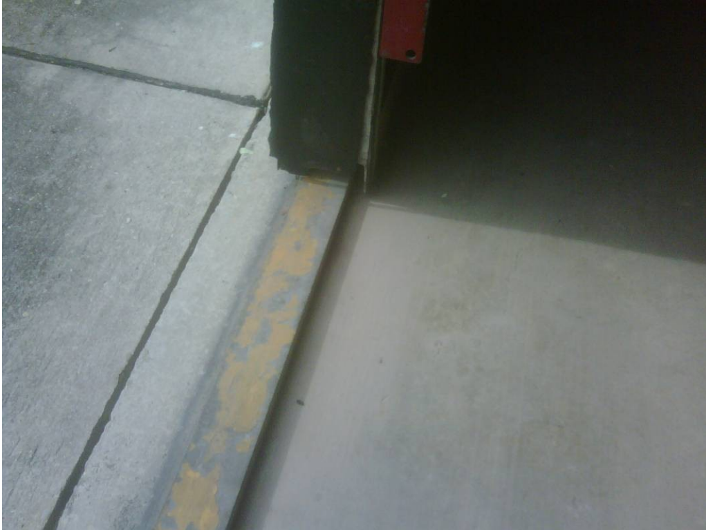
Missile Barn C: Intact yellow paint on base rail of barn door.
