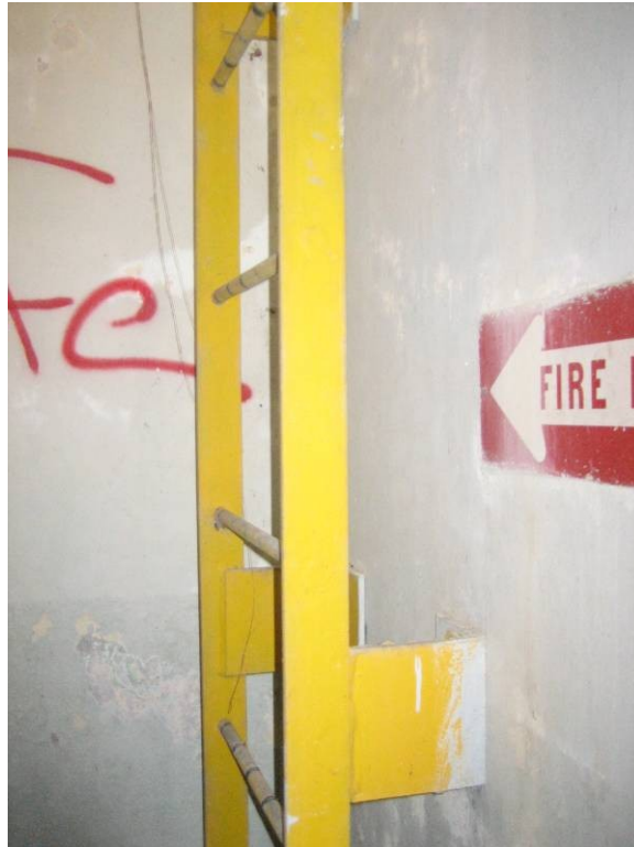
Fire-control Bunker C: Intact yellow paint on ladder in escape hatch.
