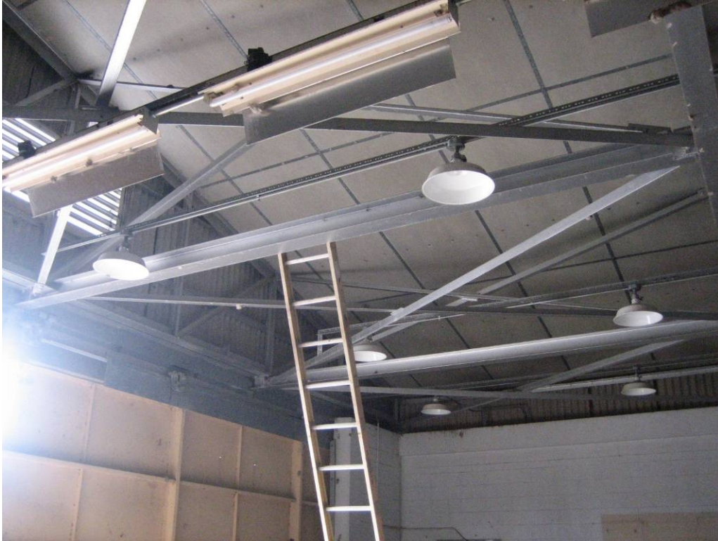
Missile Barn B: Intact gray paint on interior support beams.
