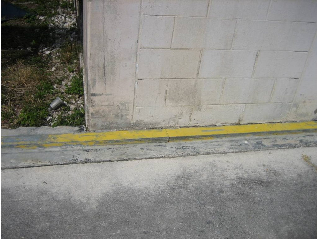
Missile Barn C: Intact yellow paint on exterior base rail for barn door.
