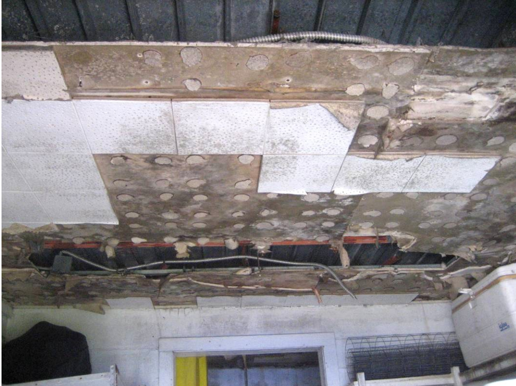
190 B Building: West side nonACM drywall, plaster, ceiling tile glue, and ceiling tile.
