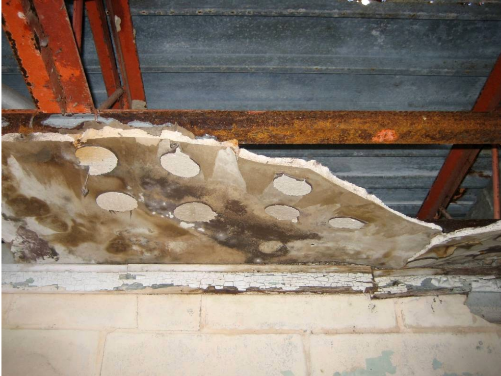
190A Building: NonACM drywall, ceiling tile glue, and ceiling tile.
