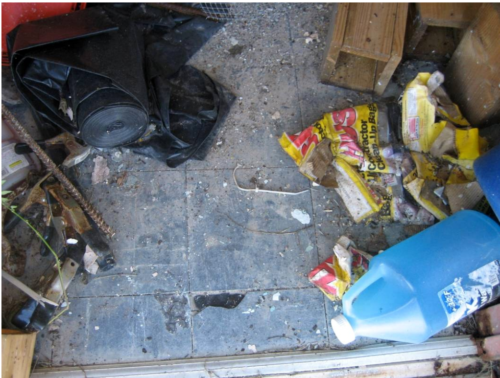
190A Building : ACM 9" black vinyl floor tile and mastic.
