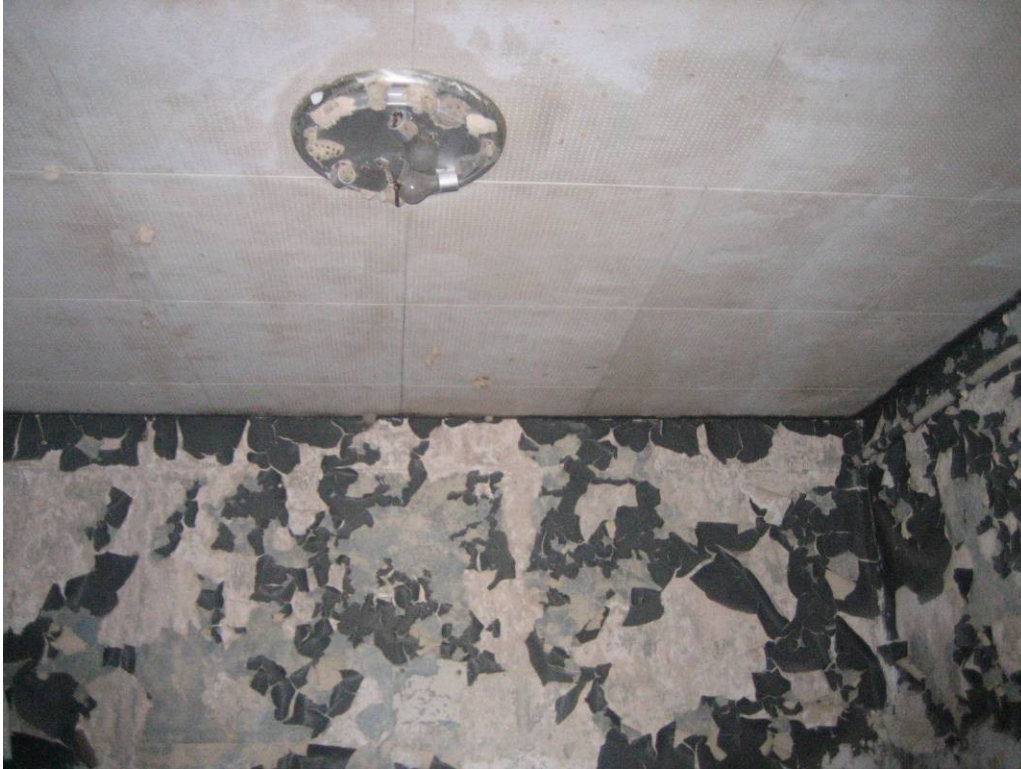
Fire-control Bunker A: ACM interior cementitious ceiling tiles.
