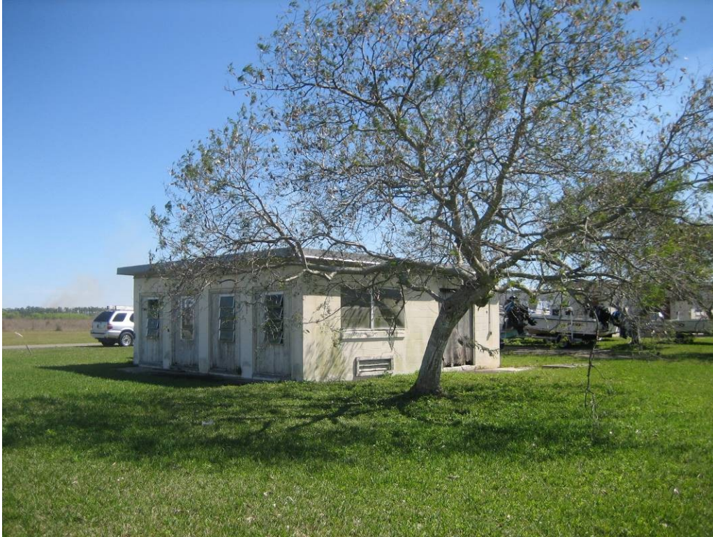
Sign/Generator Building 190A in Admin/Control Area.
