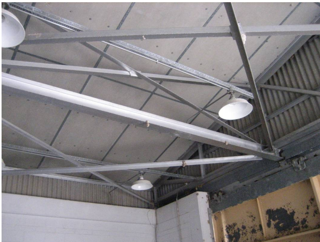
Missile Barn B: ACM interior cementitious ceiling panels.
