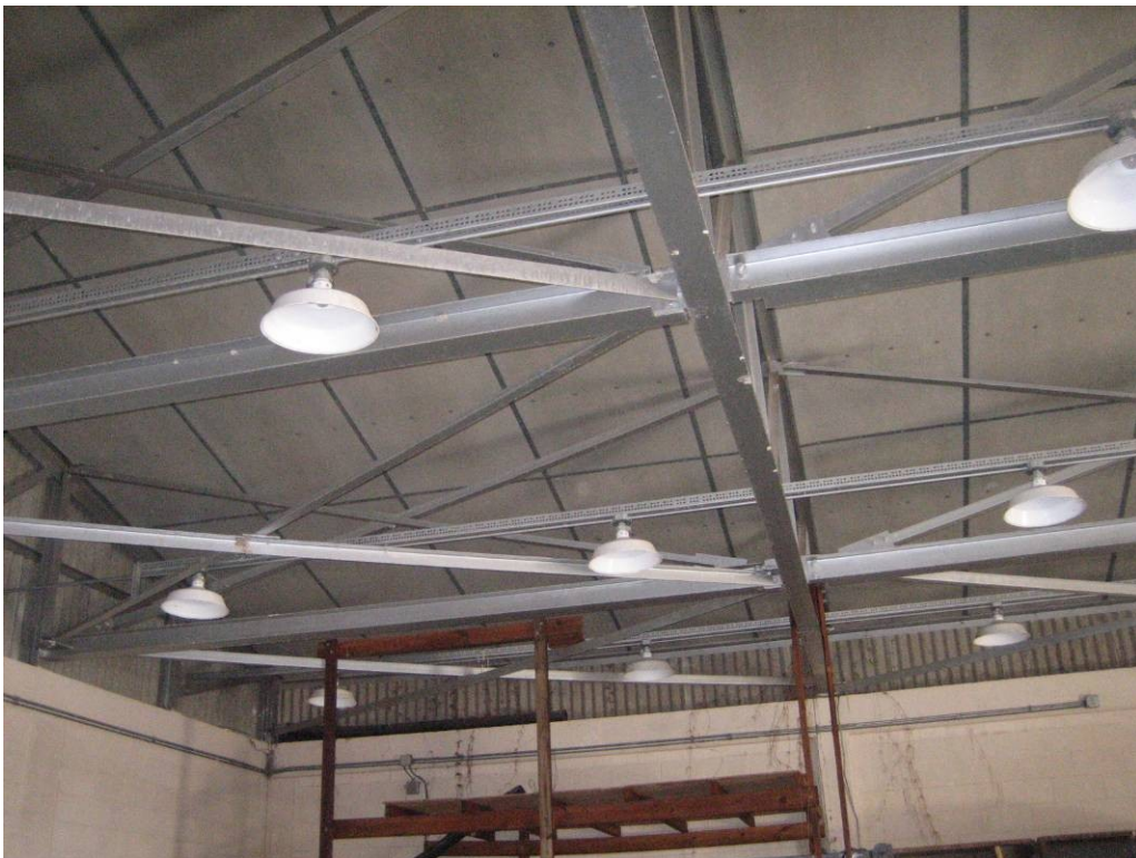
Missile Barn A: ACM interior cementitious ceiling panels.
