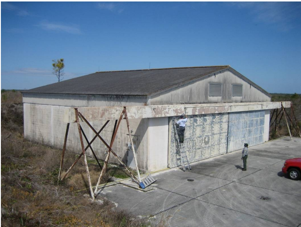
Missile Barn C: ACM exterior cementitious siding and roofing panels.
