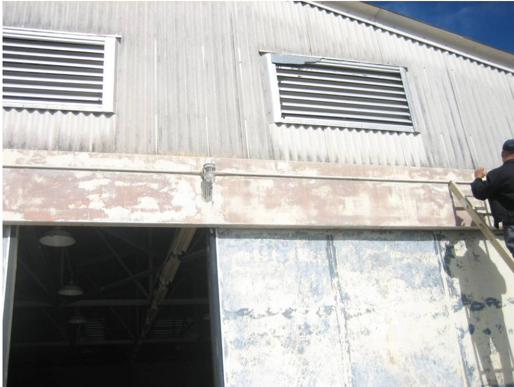
Missile Barn B: ACM exterior cementitious siding panels.
