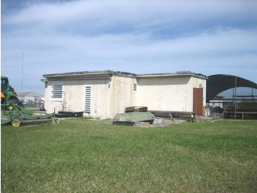
190 B Building in Admin/Control Area.
