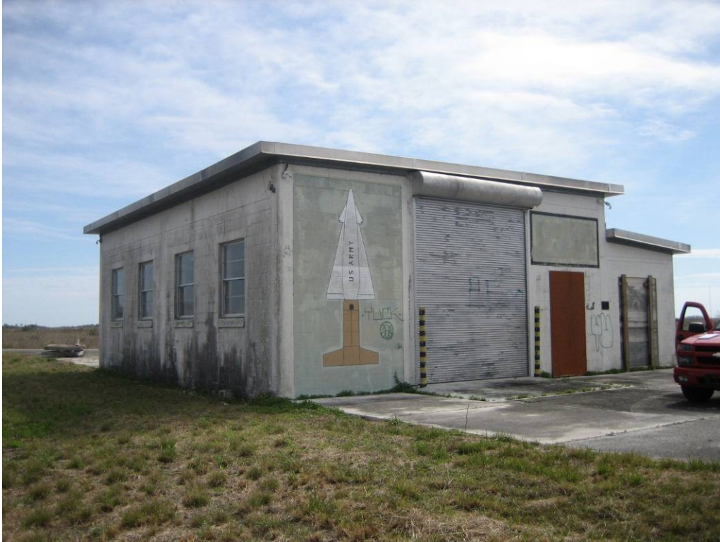
Missile Assembly Building exterior view.
