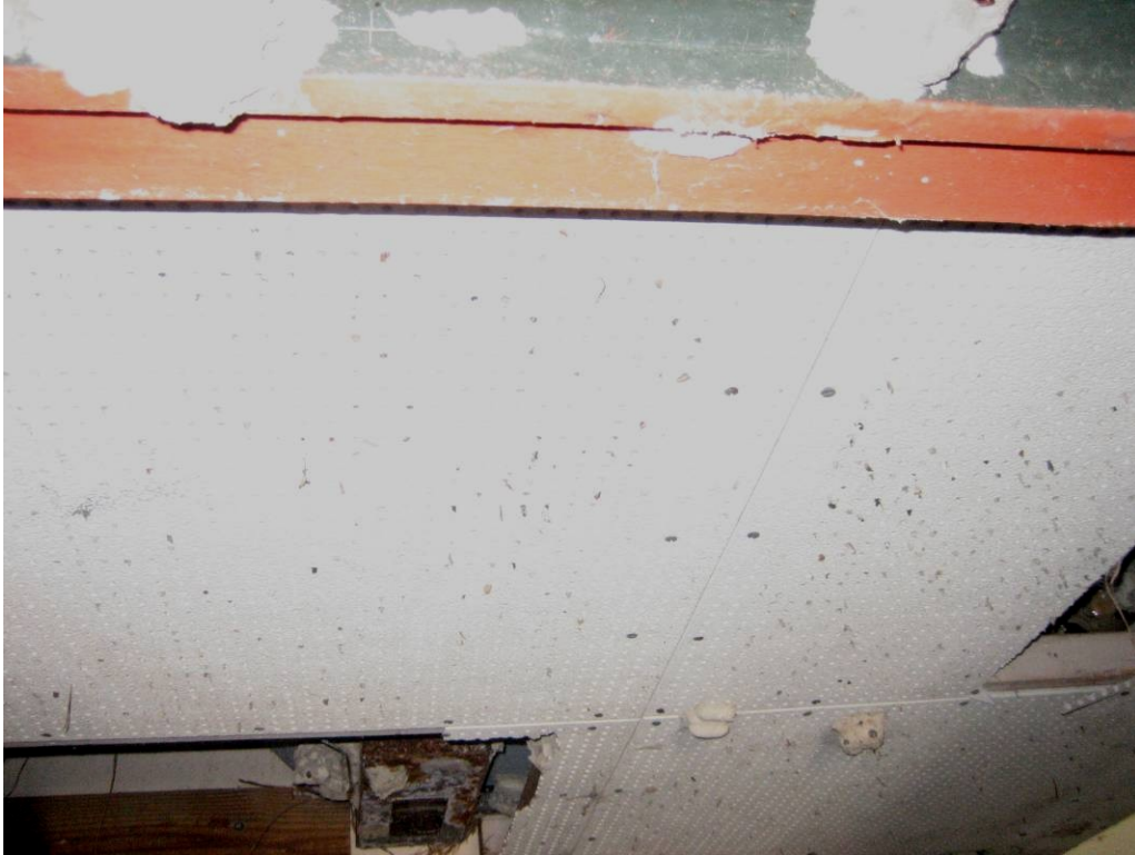
Fire-control Bunker C: ACM interior cementitious ceiling tiles.
