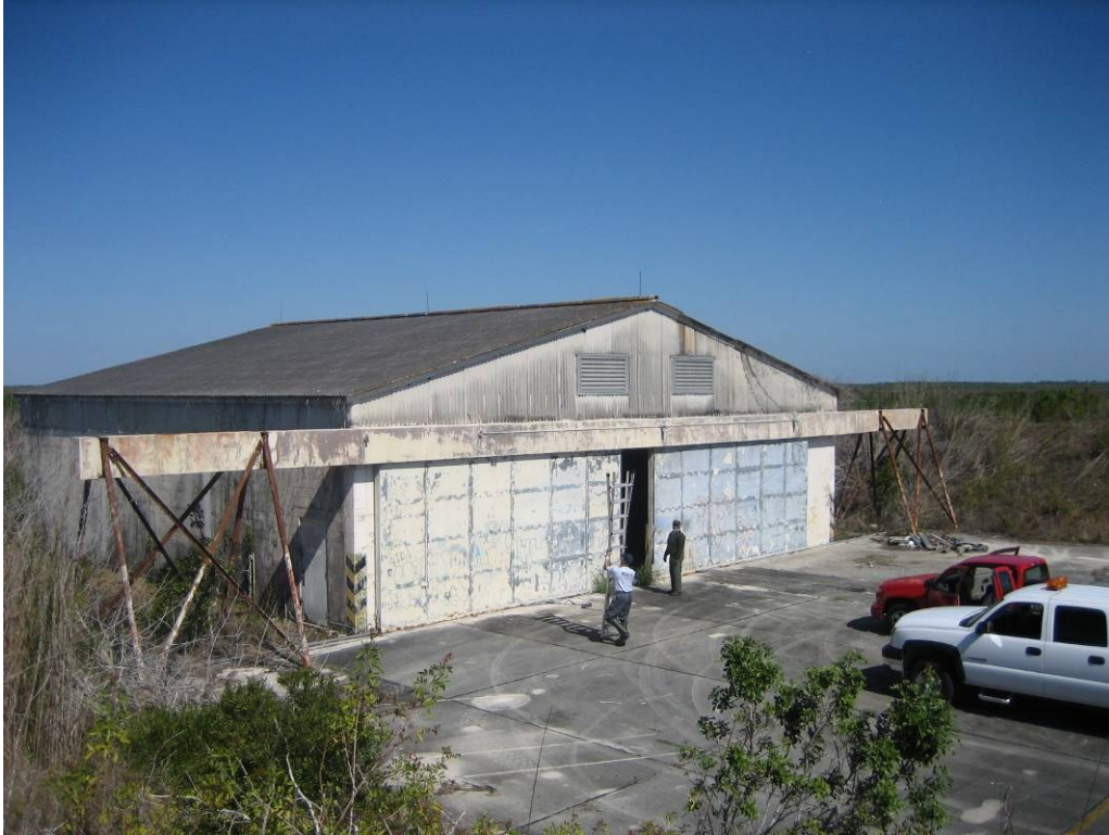
Missile Barn A: ACM exterior cementitious siding and roofing panels.
