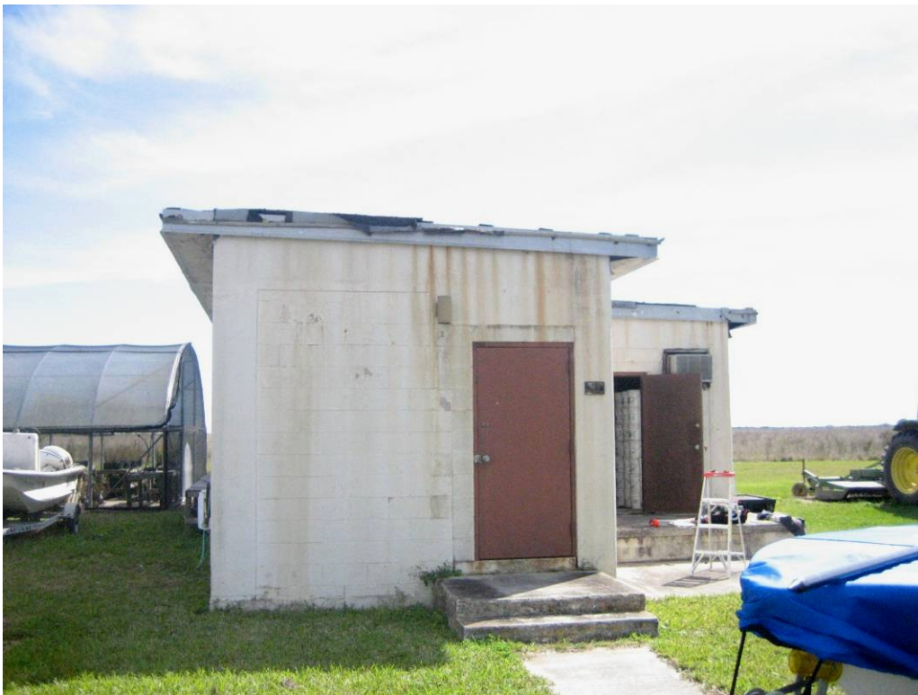
190 B Building in Admin/Control Area.
