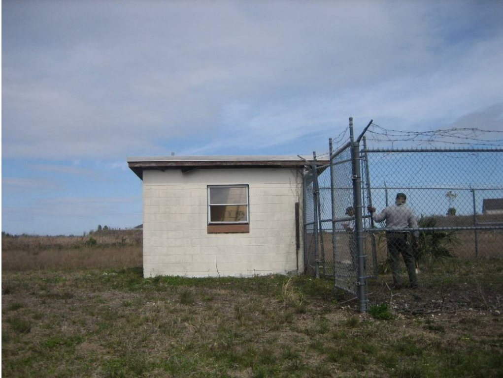
Kennel Building exterior.
