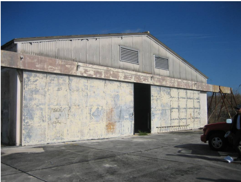
Missile Barn B: ACM exterior cementitious siding and roofing panels.
