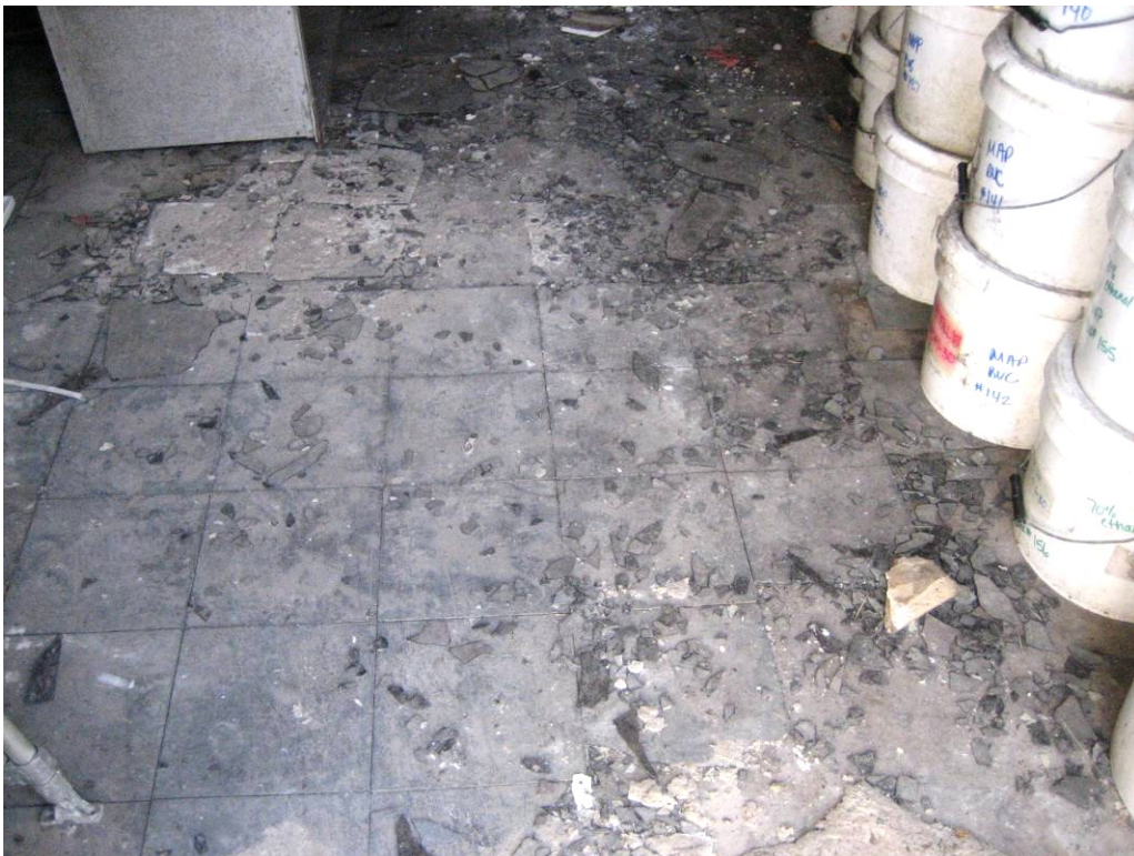
190 B Building: West side ACM 9" black vinyl floor tile and mastic.
