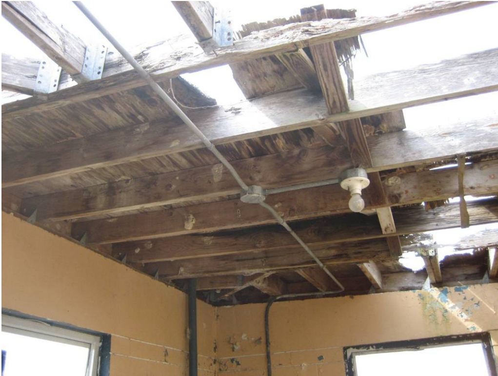
Kennel Building: NonACM roofing material.
