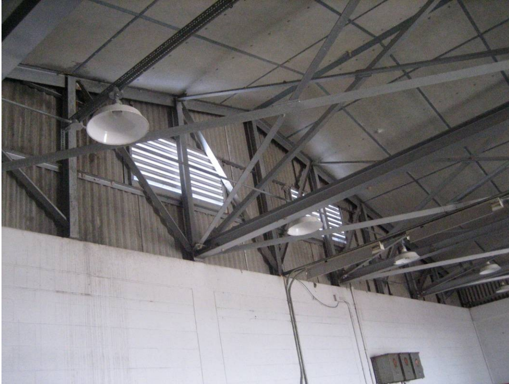
Missile Barn B: ACM interior cementitious siding and ceiling panels.
