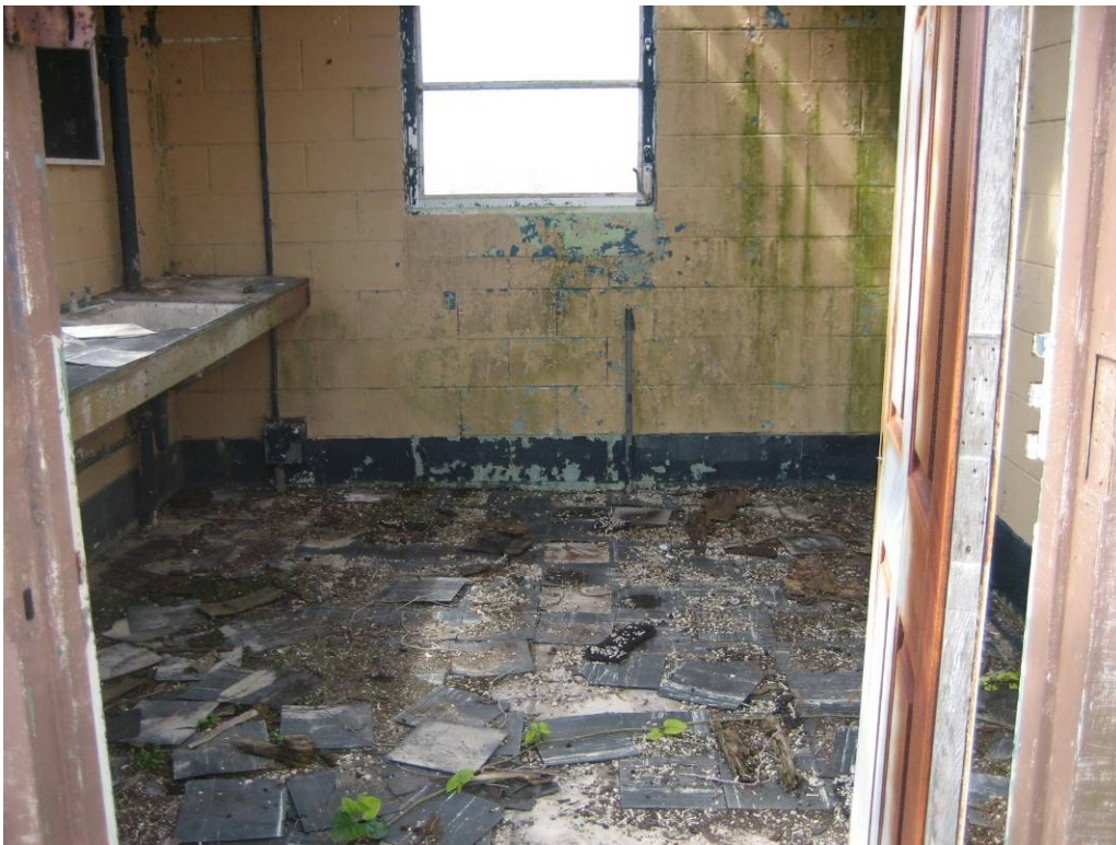
Kennel Building: ACM 9" black vinyl floor tile and mastic.
