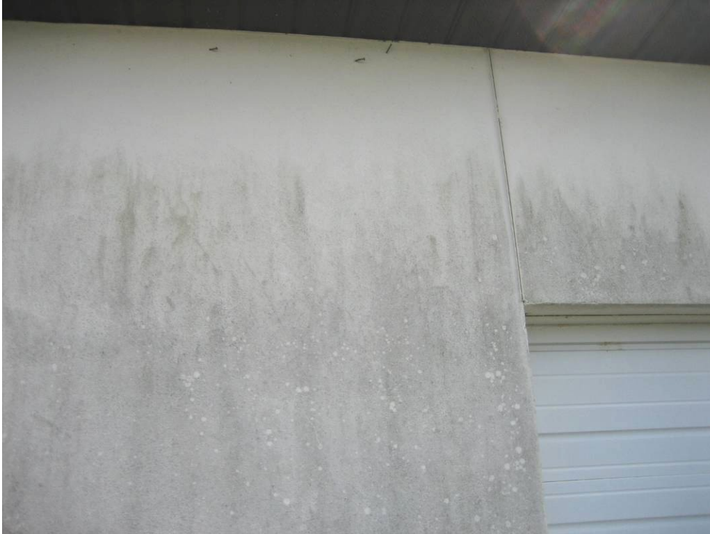
Workshop Building: NonACM exterior stucco.
