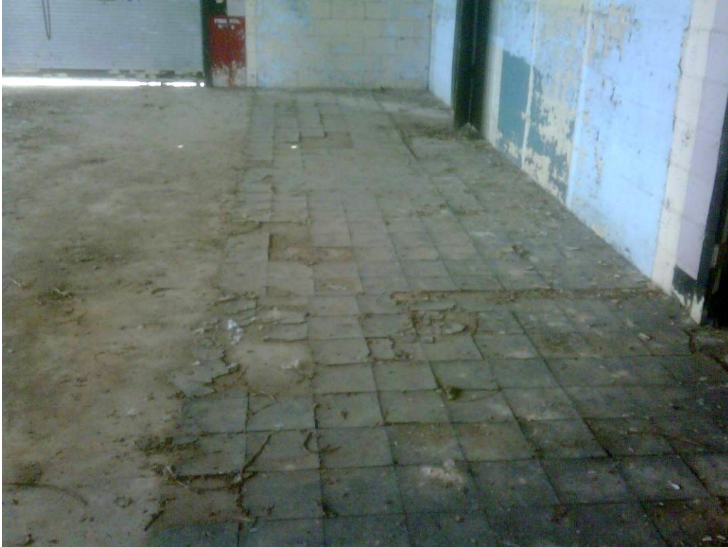
Missile Assembly Building: ACM 9" black vinyl floor tile and mastic.
