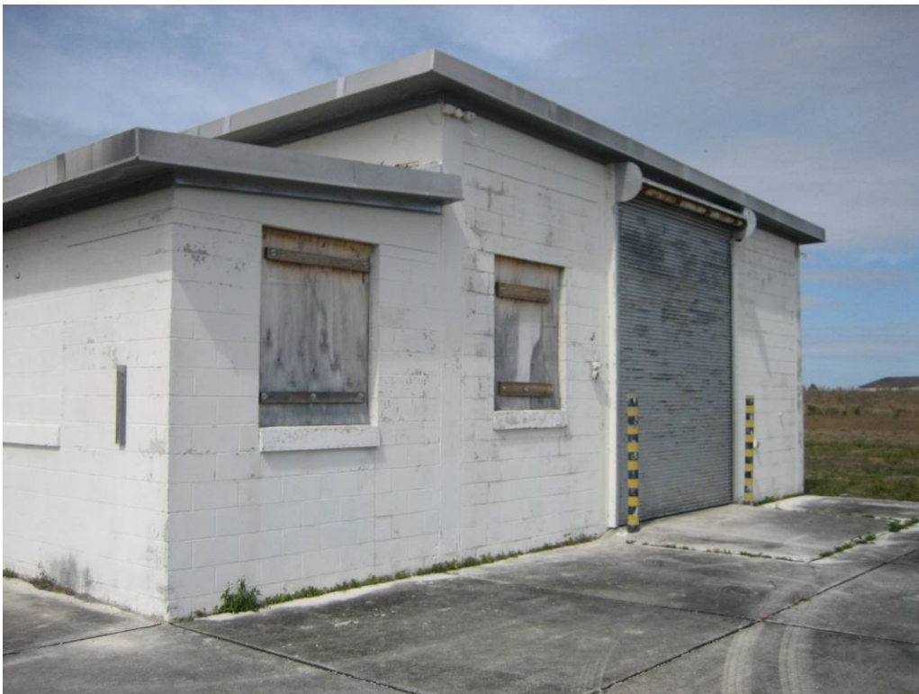
Missile Assembly Building exterior view.
