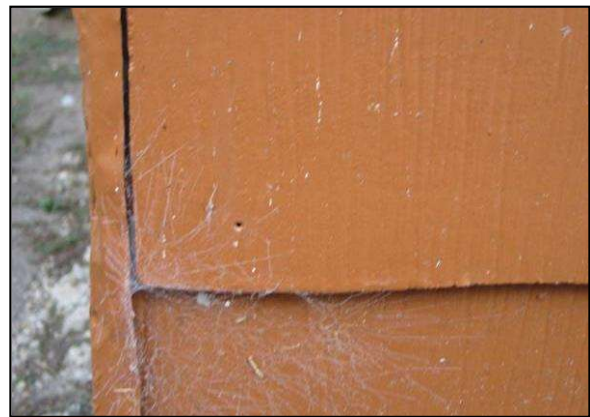
Figure 16 – Detail of nail holes, southeast corner
