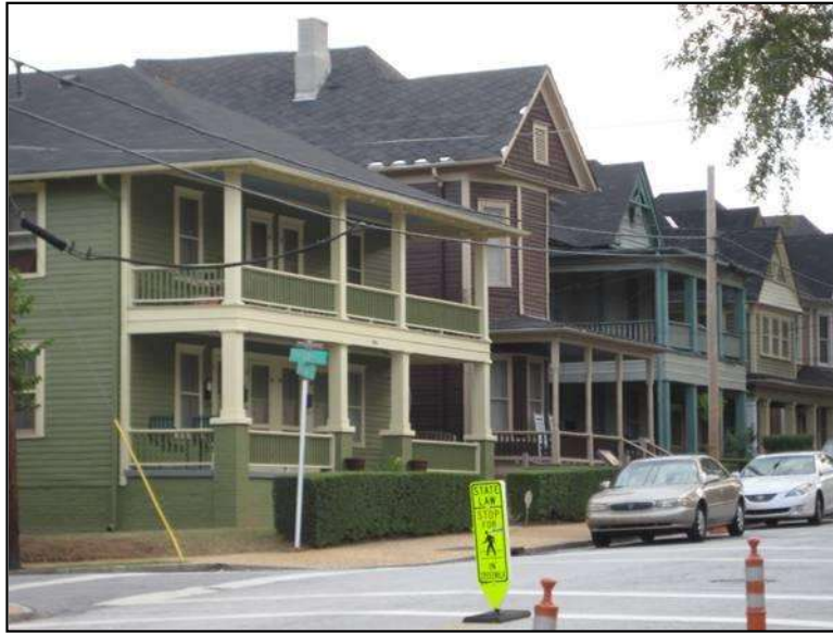
Figure 2 – North side Auburn Avenue streetscape, MLK District
