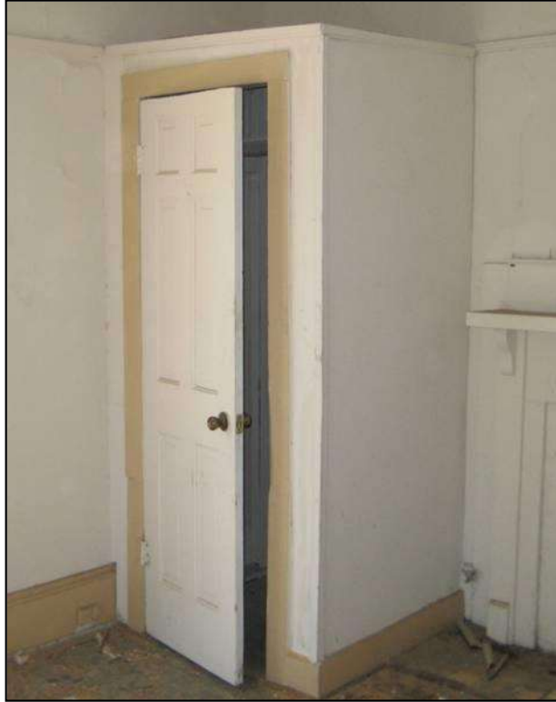
Figure 22 – Non-historic closet in room 201, southeast
