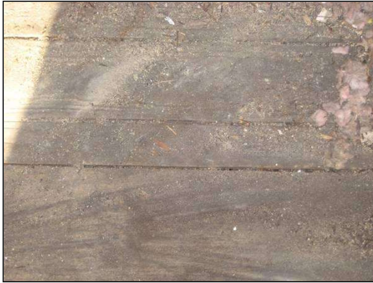
Figure 6 – Detail of typical tongue-and-groove wood, room 202
