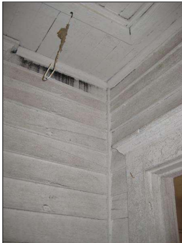
Figure 4 – Historic clapboard shown in room 205, northwest
