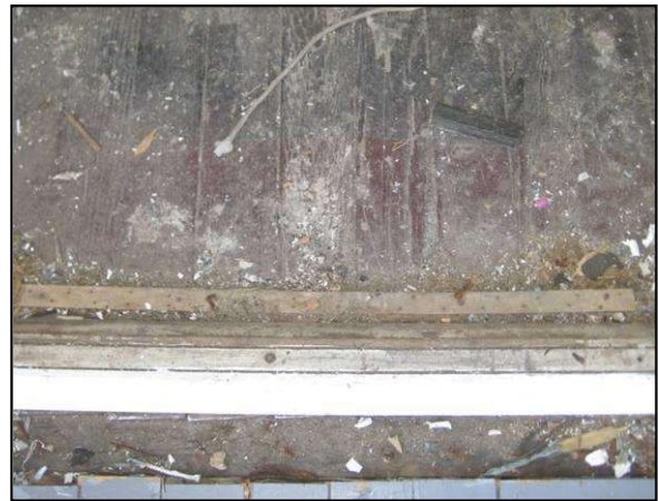
Figure 8 – Detail of furring strip in room 101
