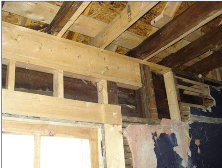
Figure 5 – Example of repairs by NPS in room 207, west wall (courtesy of Holly Schwarzmann)
