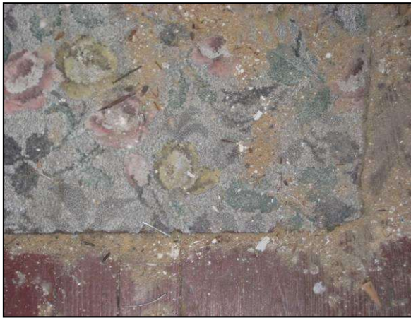
Figure 7 – Detail of vinyl in room 201
