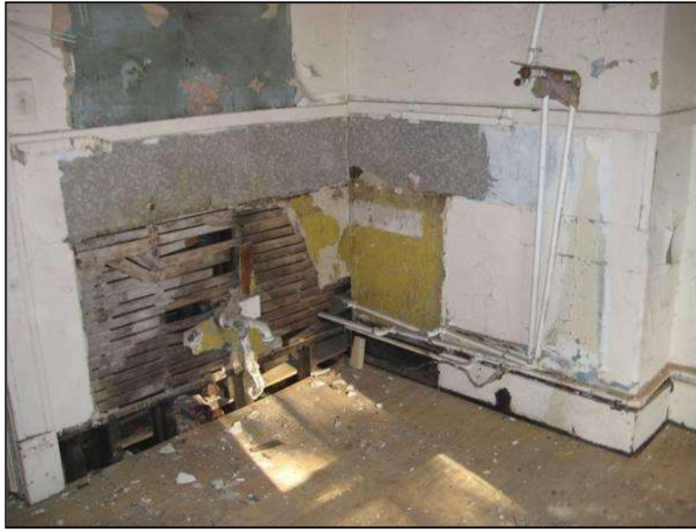
Figure 12 – Room 204 appliance lines, northwest wall
