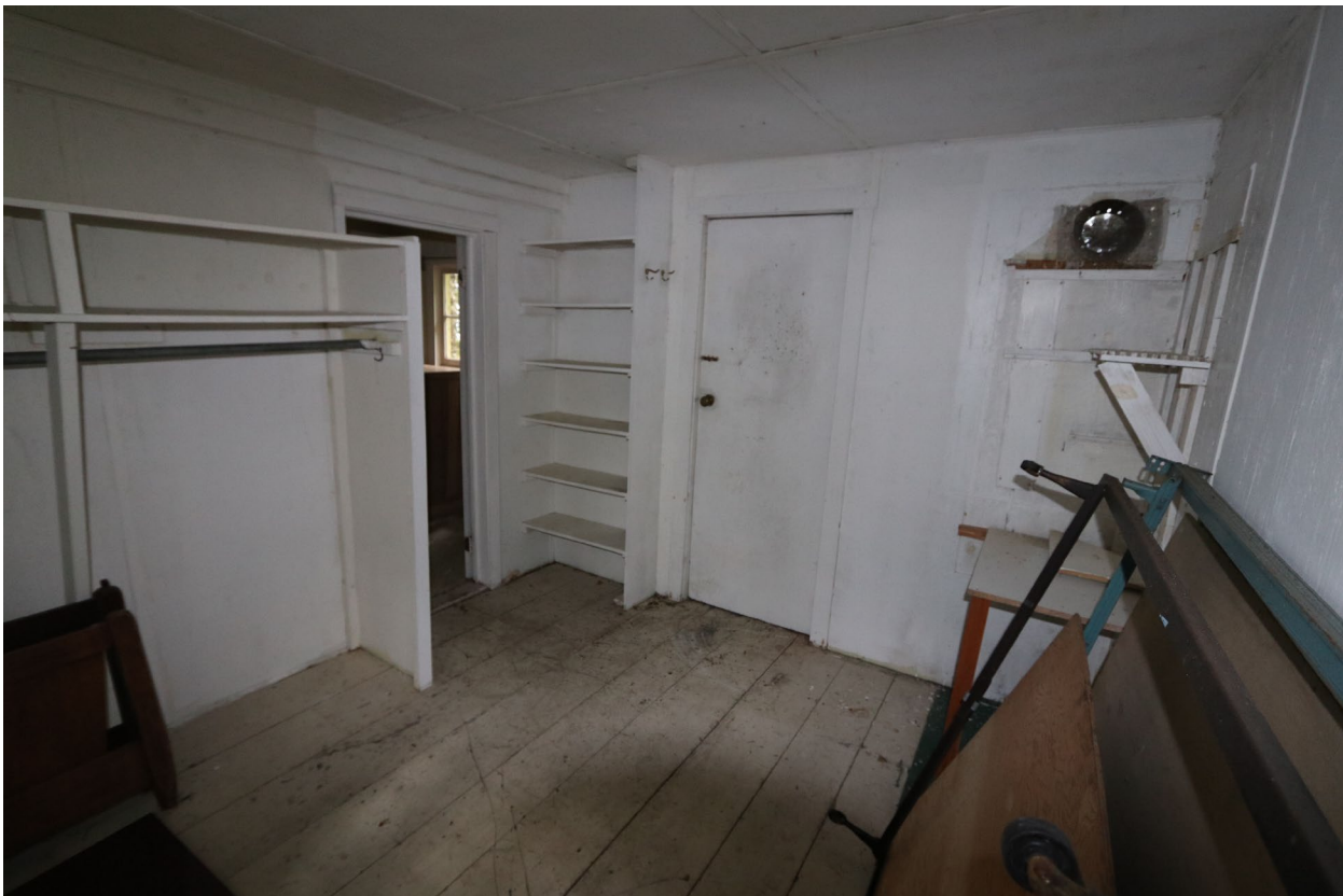
Photo 10. Lagoon Island Cabin, Interior Room 3, NPS Historic Architecture Program, 2018
