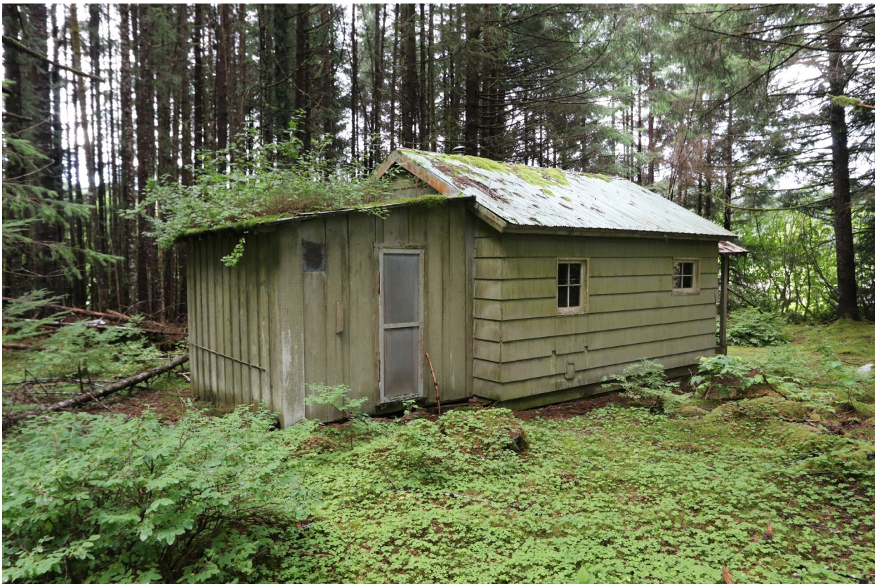
Photo 6: Lagoon Island Cabin, Toward South, NPS Historic Architecture Program, 2018
