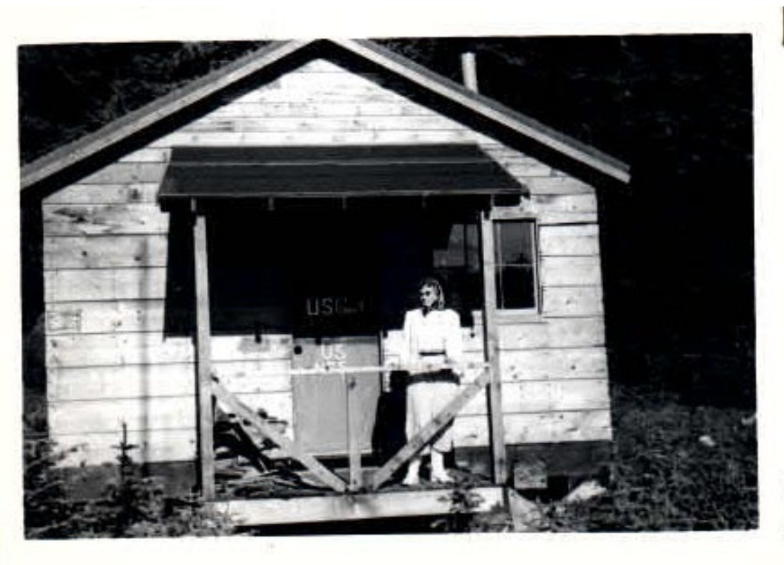
Figure 4. Southwest elevation, view towards northeast. Front elevation shows one window and what appears to be the original door with U.S. government markings. 1951, NPS Photo.
