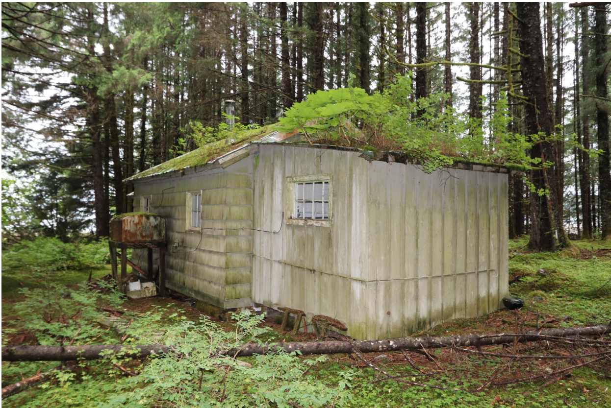
Photo 5: Lagoon Island Cabin, Toward West, NPS Historic Architecture Program, 2018
