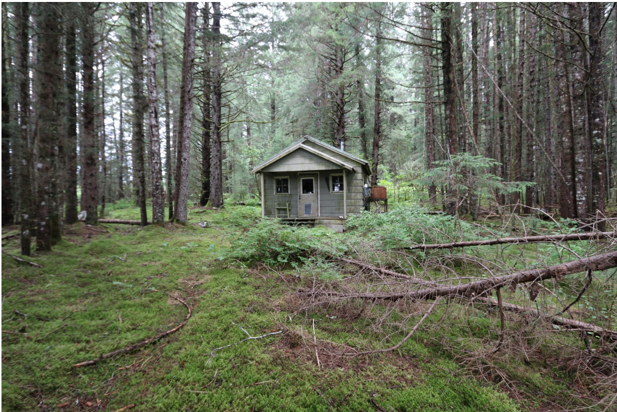
Photo 1: Overview of Lagoon Island Cabin, Toward Northeast, NPS Historic Architecture Program, 2018
