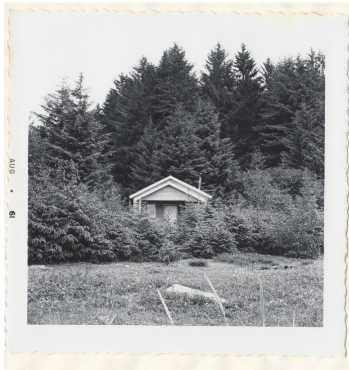
Figure 9. Southwest elevation, view towards northeast. Gable roofed porch visible. 1961. NPS Photo.
