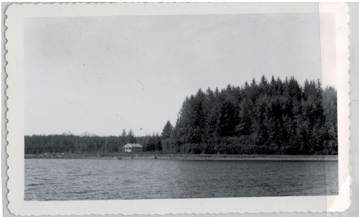
Figure 10. Undated, Cabin front elevation with flag pole, NPS Photo.
