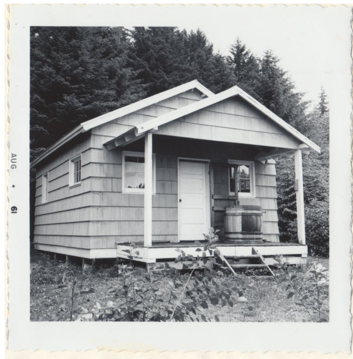
Figure 8. West and southwest elevations, view towards northeast. Windows visible on west elevation. Two windows visible on the southwest elevation. Water storage barrel on porch. 1961, NPS Photo.
