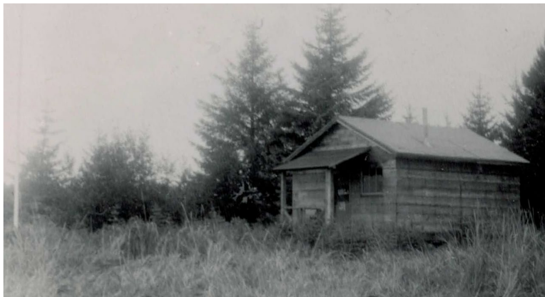
Figure 6. South and east elevations, view towards north. No windows on east elevation, one window on porch, shed roof porch. 1951, NPS Photo.
