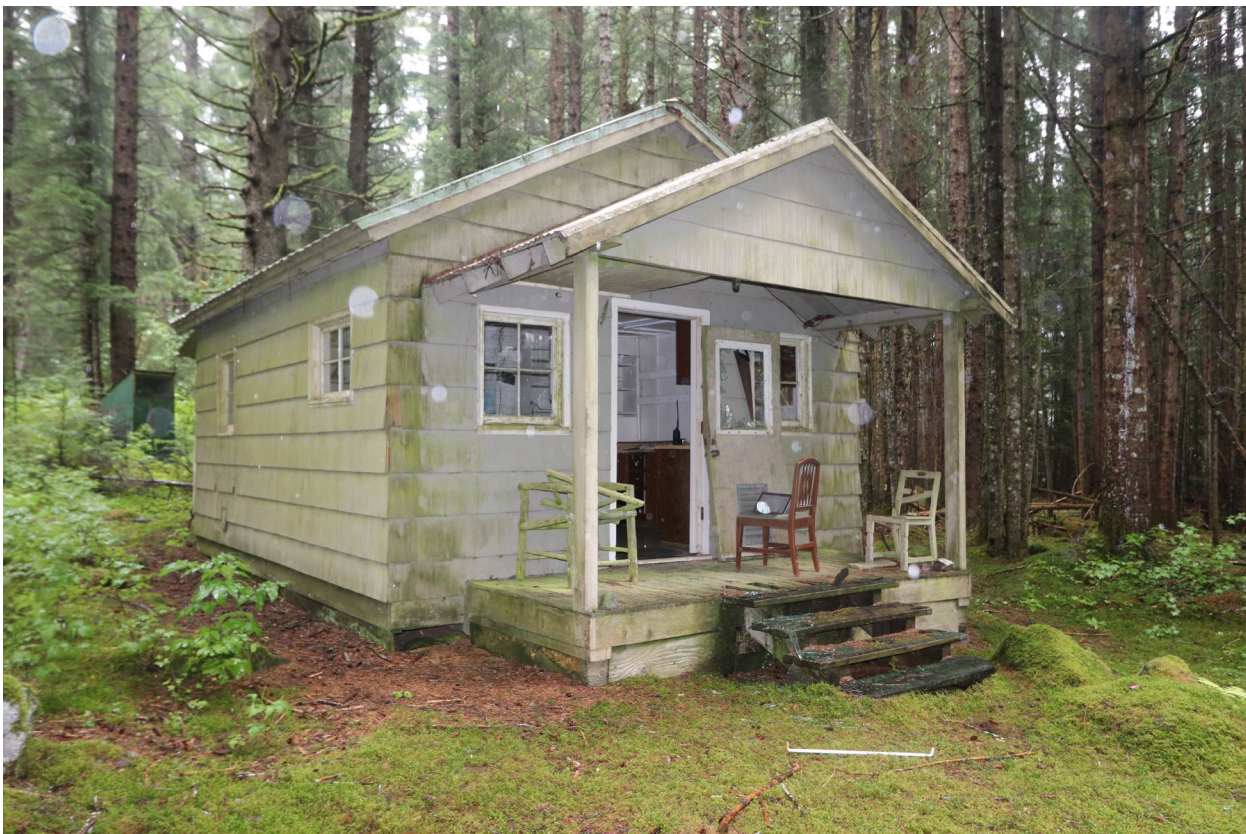
Photo 2: Lagoon Island Cabin, Toward East, NPS Historic Architecture Program, 2018
