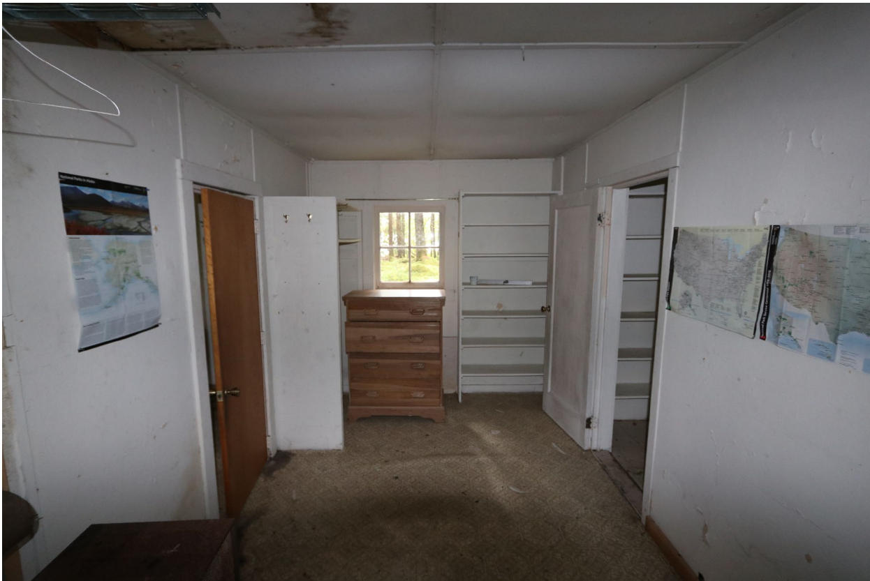
Photo 9. Lagoon Island Cabin, Interior Room 2, NPS Historic Architecture Program, 2018
