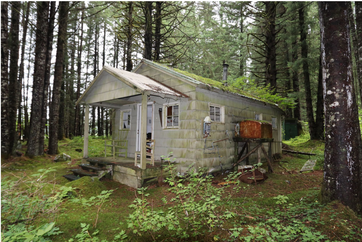
Photo 3: Lagoon Island Cabin, Toward North, NPS Historic Architecture Program, 2018
