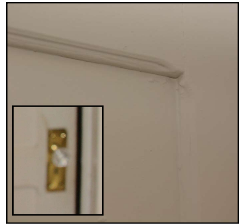
Figure 26: Detail of lamb's tongue chamfer. Inset shows detail of brass-plated escutcheon plate and glass knob. Photos by author, 2020
