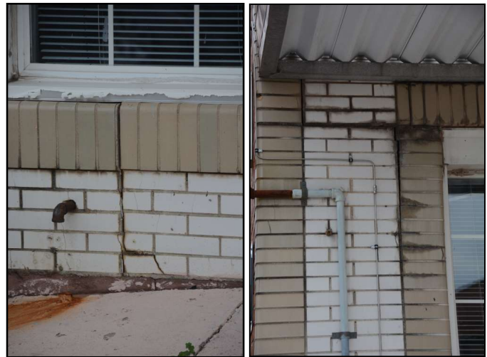
Figure 14: Cracking and water staining in the white and tan brick veneer on the east elevation. Left is below the Gurnee Avenue-facing window and right is left of the same window's header. Photo by author, 2020.
