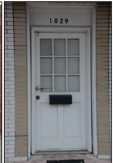
Figure 17: 1029 Gurnee Avenue front door. Photo by author, 2020.
