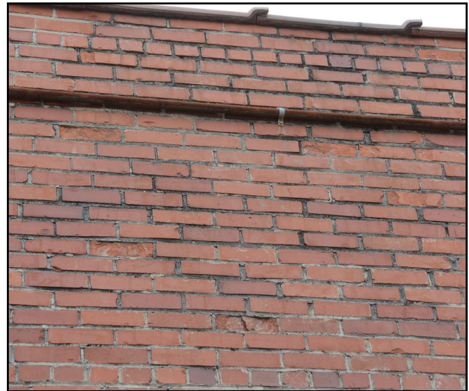
Figure 15: Some brick face spalling and wetness is evident on the upper portion of the north elevation. Photo by author, 2020.
