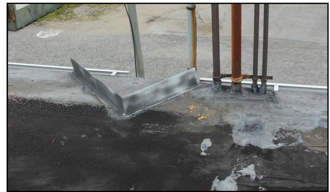
Figure 21: A roof cricket at rear of building between 1029 and 1025 Gurnee Avenue roofs divides water flow between the two building's gutters. Photo by author, 2020.
