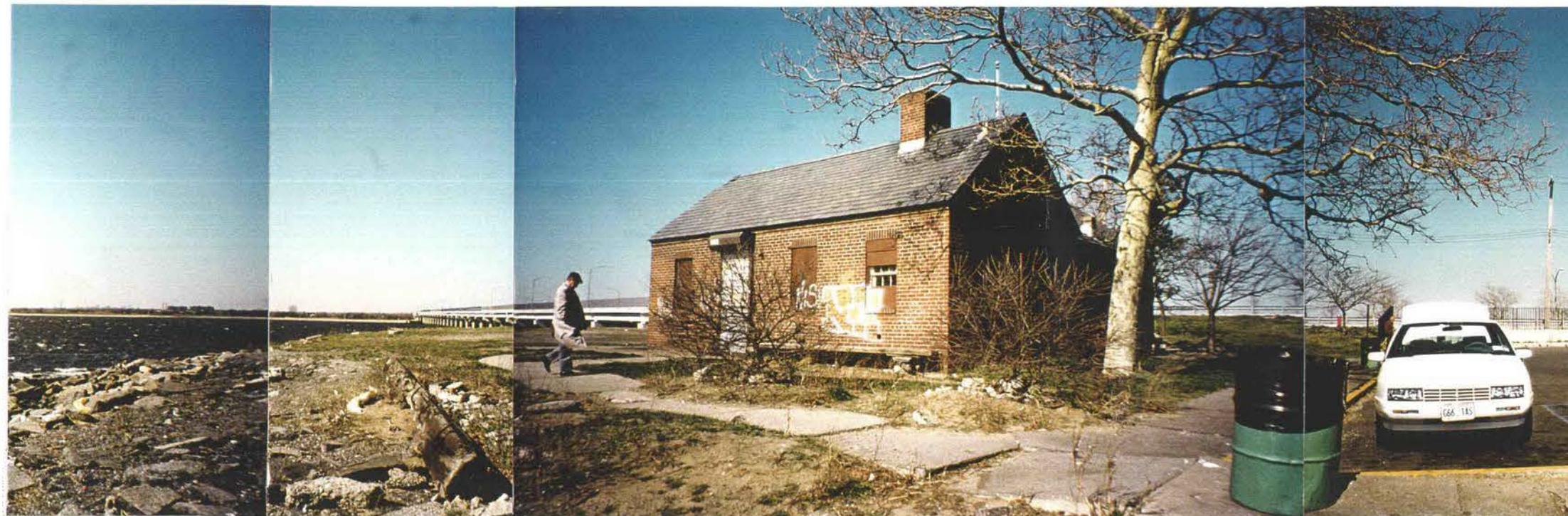
View From Southwest
