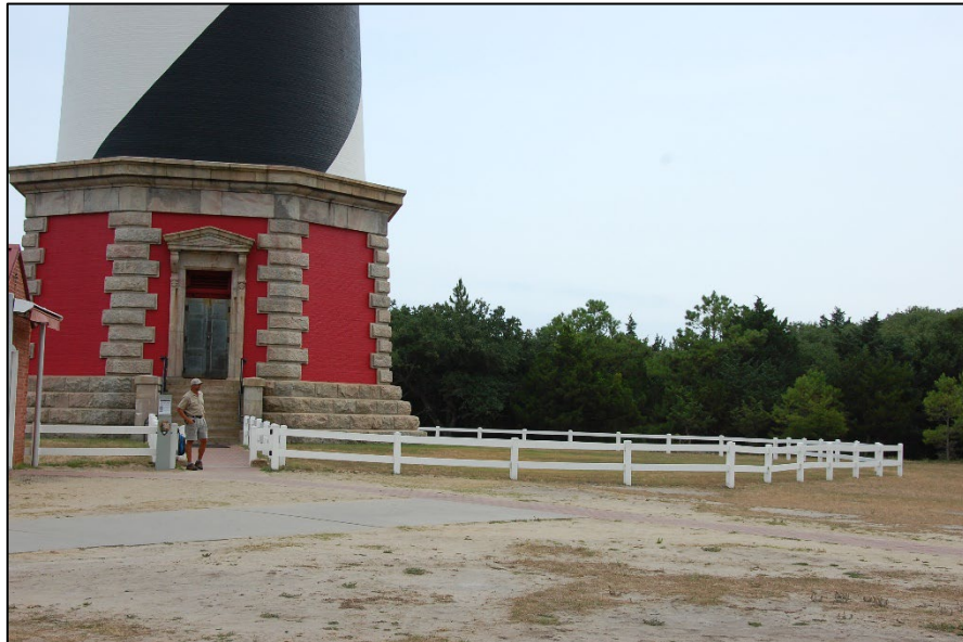
Fig 12. Reconstructed fencing around lighthouse, 2015
