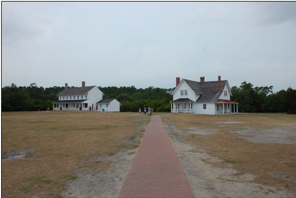
Fig 8. View of Keepers' Quarters, 2015
