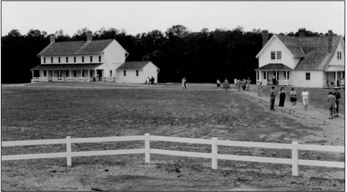
Fig. 7. View of Keeper's Quarters (2001)
