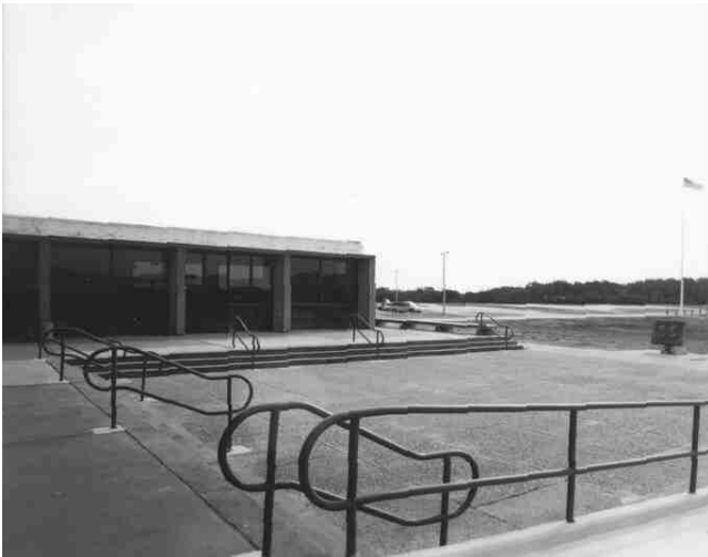
Fig 38. Handicapped rails and concrete repairs, 2000
