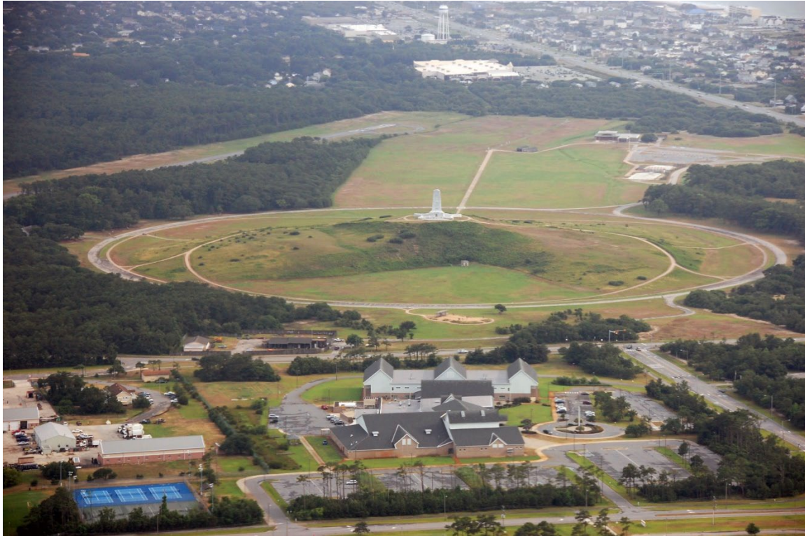
Fig 35. View of monument and powerhouse with Superintendent's quarters and maintenance complex, 2015
