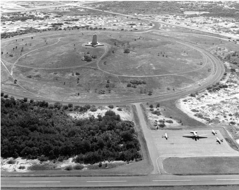
Fig 21. Aerial view of the airstrip, 1969
