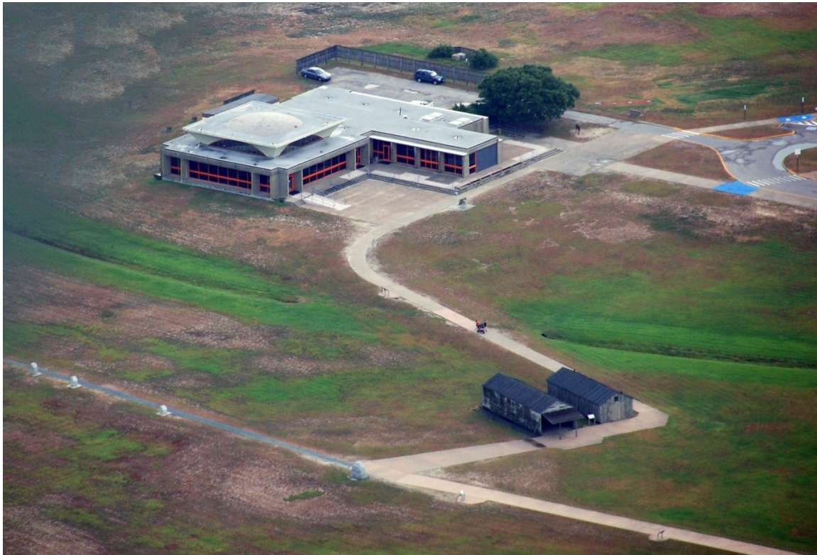
Fig 57. Aerial view of visitor center area, 2015
