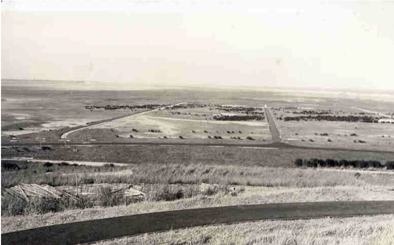
Fig 54. View of the mall showing drainage swales, 1936
