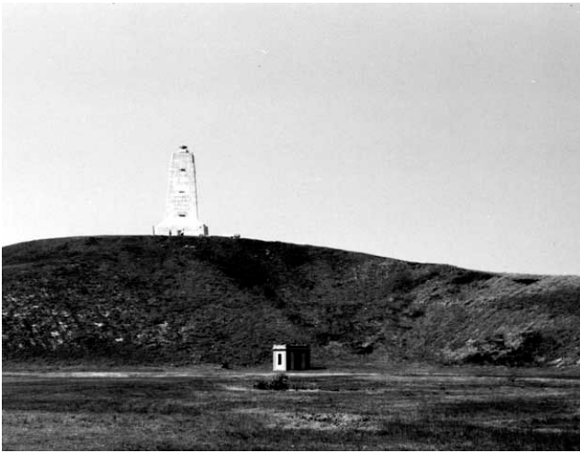
Fig 33. Monument and powerhouse, 1994
