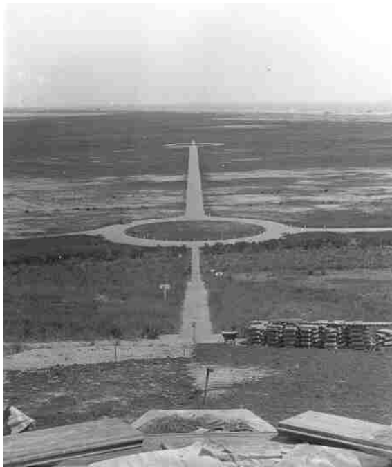
Fig 12. Boulder Road construction, 1931
