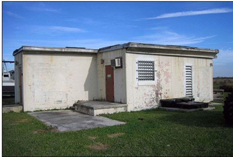
Fig 64. West elevation of the interconnecting corridor building. Source: WJE, 2010
