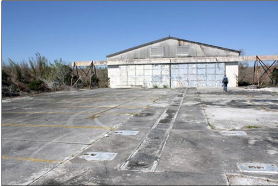
Fig 53. Launch pad, with remains of the missile-moving track. Source: JMA, 2010
