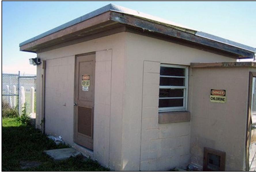
Fig 61. View from northwest of the pumphouse. Source: WJE, 2010
