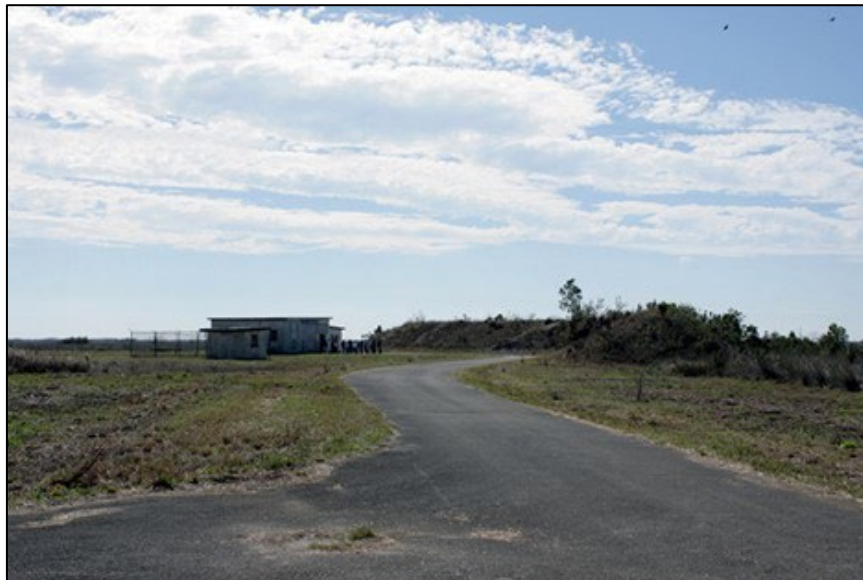
Fig 19. The crescent-shaped berm adjacent to the missile assembly and test building. Source: JMA, 2010
