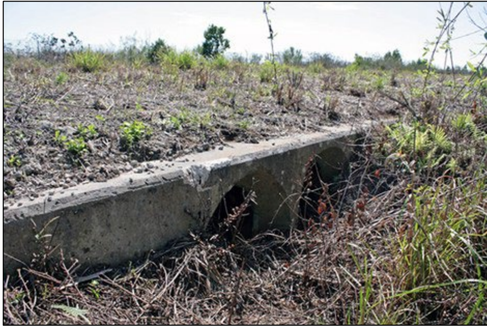
Fig 83. A drainage structure with a double pipe elevation. Source: JMA, 2010
