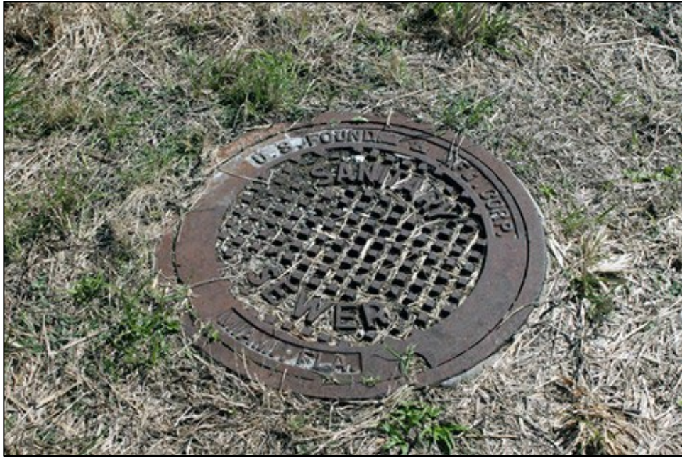
Fig 116. Manhole covers in the Launch Area. Source: JMA, 2010
