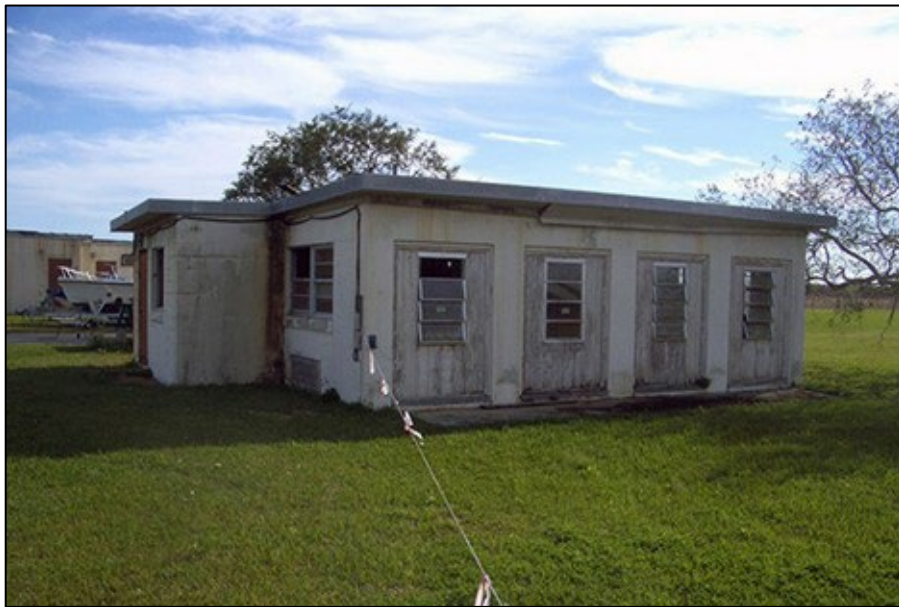
Fig 62. North elevation of the generator building. Source: WJE, 2010
