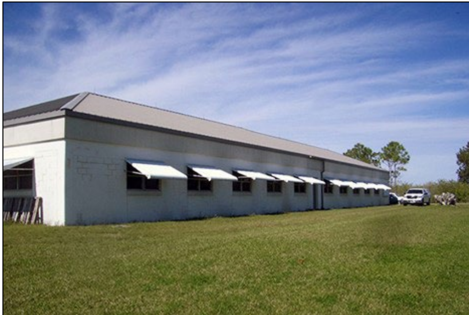
Fig 58. East elevation of the administration and barracks building. Source: WJE, 2010
