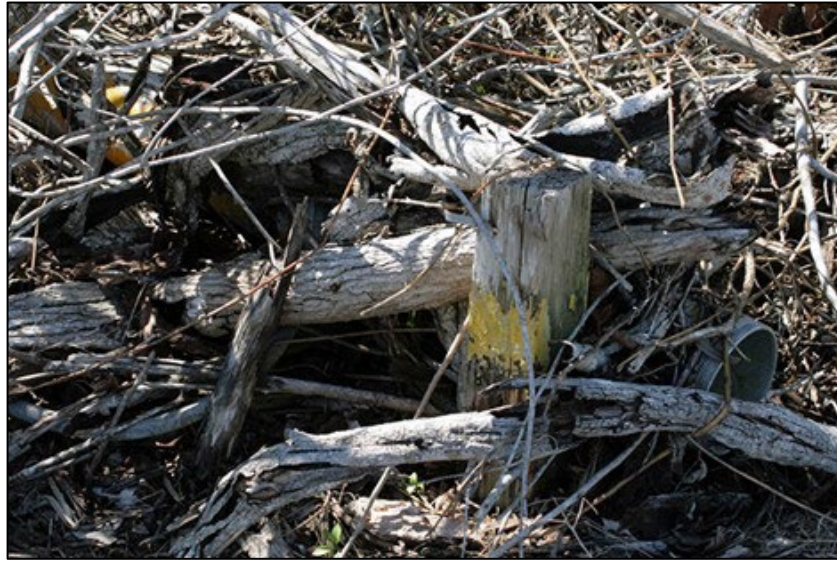
Fig 114. Painted wood post located near conduit pipe was likely used as support for the pipes. Source: JMA, 2010.
