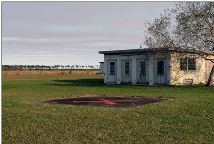
Fig 46. One non-historic helipad is located north of the generator building. Source: JMA, 2010.
