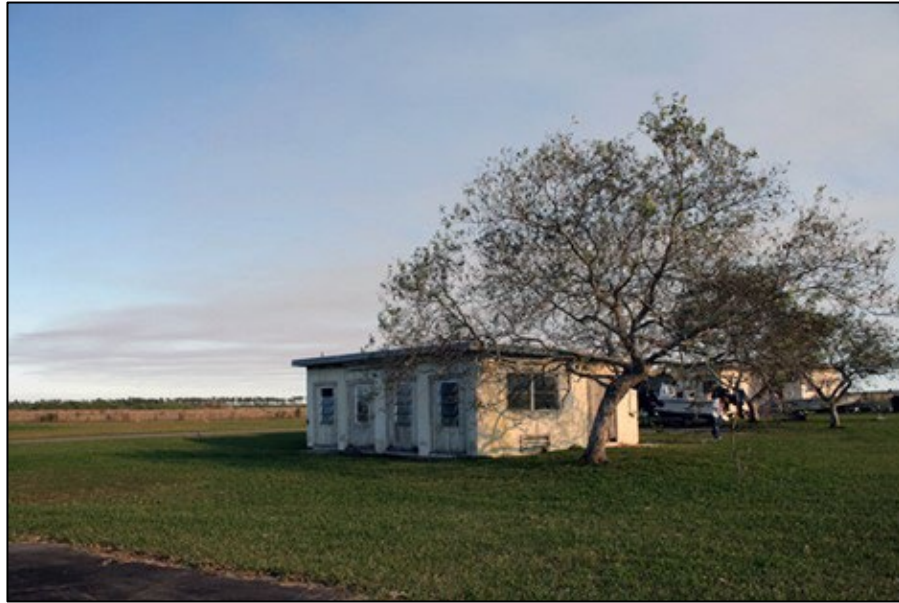
Fig 31. False tamarind ( lysoloma ) located at the southwest side of the generator building. Source: JMA, 2010
