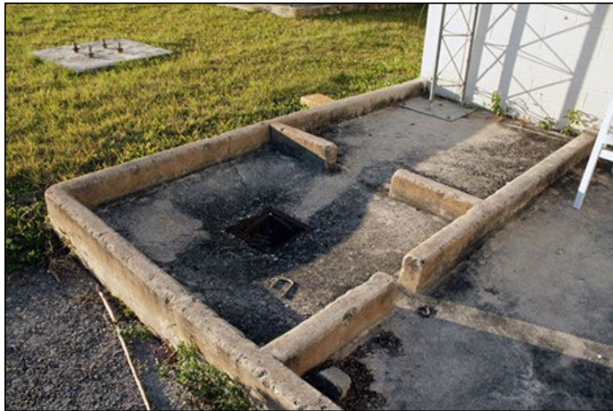
Fig 84. Concrete feature adjacent to the administration and barracks building, identified as a mop basin. Source: JMA, 2010
