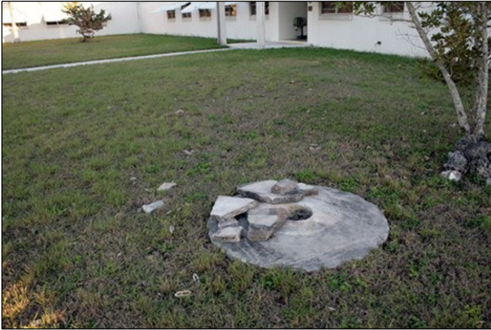
Fig 100. Concrete flagpole base. Source: JMA, 2010
