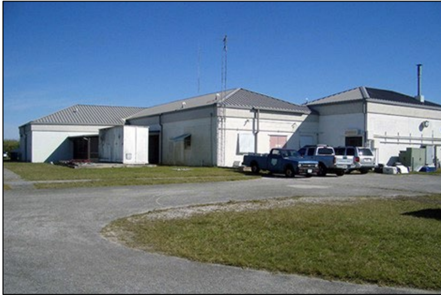
Fig 59. Southwest elevation of administration and barracks building. Source: WJE, 2010
