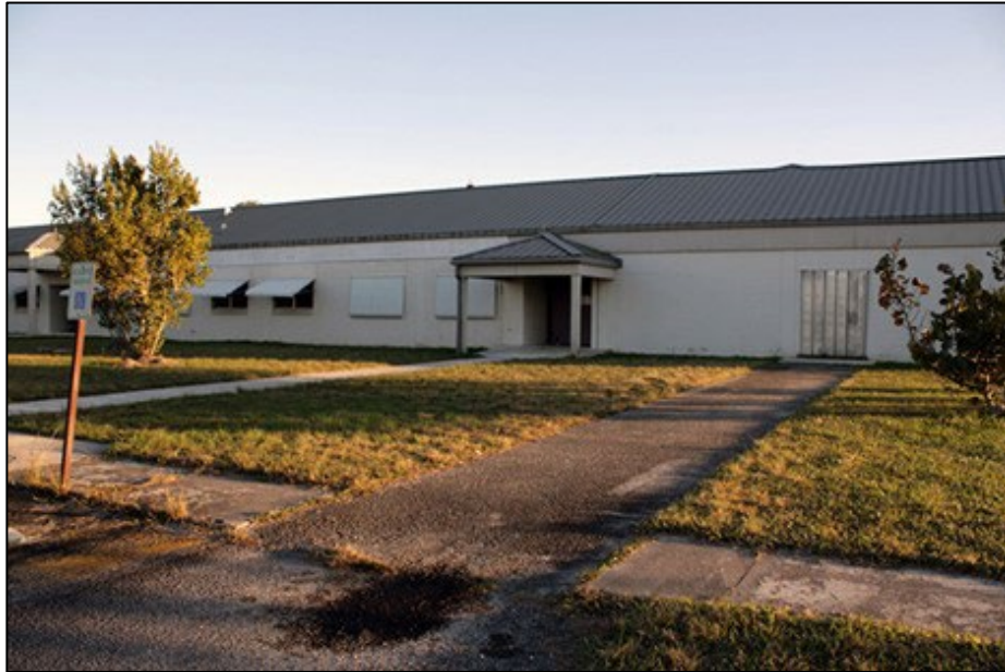
Fig 41. Asphalt and concrete sidewalks in front of the administration and barracks building. Source: JMA, 2010.
