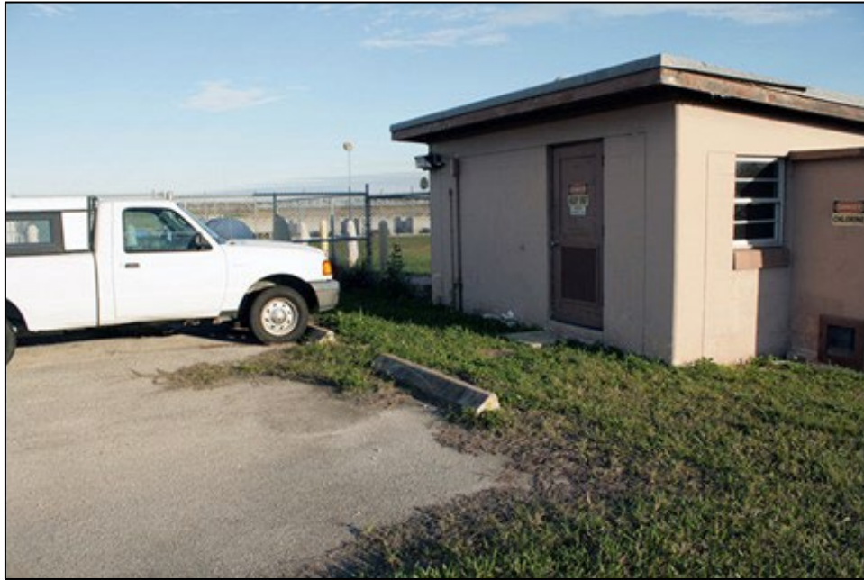
Fig 102. Wheel stops near the pumphouse. Source: JMA, 2010
