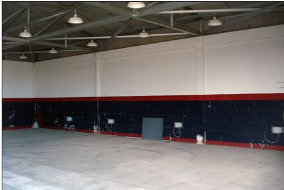
Fig 72. Interior of missile shelter building B with curve-faced wall-mounted light fixtures. Source: WJE, 2010
