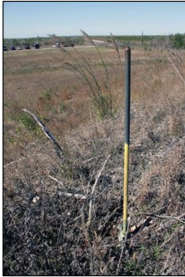
Fig 118. Lightning rods are placed at regular intervals along the ridge of each berm. Source: JMA, 2010
