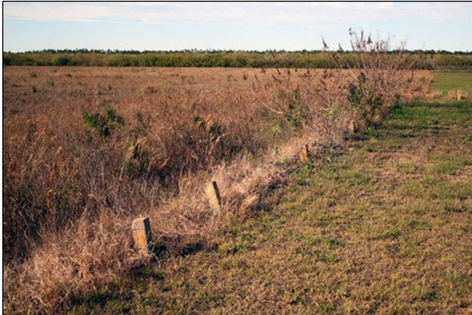
Fig 98. Concrete posts line the south and west sides of the septic field. Source: JMA, 2010.
