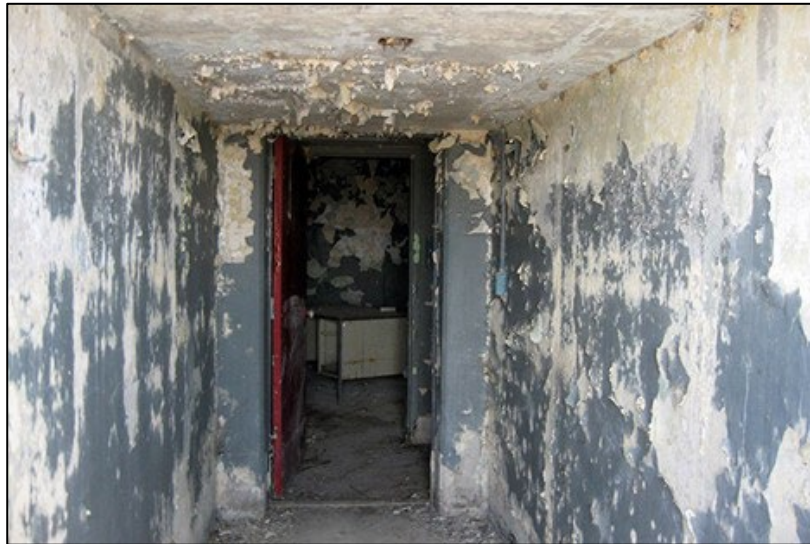
Fig 78. Interior of entry vestibule at bunker A. Source: WJE, 2010
