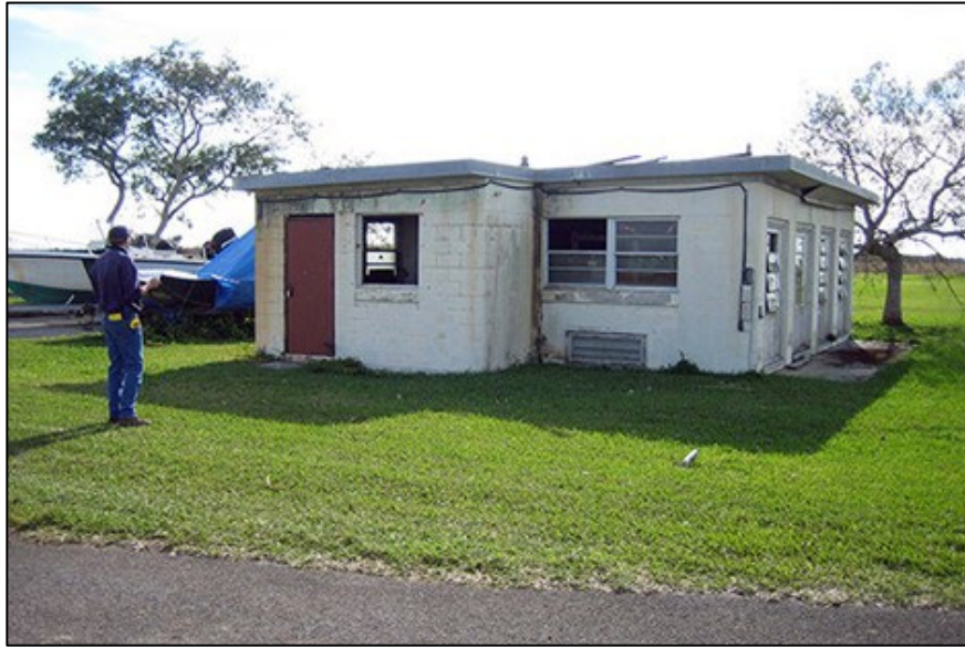
Fig 63. East elevation of the generator building. Source: WJE, 2010
