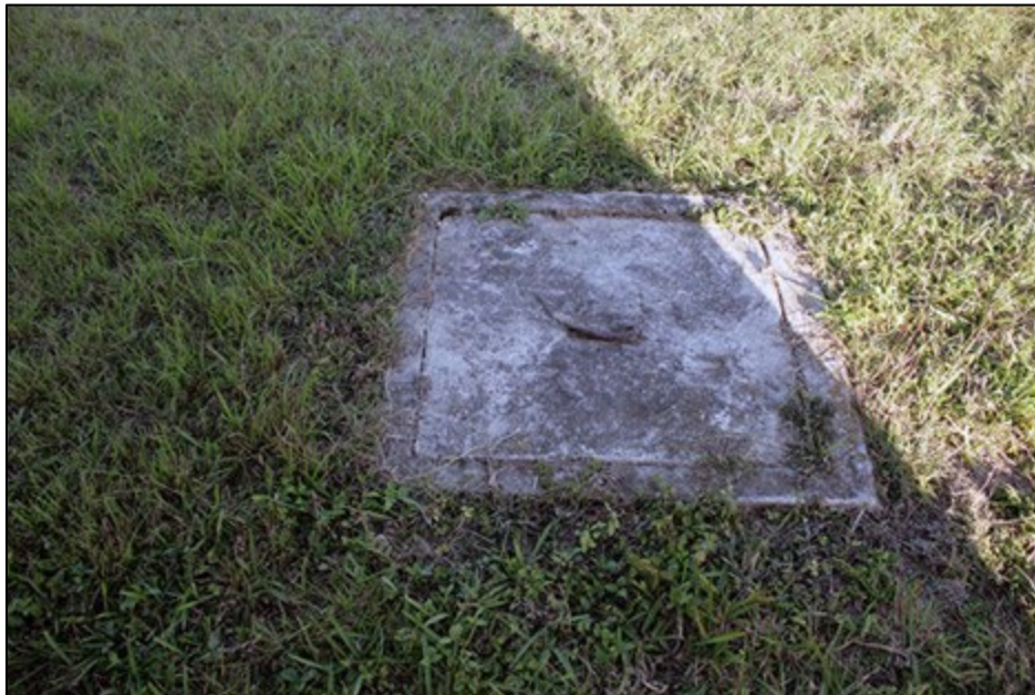
Fig 101. Concrete feature with concrete cover and metal handle. Source: JMA, 2010
