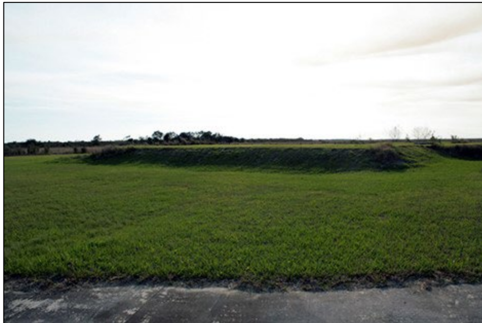
Fig 17. The sewage drainfield in the Control Area. Source: JMA, 2010
