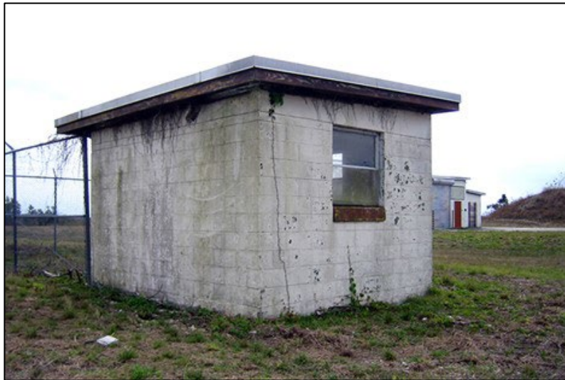
Fig 82. View from northwest of canine support building. Source: WJE, 2010
