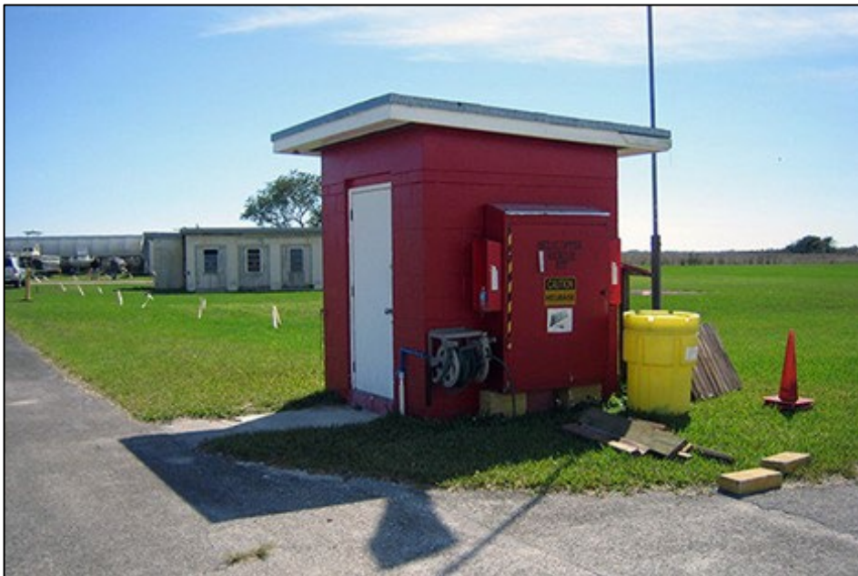
Fig 60. North elevation of the paint and oil storage building. Source: WJE, 2010
