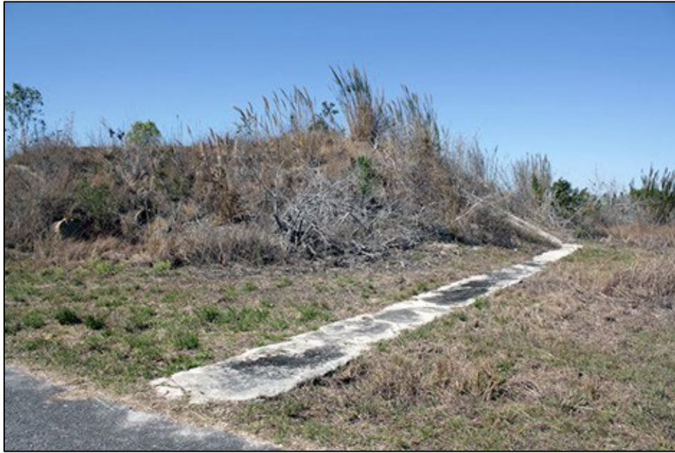
Fig 55. Concrete sidewalks lead from the loop road to each Launcher Section Control Center. Source: JMA, 2010
