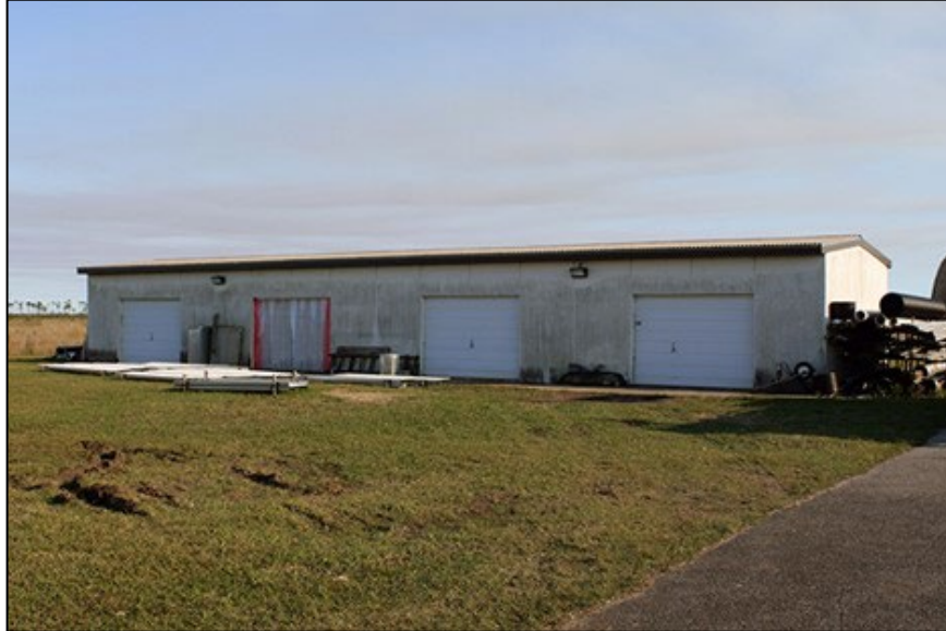
Fig 66. North elevation of the general purpose warehouse. Source: JMA, 2010
