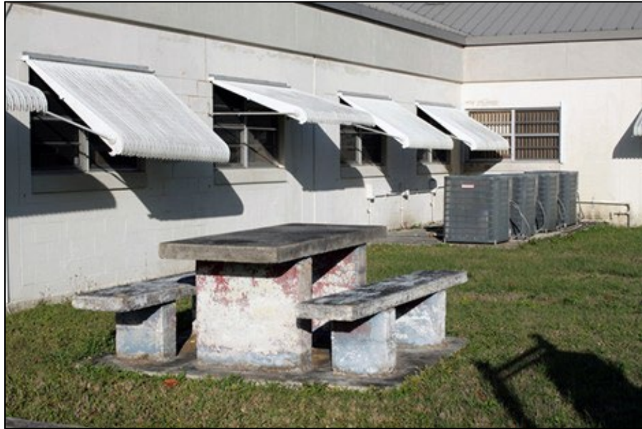
Fig 95. Concrete picnic table and benches located between the research center and athletic court. Source: JMA, 2010
