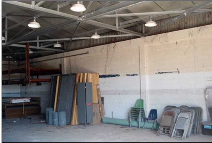
Fig 71. Interior paint coating in missile shelter building A with wood-framed loft. Source: WJE, 2010.
