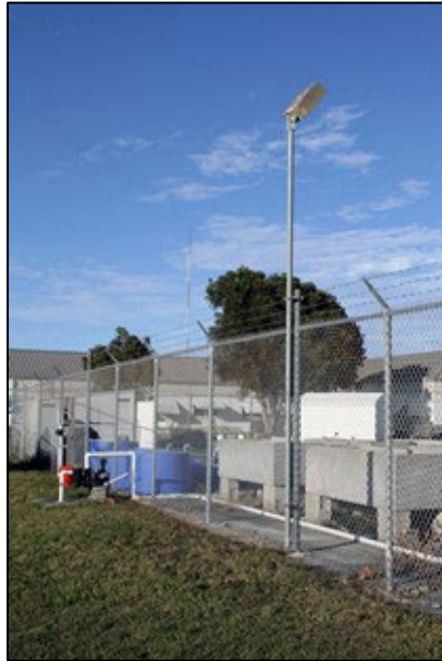
Fig 89. Chain link fence surrounding the former athletic court. A pump and tanks associated with aquatic invertebrate and fish research are also visible. The light pole may be remaining from the period of significance. Source: JMA, 2010
