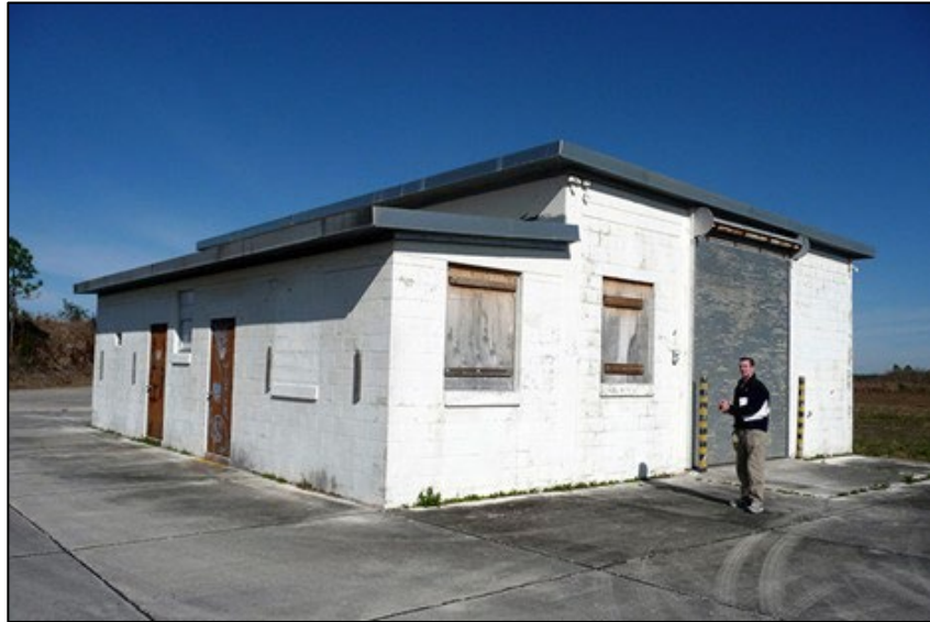
Fig 68. View from the southeast of the missile assembly and test building. Source: WJE, 2010.
