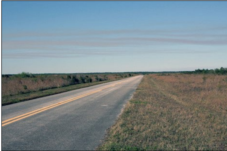
Fig 16. The road connecting the Control and Launch areas. Source: JMA, 2010
