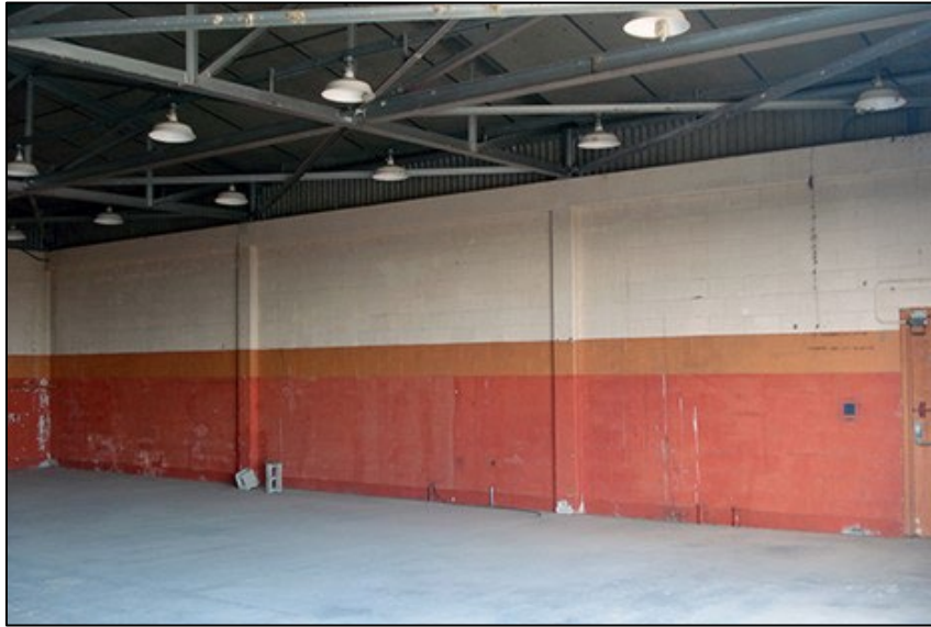
Fig 73. Interior of missile shelter building C. Source: WJE, 2010
