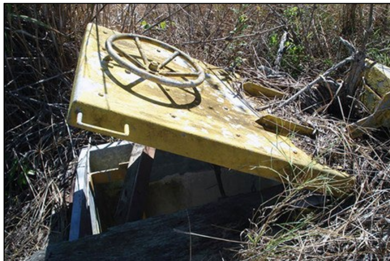
Fig 76. Steel escape hatch for bunkers. Source: WJE, 2010
