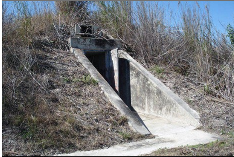
Fig 75. Typical entrance area to bunkers. Source: WJE, 2010
