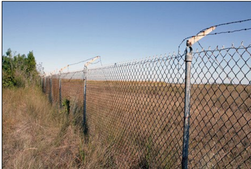
Fig 109. Fence remnant in the Launch Area. Source: JMA, 2010
