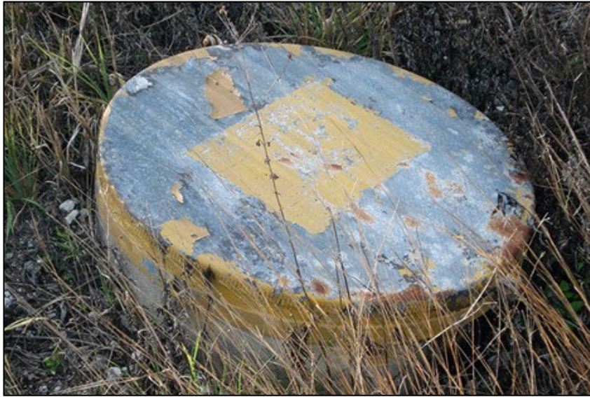
Fig 77. Concrete storage well embedded in earthen berm. Source: WJE, 2010
