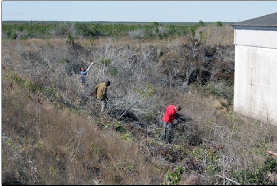
Fig 35. A volunteer program exists to clear the berms of damaging vegetation. Source: JMA, 2010.
