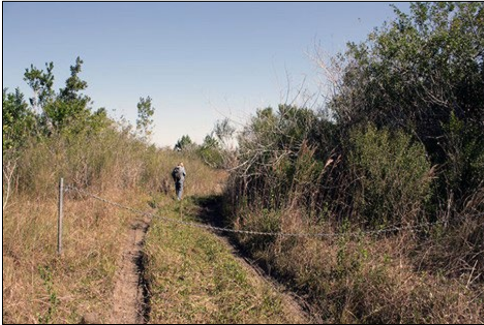
Fig 104. Post and chain fence across the borrow pit road. Source: JMA, 2010
