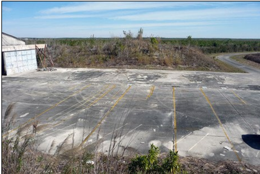
Fig 74. Typical launch pad pavement. Source: WJE, 2010
