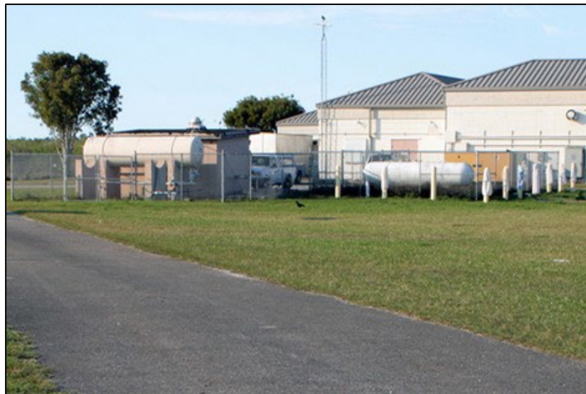
Fig 37. Control Area access road. Note chain link fence and bollards around the pumphouse. Source: JMA, 2010.
