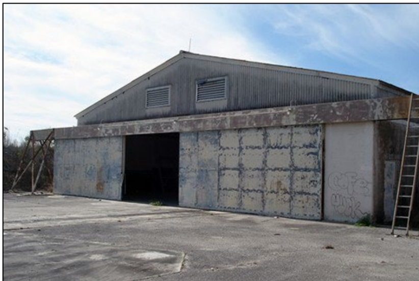
Fig 70. Typical southeast elevation of the missile shelter buildings. Source: WJE, 2010
