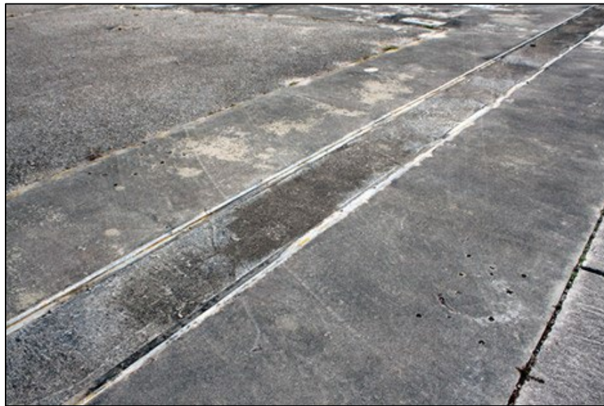
Fig 54. Remains of the missile-moving track, embedded in the concrete launch pad. Source: JMA, 2010
