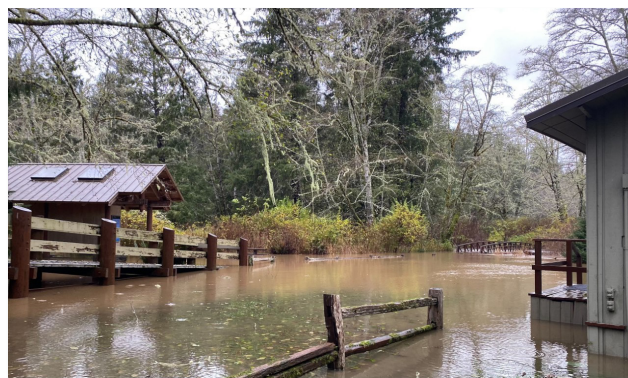
Figure 2. Flood waters from Ozette Lake inundate the Ozette Ranger Station hiker's kiosk and Coal Creek bridge in late November 2021.
