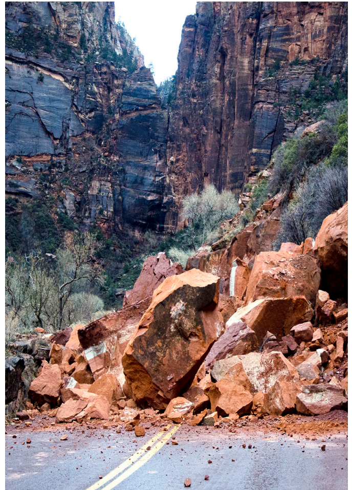
GIP Justin LaForge evaluating a potential rockfall slope in Zion Canyon, Zion National Park, Utah (left photograph). Rockfall that closed the Scenic Drive in Zion Canyon that was assessed by Justin LaForge prior to failure (right photograph). (NPS photos)
