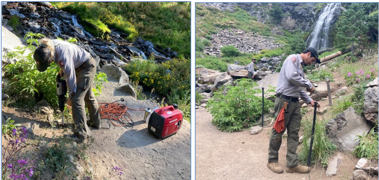
Figure 11. Installation of fence post receivers (left). Installation of fence posts, chain, and signage along the trail edge (right). Photos by Carrie Wyler.
