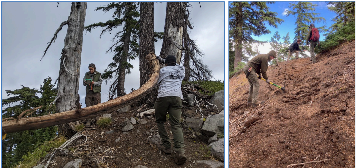
Figure 14. Placing locally available woody debris to block access to visitor-created trails and trampled areas (left); decompacting large heavily trampled areas ahead of planting. Photos by Carrie Wyler.
