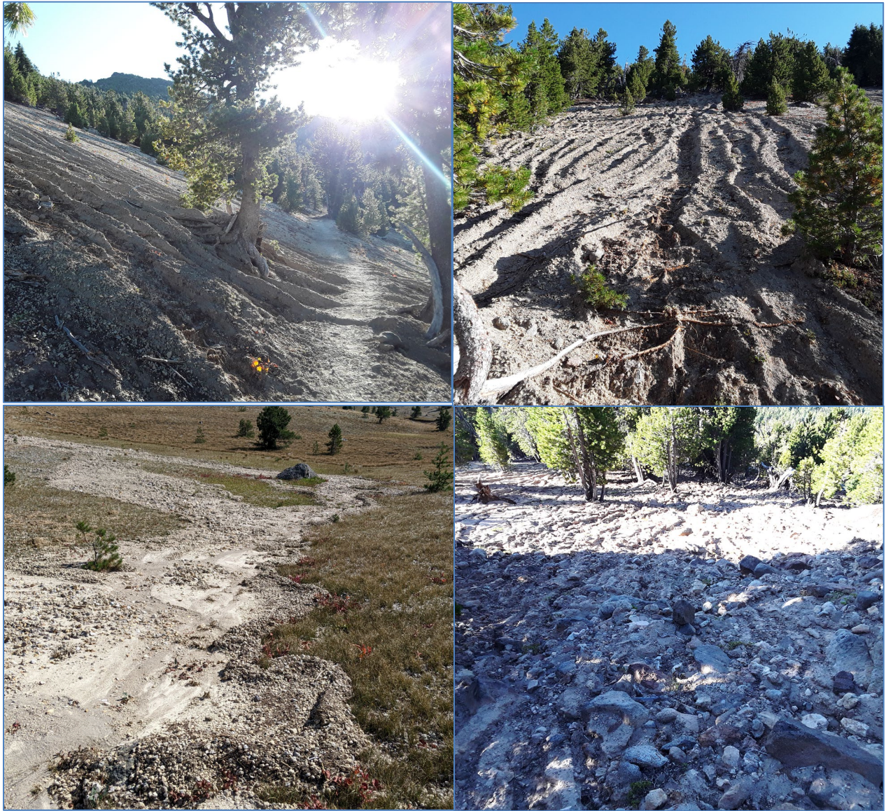
Figure 4. Erosion damage on Mt. Scott resulting from an intense monsoonal rainstorm in August 2022. Clockwise from top left: 1) deep runoff-created rills surrounding mature whitebark pine; 2) roots of mature whitebark pine exposed and abraded by runoff; 3) an area where surface runoff flows scoured away most of the upper soil layers and all understory vegetation; and 4) deposition of eroded soil particles at the base of Mt. Scott; this rock-hard crust of deposited material is several inches thick and entombs low-growing vegetation. Photos by Scott Heisler.
