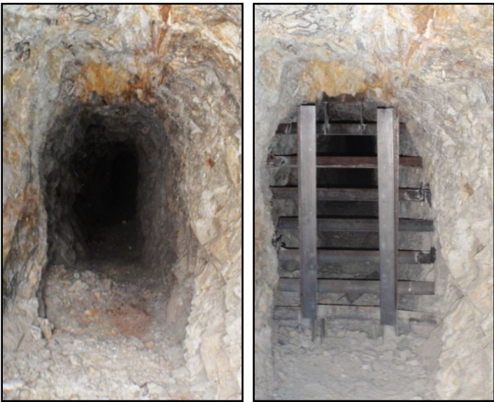
Figure 3. The open mine opening at left was sealed with a custom wildlife gate, allowing access for bats, tortoises, or other wildlife. (NPS)
