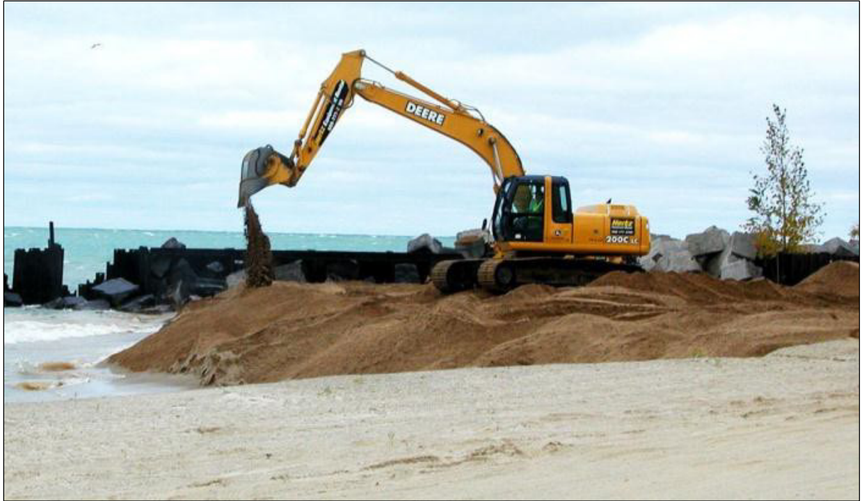
Figure 8. Excavator placing sediment along the Lake Michigan shoreline, Indiana Dunes National Lakeshore, Indiana (NPS).
