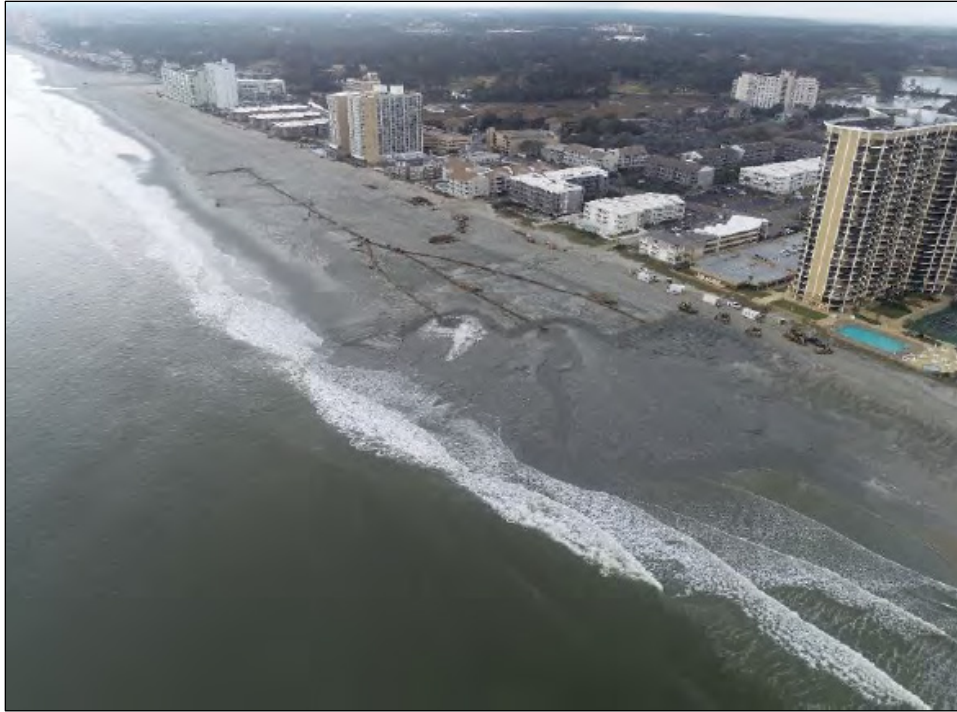
Figure C-3. Aerial of onshore beach nourishment setup depicting elbow pipe (CSE).
