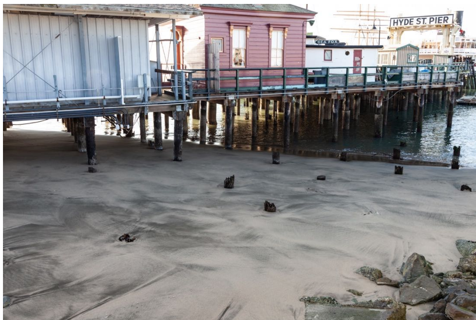
Photo 10 of 16 East side of pier at low tide, showing back of Tubbs Bldg. and stump ends of removed piles.
