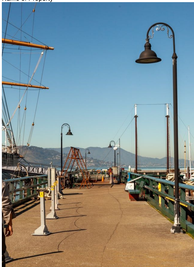
Photo 9 of 16 View northwest along main pier showing streetlights.
