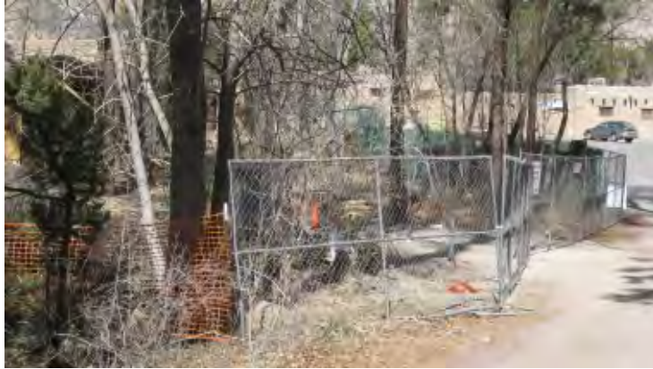
Visitor Center Rehabilitation Underway
