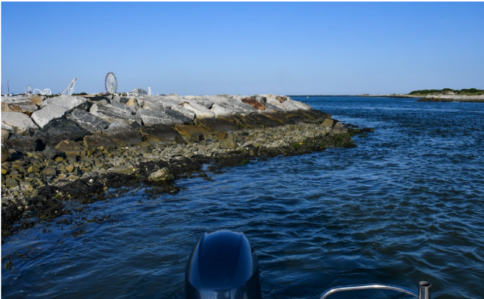
Figure B-8. ID MFB_5701 2021-07-12. Station R05-01-PRI. Typical rocky habitat consisted of Class III rip-rap jetties and armoring.
