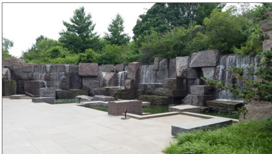
Figure 5.1. The Room 4 Fountain at the FDR Memorial. Photo taken July 14, 2014.
