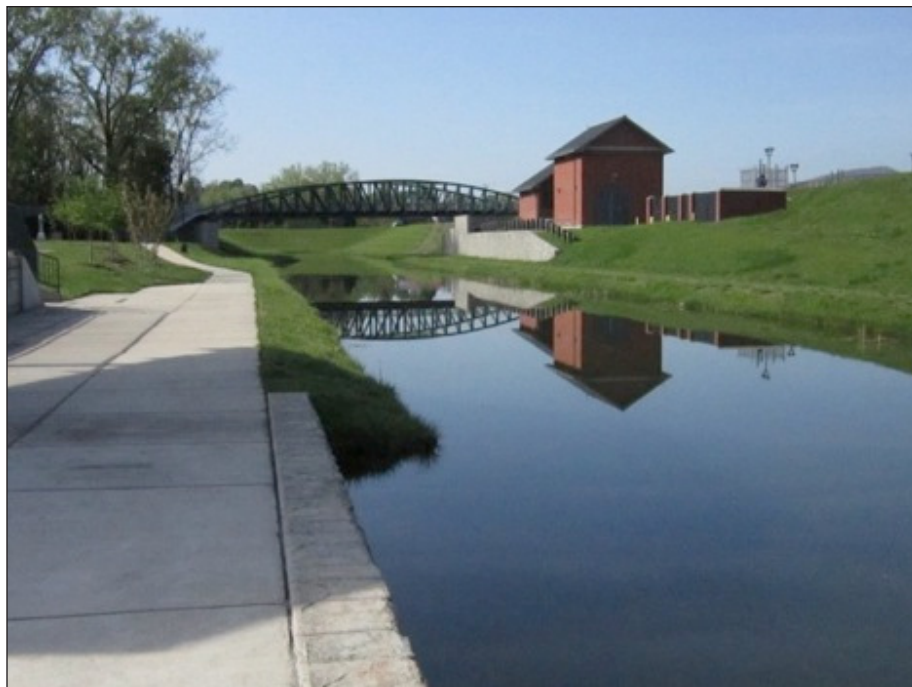
Figure 6.1. The CHOH Canal Basin at the Terminus in Cumberland, MD.
