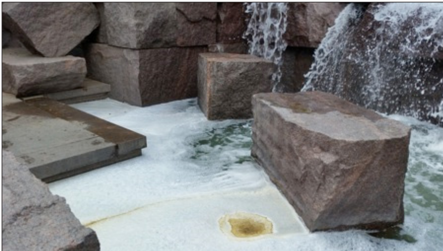
Figure 5.5. Foam across the water surface in the Room 3 Fountain on September 17, 2014.
