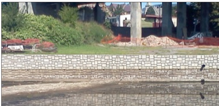
Figure 6.6. Water level in the CHOH Canal Basin. Photo taken August 26, 2014.
