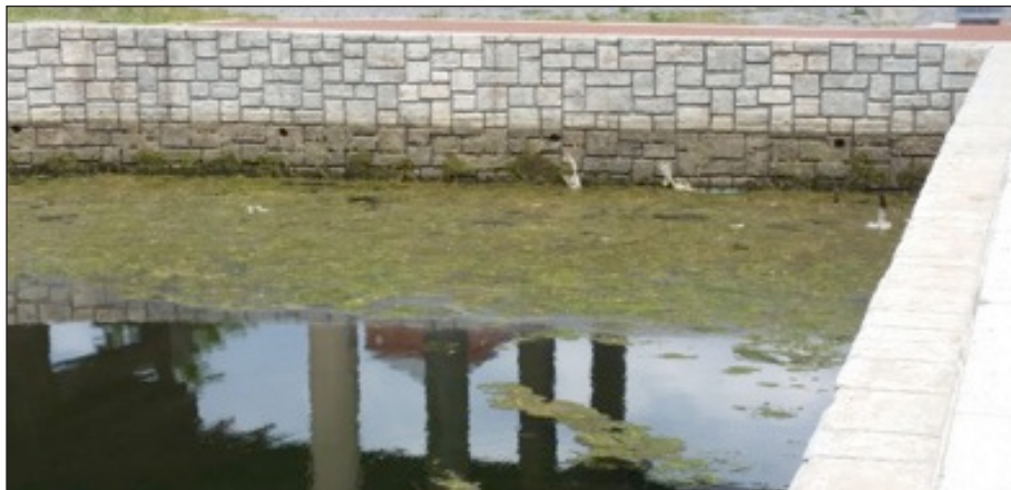
Figure 6.5. Water level in the CHOH Canal Basin. Photo taken July 8, 2014.
