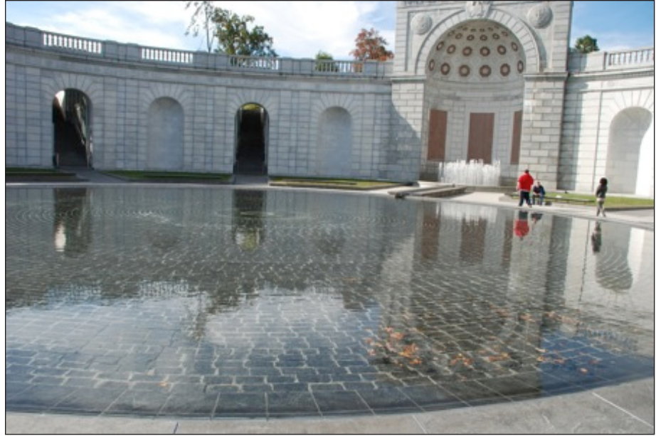
Figure 4.8. Clear water in the WIMSA Memorial reflecting pool on October 24, 2014. Note the cobble and mortar bottom structure.
