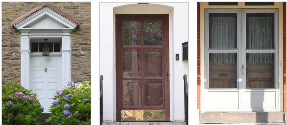
Doors and door hardware that are characteristic of a resource should be preserved. Left: Distinct panel configurations of historic entrance doors, like this eight-panel door on Harmony Hill, should be preserved. Center: The six-light configuration of this storm door on Price Street allows the historic panel configuration of the entrance door to remain visible and matches its color. Right: Mill finish aluminum storm doors that obscure the design of historic doors are not recommended.
