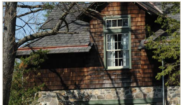
Character defining building materials of historic resources typical to East Bradford Township, such as slate shingles, log assemblies, wood shingle siding and pointed stone masonry, should be preserved.
