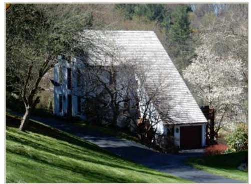
The high visibility of these two cedar shingle roofs on Harmony Hill (left) and Connor Road (right) warrants the continued use of cedar over a replacement asphalt shingle roofing.
