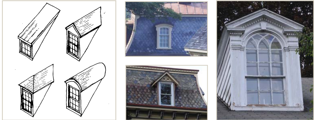
Left: Types of dormer forms include (clockwise from top left) shed dormer, gabled dormer, segmental-arched dormer and hipped dormer. Center: Decorative trim at dormers is as important as the dormer windows themselves and should be preserved. Right: In this example in East Bradford, the gothic arch light divisions of the upper sash of the dormer windows is a typical feature of the Classical Revival style.
