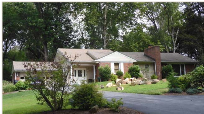
Examples of the Ranch and Split Level styles can be found in East Bradford Township on Darlington Drive off of Lenape Road.
