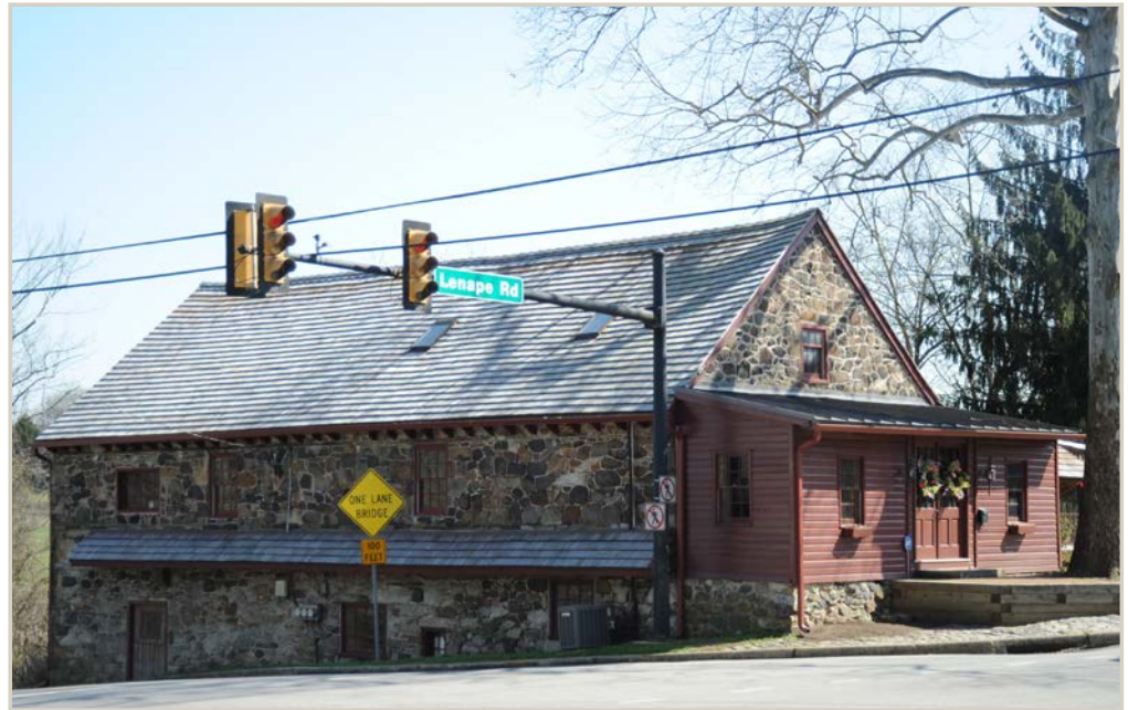
The Strode's Mill Historic District is one of the few places within the Township where building setbacks are minimal. These spatial relationships should be preserved within the District.
