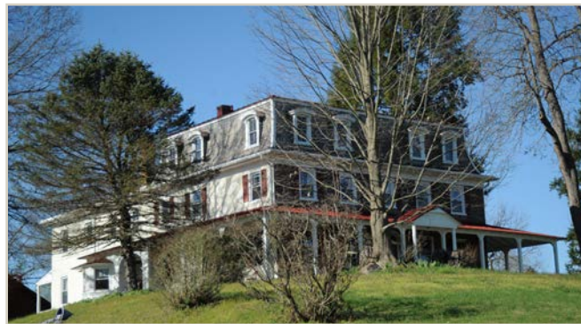
Originally constructed as a Georgian style dwelling, the 1880 addition of the Mansard roof and dormers transformed the Allerton Farmhouse to an example of the French Second Empire Style.
