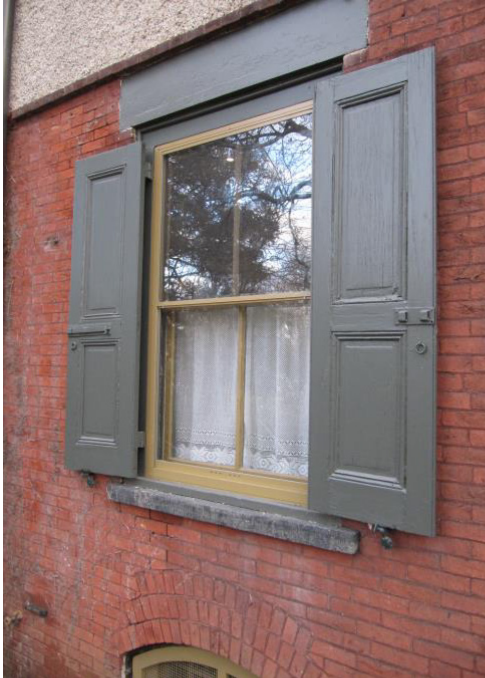
Custom color, three-track storm windows are now available as flush units that are placed in the shutter rabbet of the historic window frame.
