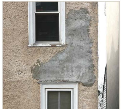
Parge-pointing on historic mill (top left); Smooth stucco patch prior to whitecoat (top right); Heavily textured or swirled stucco is inappropriate (bottom left); Inappropriate stucco patch (bottom right).
