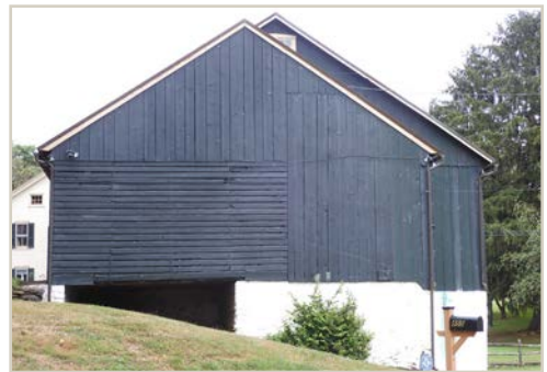
Left: It is common that wood siding for primary buildings is horizontal clapboarding, while outbuildings are more likely to have vertical board siding. Above: Patterns of historic vertical and horizontal siding should be preserved.
