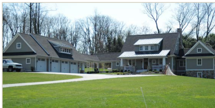
Successful new construction in the Taylor-Cope Historic District has been set back from the street and continued a rhythm that does not compete with the existing forms of the district.
