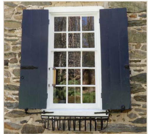
Traditionally shutters were paneled on the first floor (left) and louvered blinds on the second floor. Less often, they were made of boards (right). Where possible, old shutters should be retained and restored, or if necessary, replaced in kind.
