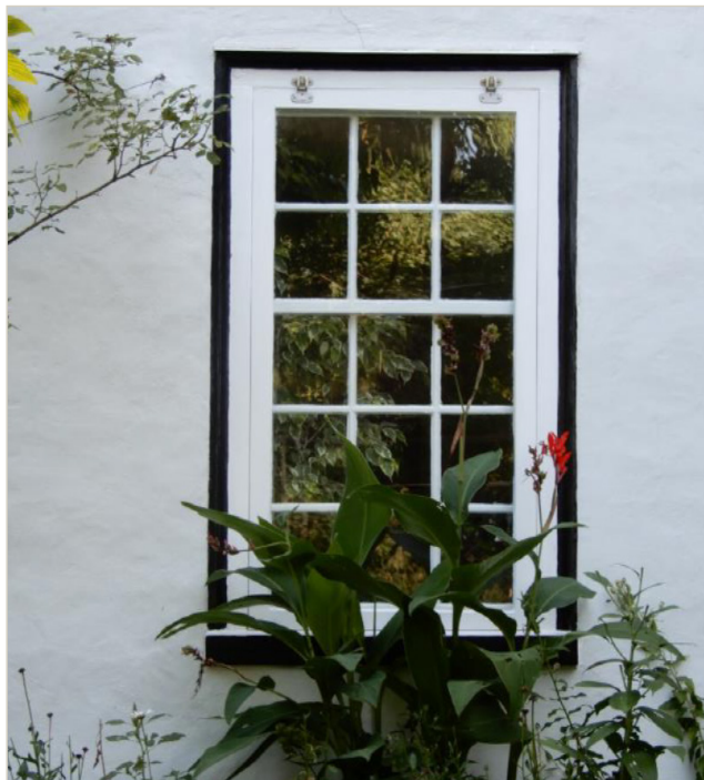
Historic storm windows like this one were made of wood and were removed seasonally.
