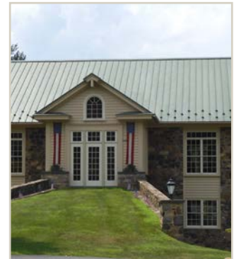
Historic and replacement standing seam metal roofing can be seen on many historic resources in East Bradford.
