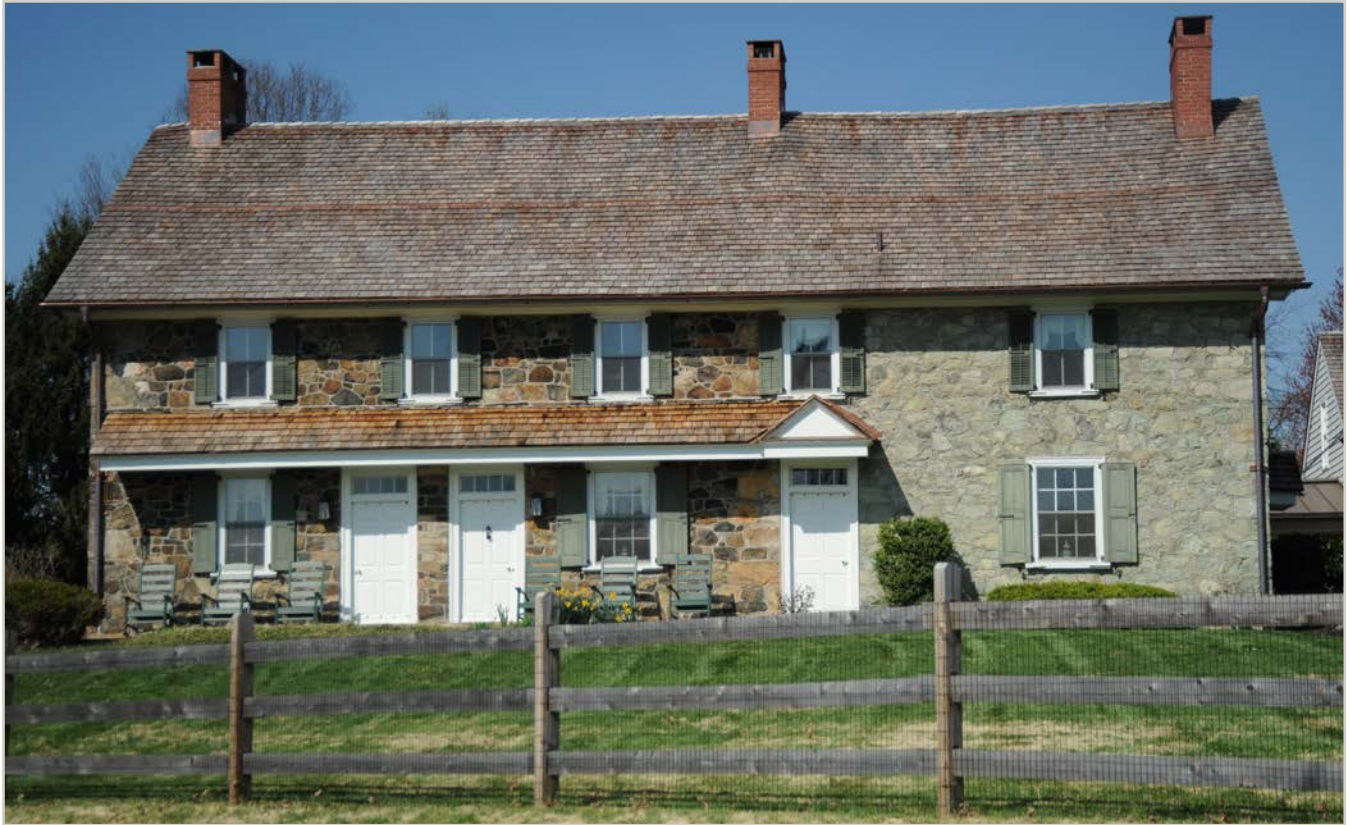
Many buildings in East Bradford Township, including this resource on Birmingham Road in the Strode's Mill Historic District, were added to very early. These additions are significant changes that should be preserved. In this example, the two-bay serpentine stone wing on the right was added to the original three-bay stone farmhouse in 1800.
