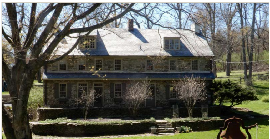
Retaining existing slate roofing is highly encouraged, particularly in highly visible locations like the Mansard roof on Allerton Road and the steeply pitched gable along Copeland School Road.
