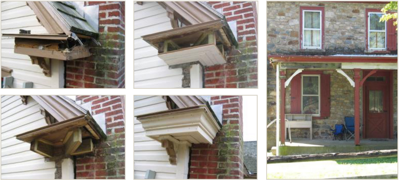
Left & Center: Sequence of restoration of a severely deteriorated cornice return. The crown molding was custom-cut for the project, a procedure that requires scheduling but does not add significantly to the repair cost. Right: Repair, restoration or replicate components should be employed when character defining features like porch posts and brackets are deteriorated, as seen here at this in- progress restoration.
