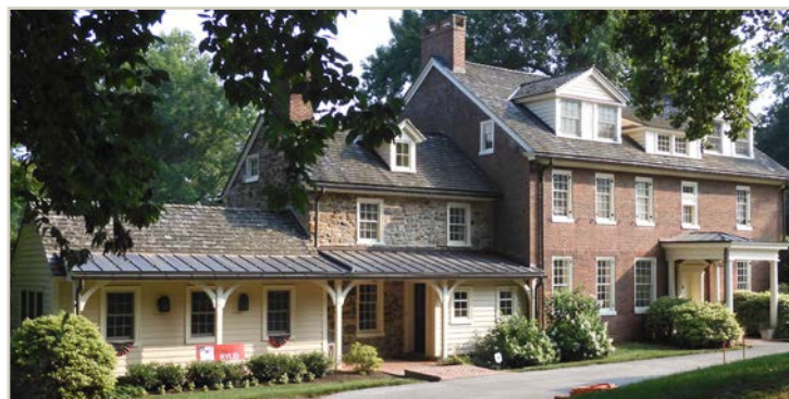
The compatible additions to the historic core of the Townsend Farm Main House repeat the gabled roof form parallel to Hillsdale Road.
