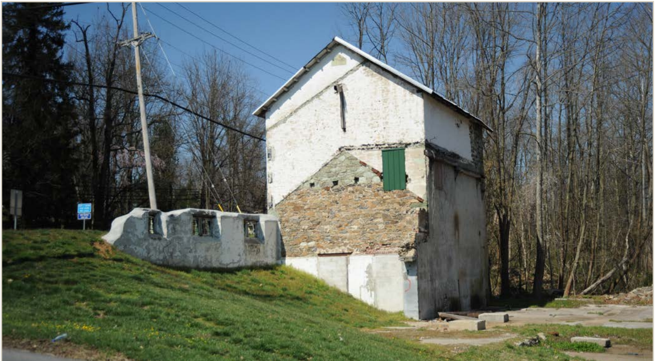
Strobe's Barn, Strobe's Mill Historic District.
