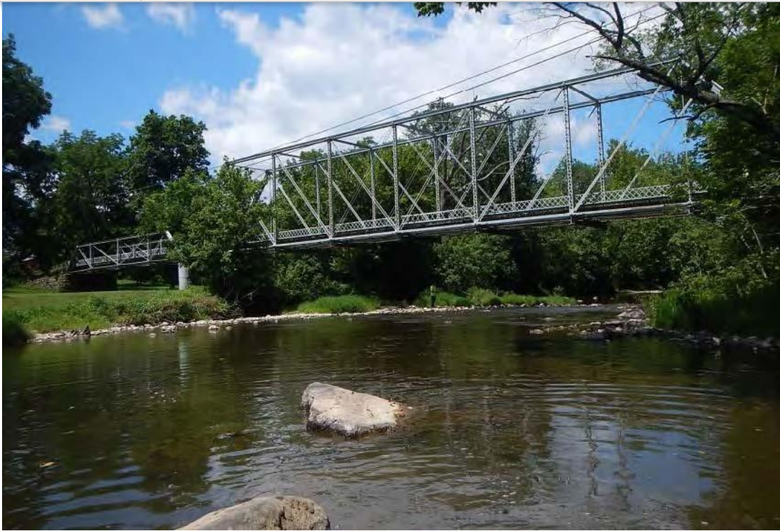
Hull Drive Bridge over Bermudian Creek.
