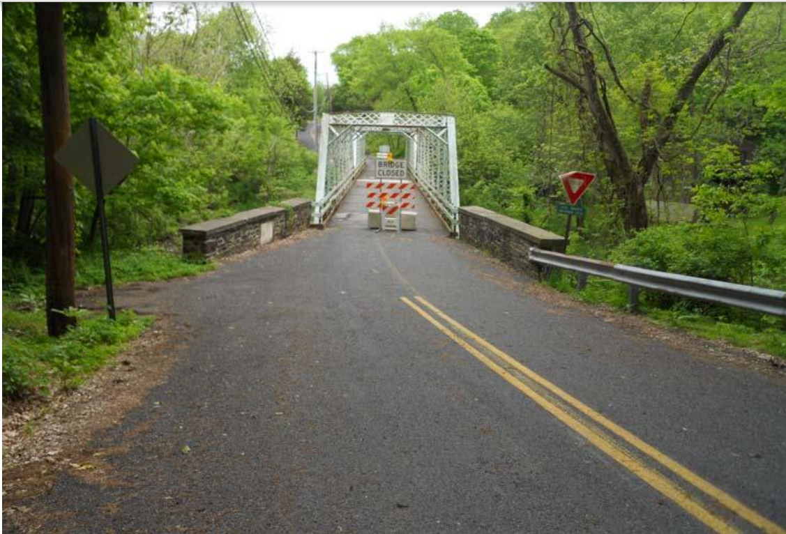
Bergey's Mill Road Bridge in Lower Salford Township, Montgomery County. Image courtesy of PennDOT.
