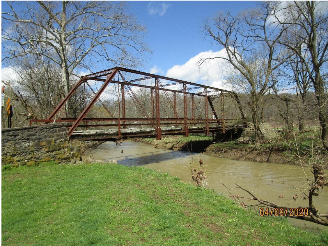
Hodgens Bridge in Blaine Township, Washington County. Source: PennDOT inspection Records.
