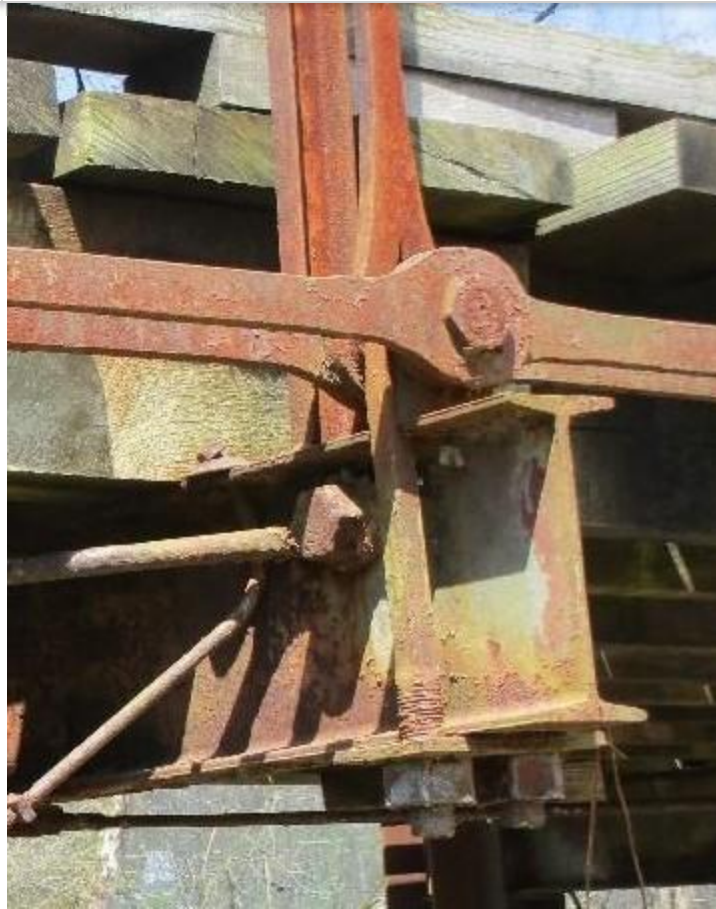
Pin Connection on the Hodgens Bridge. Source: PennDOT inspection Records.
