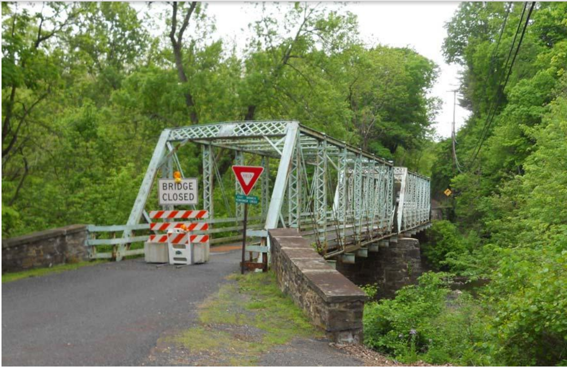
Bergey's Mill Road Bridge in Lower Salford Township, Montgomery County. Image courtesy of PennDOT.
