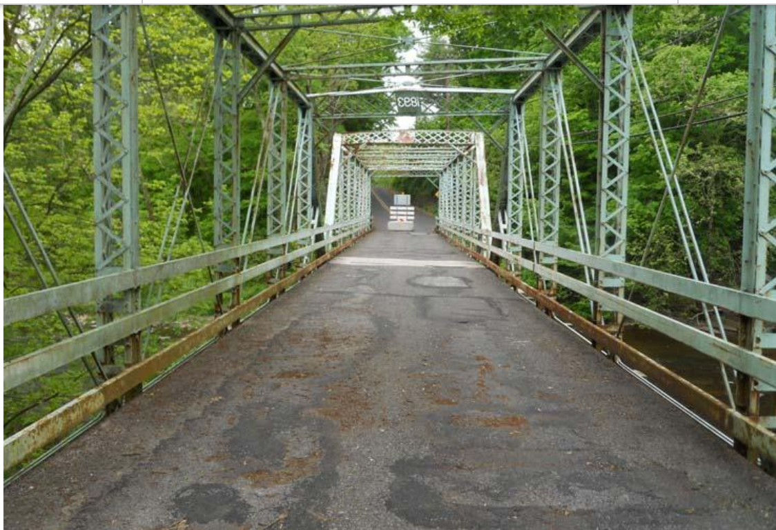
Looking through the two spans of Bergey's Mill Road Bridge in Lower Salford Township, Montgomery County. Image courtesy of PennDOT.
