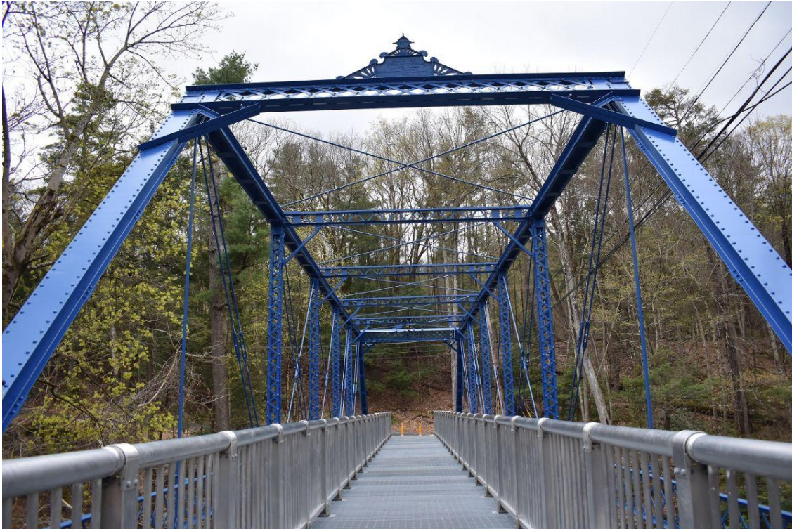
Mott Street Bridge after rehabilitation was complete.
