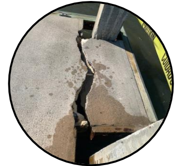
Damage to the Kingsley Plantation dock from high storm waves (NPS)
