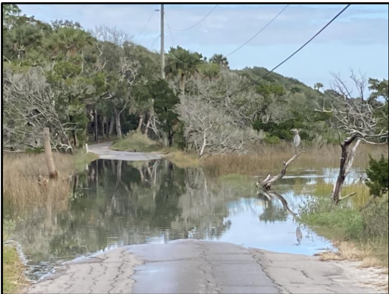
This image shows sunny day, high tide flooding of the road that leads to Kingsley Plantation, which is one of the most popular visitor locations at the preserve (NPS)
