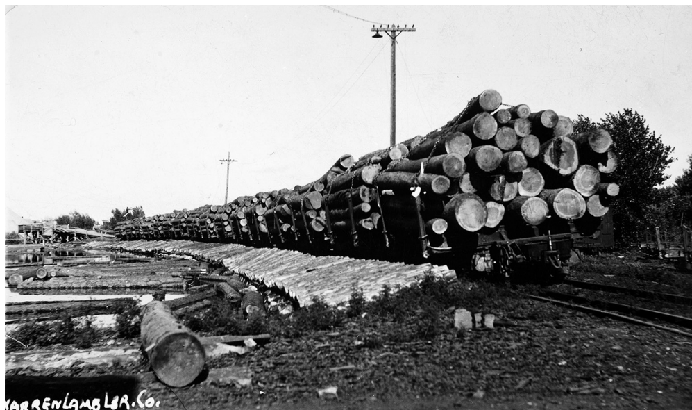
Facilities near Cowboy Hill, such as the one pictured here, processed timber from the Black Hills. The lumber industry thrived in the area from the 1910s to the 1960s.
