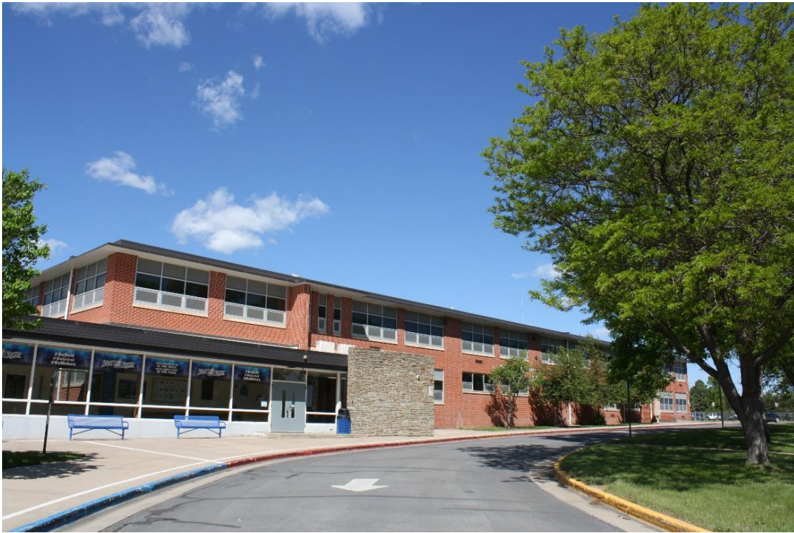
West Junior High School main façade looking northwest
