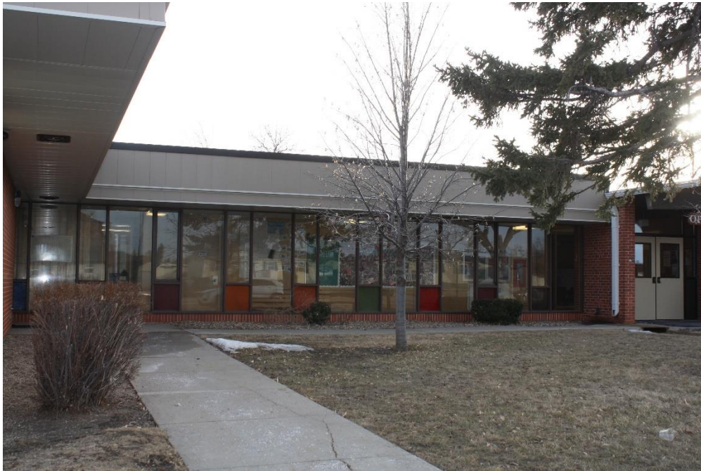
Knollwood Elementary looking southwest at window wall corridor
