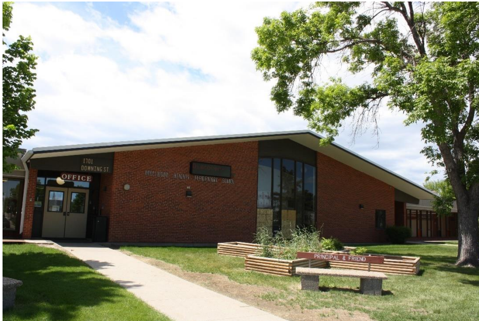
Knollwood Elementary School main entry bay looking southwest
