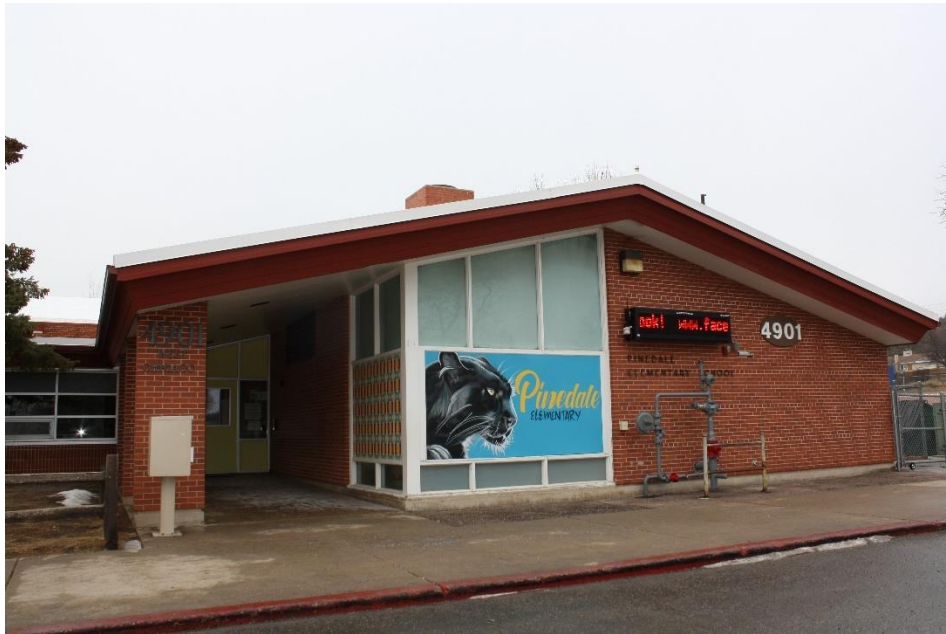
Pinedale Elementary School main entry bay looking south
