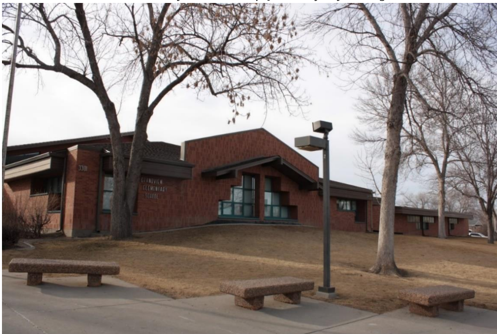
Grandview Elementary School main façade entry bay looking northwest
