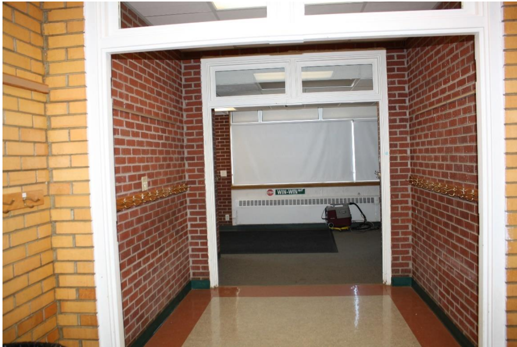
Transition between original building and 1963 addition.
