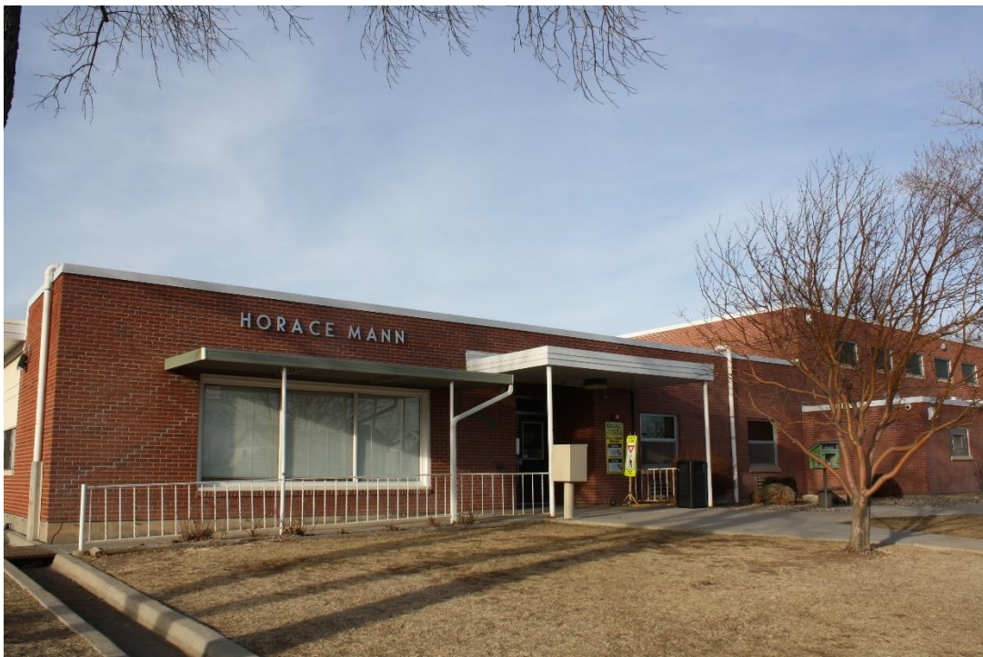
Office/main entrance at west end of south façade looking northeast.
