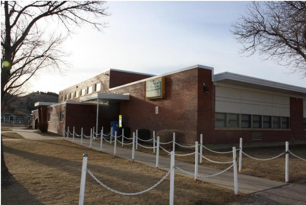
South and east elevations looking northwest
