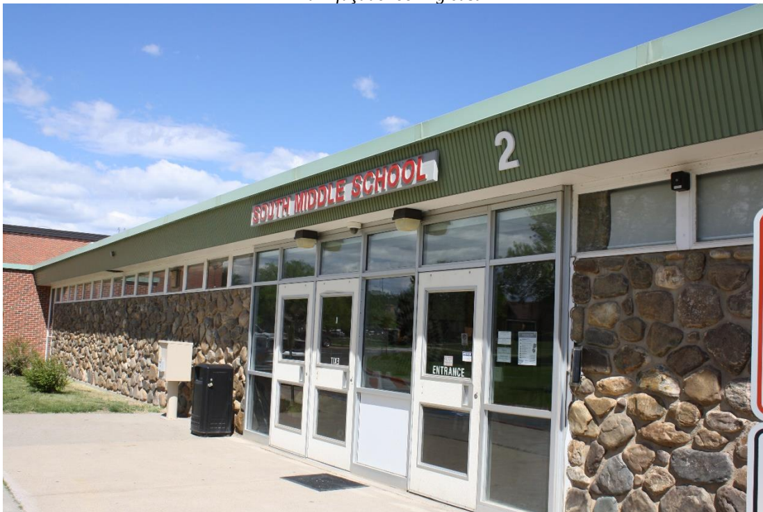
Detail of main entry doors
