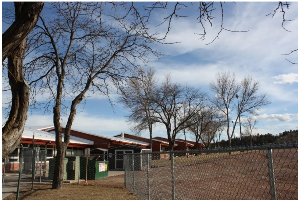
Pinedale classrooms and additions looking southeast
