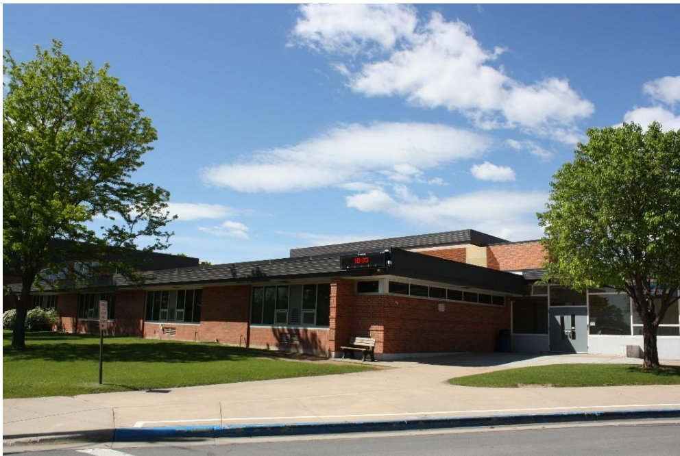
East façade cafetorium addition looking southwest
