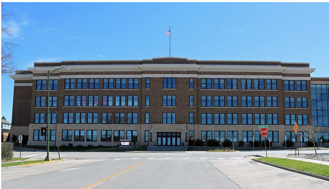
Figure 8. The former Rapid City High School, built in 1923 was listed in the National Register of Historic Places in 2010 for its historical and architectural significance. It served as the only Rapid City high school from 1937 through 1969 when Steven's High School was built. Photo: Author, June 2022.
