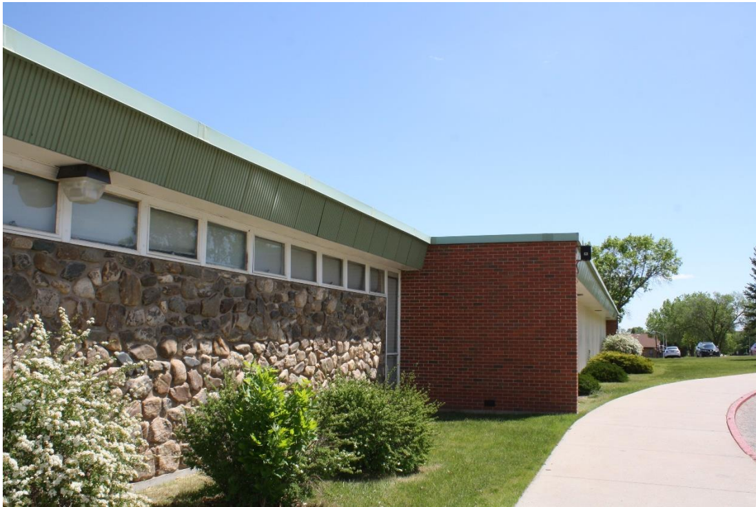
Main façade looking east
