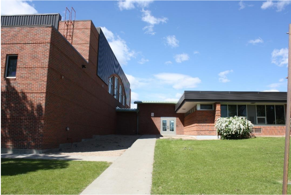
East façade looking west at connection between school and community center.
