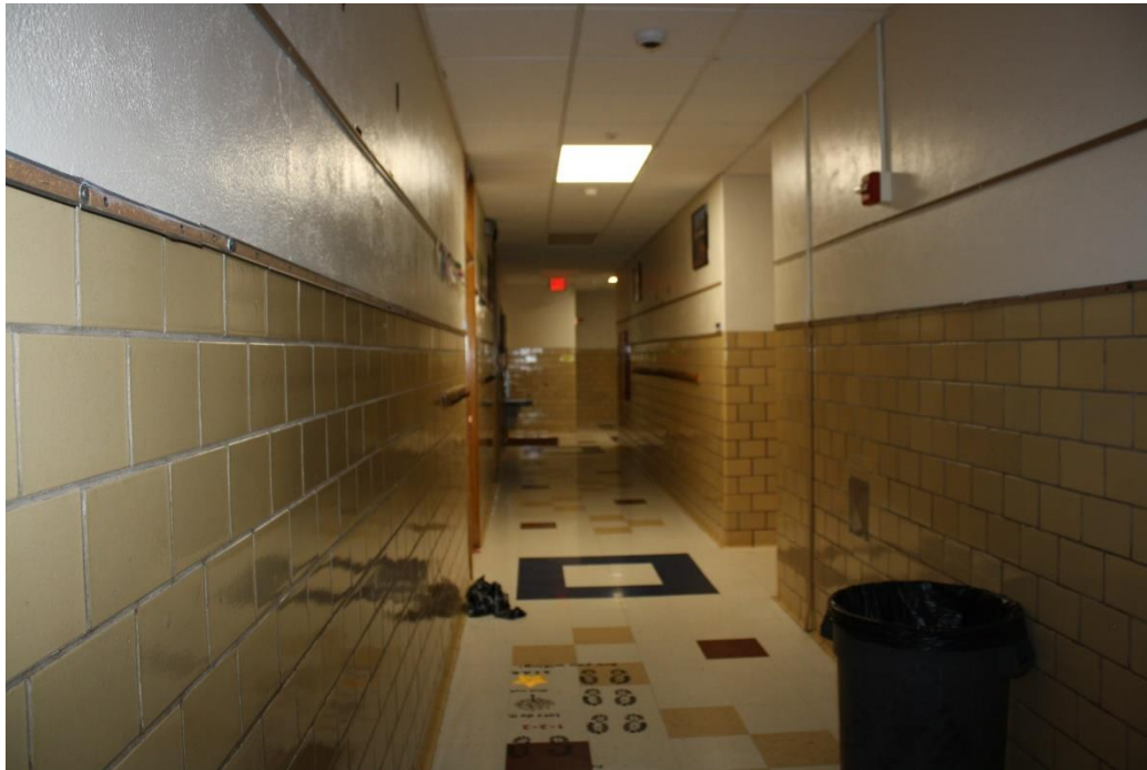
Corridor with glazed block walls and tile floors
