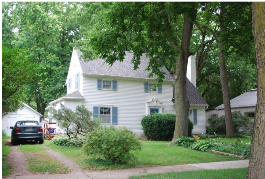
Photo #12: 110 S. Yale St. [SD_Clay County_Jolley Historic District_0012] West façade (right) and north elevation (left), with garage, camera facing southeast
