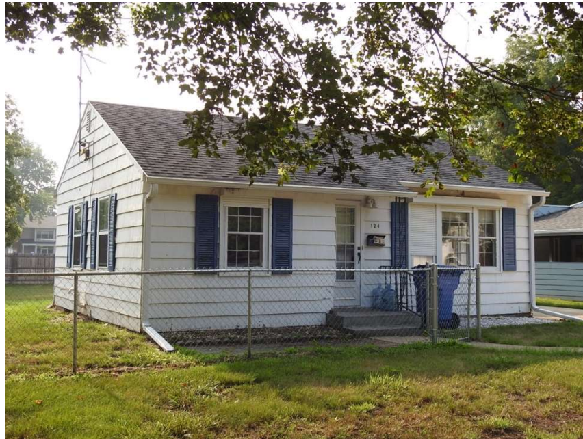
Photo #21: 124 S. Pine St. [SD_Clay County_Jolley Historic District_0021] West façade (right) and north elevation (left), camera facing southeast
