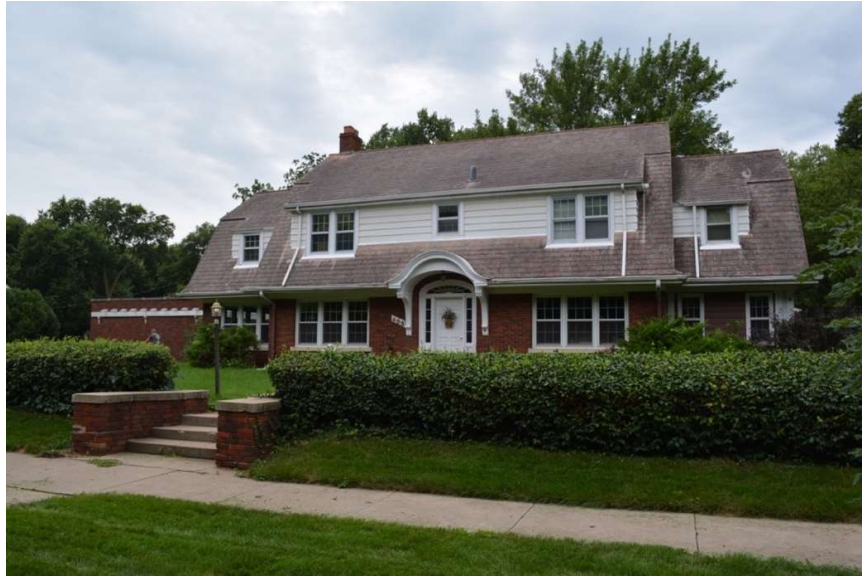
Photo #9: 405 S. University St. [SD_Clay County_Jolley Historic District_0009] East façade, camera facing west
