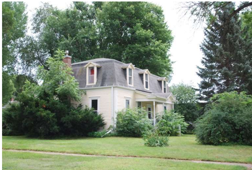
Photo #2: 104 S. Harvard St. [SD_Clay County_Jolley Historic District_0002] West façade (right) and north elevation (left), camera facing southeast
