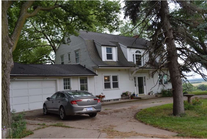
Photo #11: 401 Park Lane. [SD_Clay County_Jolley Historic District_0011] North façade (right) and east elevation (left, with garage), camera facing southwest
