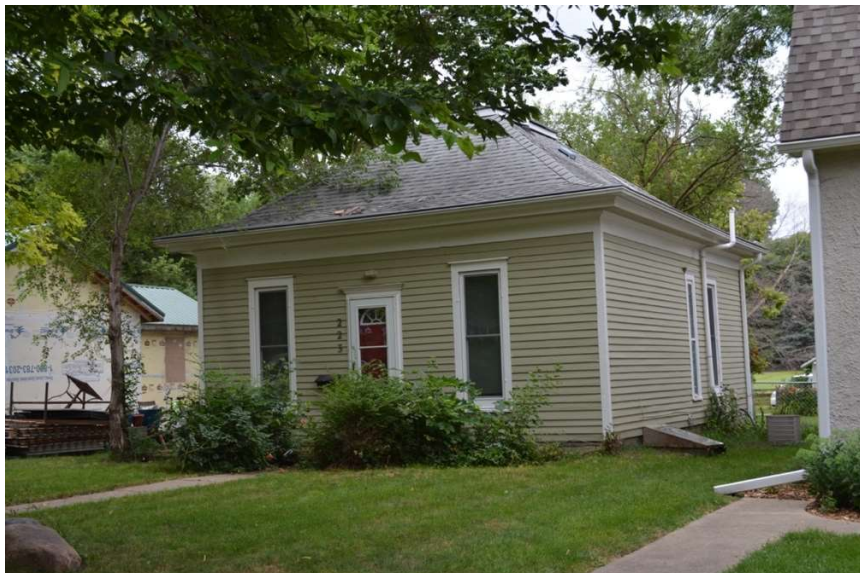
Photo #28: 223 S. Yale St. [SD_Clay County_Jolley Historic District_0028] East façade (left) and north elevation (right), camera facing southwest
