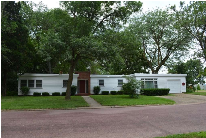
Photo #18: 405 Canby St. [SD_Clay County_Jolley Historic District_0018] North façade, camera facing south
