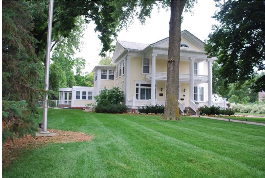
Photo #5: 415 E. Main St. [SD_Clay County_Jolley Historic District_0005] North façade (right) and east elevation (left), camera facing southwest
