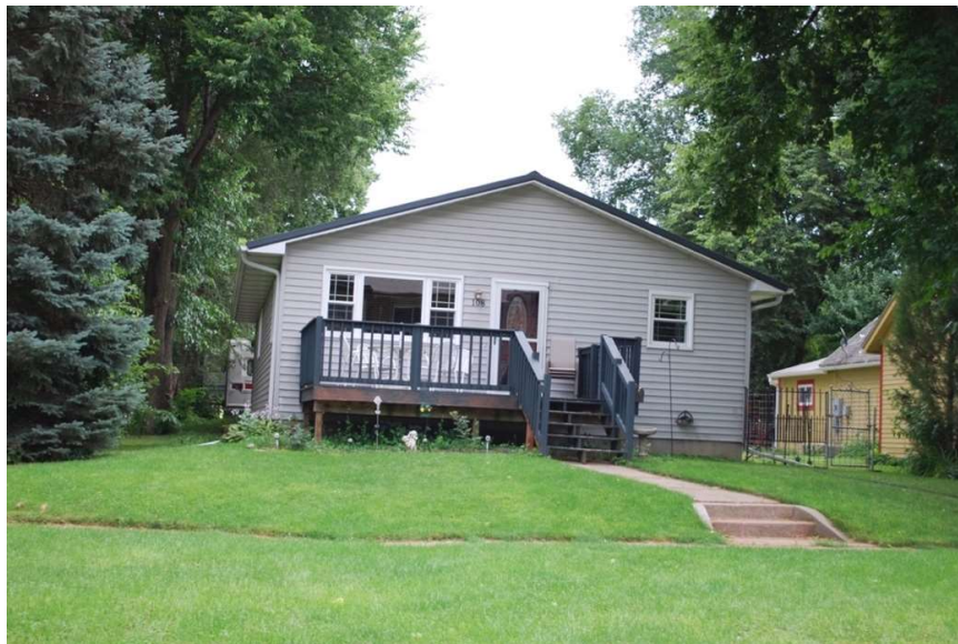
Photo #36: 108 S. Harvard St. (Non-Contributing) [SD_Clay County_Jolley Historic District_0036] West façade, camera facing east
