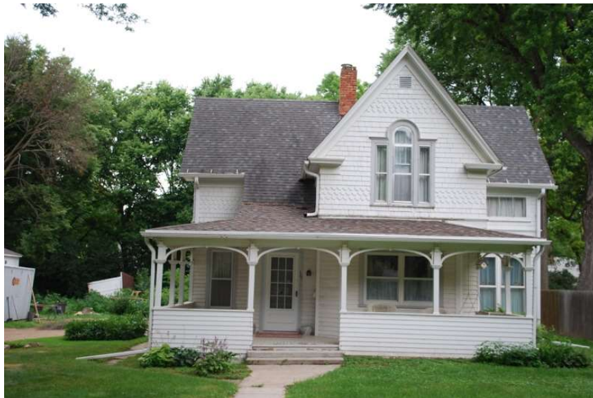
Photo #4: 101 S. University St. [SD_Clay County_Jolley Historic District_0004] East façade, camera facing west
