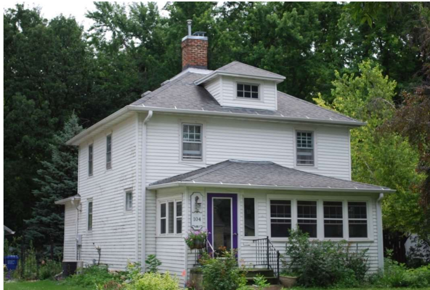
Photo #29: 104 S. Yale St. [SD_Clay County_Jolley Historic District_0029] West façade (right) and north elevation (left), camera facing southeast
