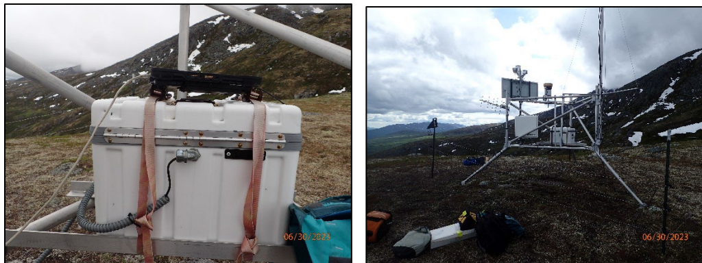
Figure 7. Ruth Glacier climate station June 30, 2023. Power cable before it was replaced (left) and station at end of site visit (right).
