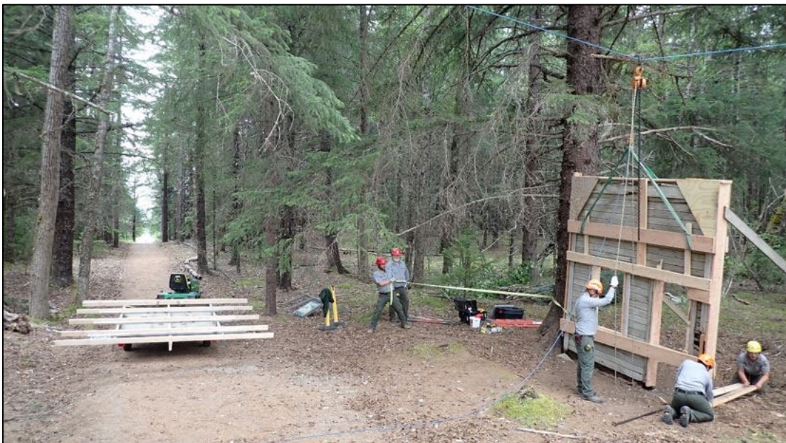
Figure 9. Area between trail and False Front relocation site cleared of invasive plants, with KLGO maintenance team installing the artefact. (NPS)
