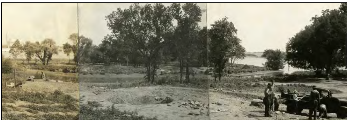
FIGURE 42: CCC Members Working on the Overlook Terrace, July 1935 (JM&T 2018)
