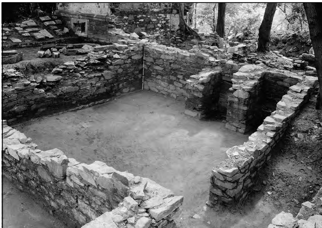
FIGURE 44: The Mason House Under Excavation, 1936 (Library of Congress 1936)
