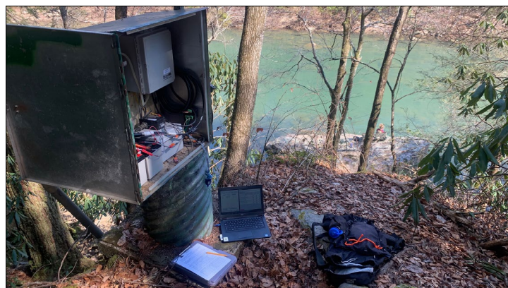
Site visit to Clear Fork Creek. NPS photo / APHN staff.
