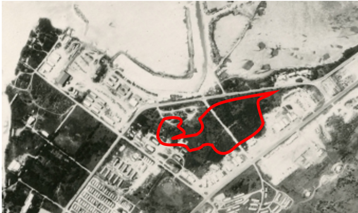
Figure 2. Aerial photo dated July 1949 showing structures and roads within the area now designated as the mangrove wetland, and an approximate historical extent of the mangrove wetland (red line) as described by Prasad (1997).
