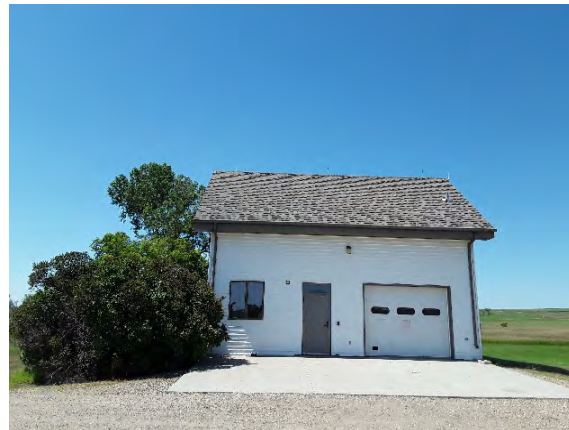
2022_KNRI_66832_Maint. Office Building_Front.jpg
