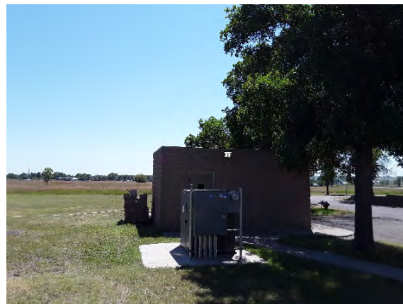
2022_KNRI_66811_Tractor Storage Building_Front.jpg
