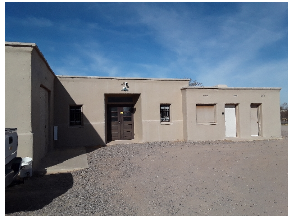
2021_CAGR_40384_B-9 Maintenance Office_Front.jpg
