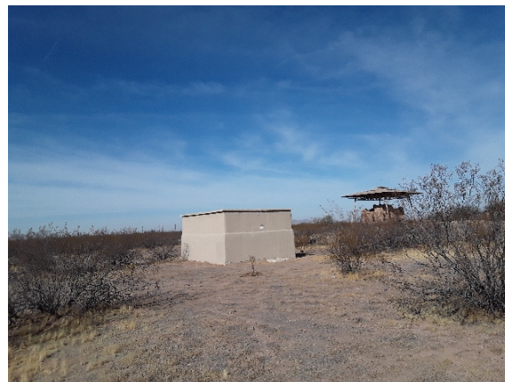
2021_CAGR_not found _Pumphouse_Front.jpg
