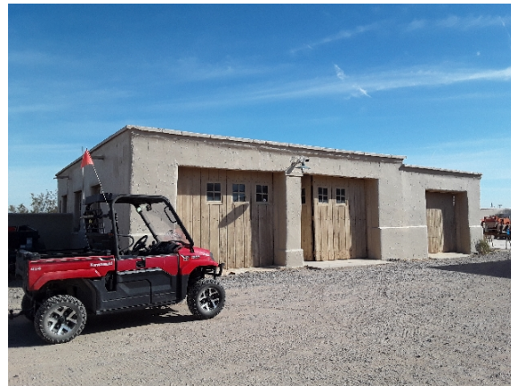
2021_CAGR_40390_B-11 Maintenance Shop_Front.jpg
