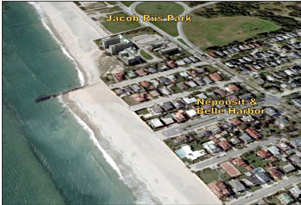
Figure 7. Groin between the Neponsit & Belle Harbor communities and Jacob Riis Park, both part of Gateway National Recreation Area, causing sediment accumulation on the updrift side and erosion and inland beach displacement on the downdrift side. Aerial image accessed February 2010. (Source: bing.com/maps/ )
