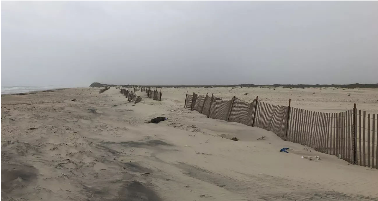
Figure 6. Silt fence installed in 2021 near transect 109 to trap sediment at a washover zone that was breeched by Hurricane Hanna.
