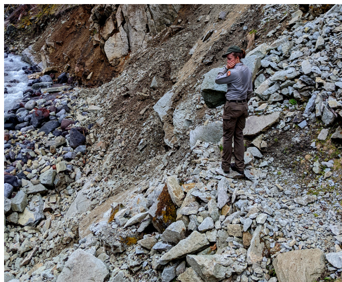
Figure 2. Damage on the Wonderland Trail from the storm (NPS photo).
