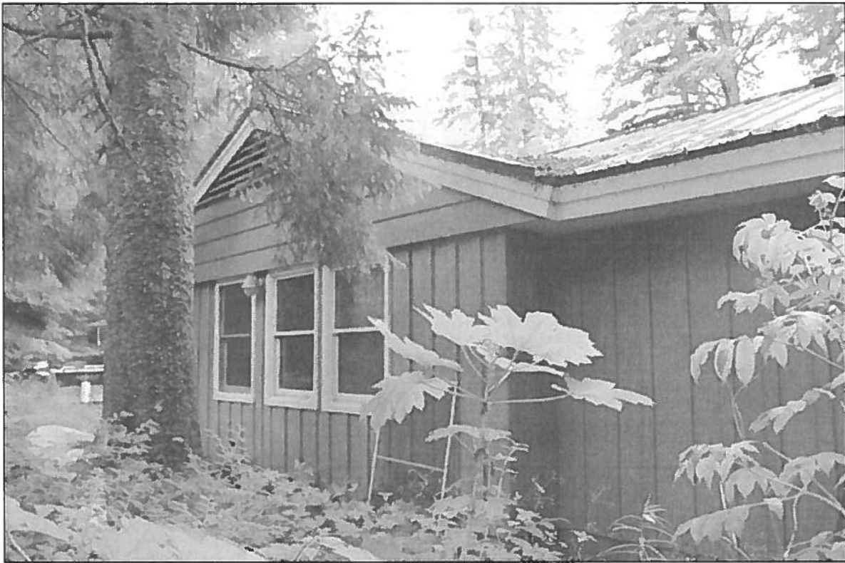
Photo 6: GBQ-5 Residence, Northeast Elevation facing southwest.
