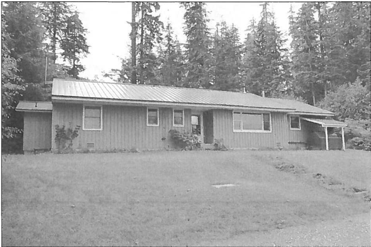
Photo 8: GBQ-3 Residence, Northwest Elevation facing southeast.
