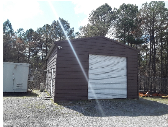
2022_LIRI_104050_LIRI Fire Building & Gym_Front.jpg
