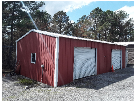
2022_LIRI_97577_RT and Fire Building_Front.jpg
