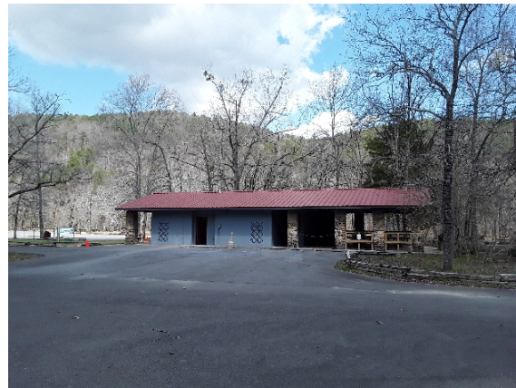
2022_LIRI_66396_CMP Multi-Use Facility_Front.jpg
