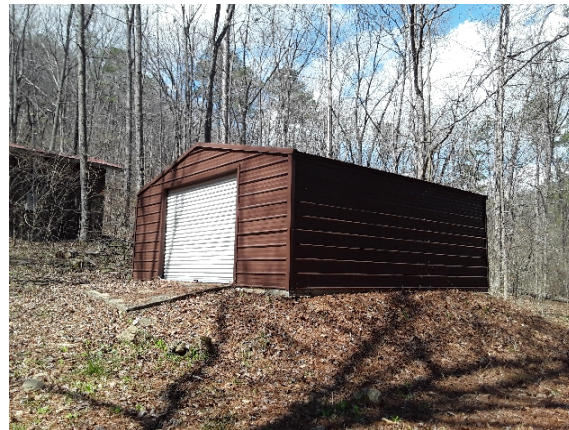
2022_LIRI_227444_CMP Storage Building_Front.jpg
