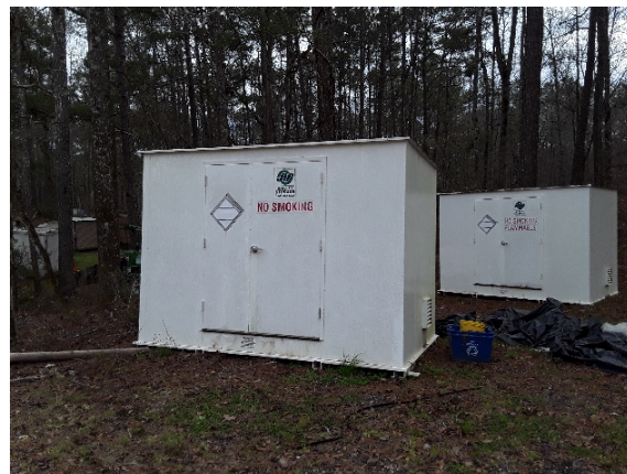
2021_HOBE_not found _HAZMAT storage 1_Front.jpg
