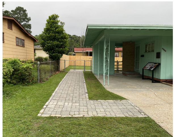
FIGURE 3–25. The stone paver path extends parallel to the carport to the rear entrance (source: DHM Design, 2023).
