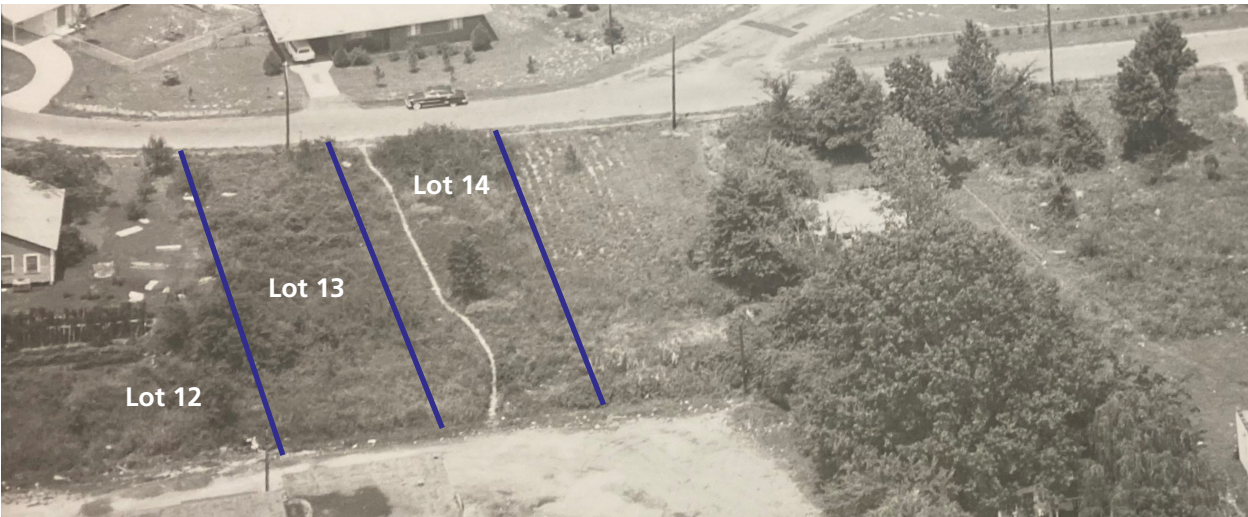
FIGURE 4-2. Birds-eye view of the Missouri Street Lots (separated as 12, 13, 14 in purple), circa 1963. This photo partially shows the residence on Lot 12, which was razed in the mid-1970s (source: Photograph in Box 221, DeLaughter Collection, Mississippi Department of Archives and History).
