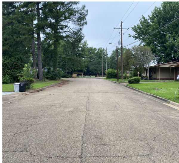
FIGURE 3-22. Margaret W. Alexander Drive is defined by concrete curb and gutter on both sides (source: DHM Design, 2023).
