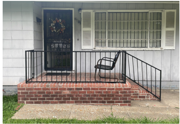
FIGURE 5–4. The wrought iron handrail and the brick stoop above are examples of features within the Medgar Evers Historic District which reflect its historic character. Future additions within the district should be compatible with existing features (source: NPS, 2024).
