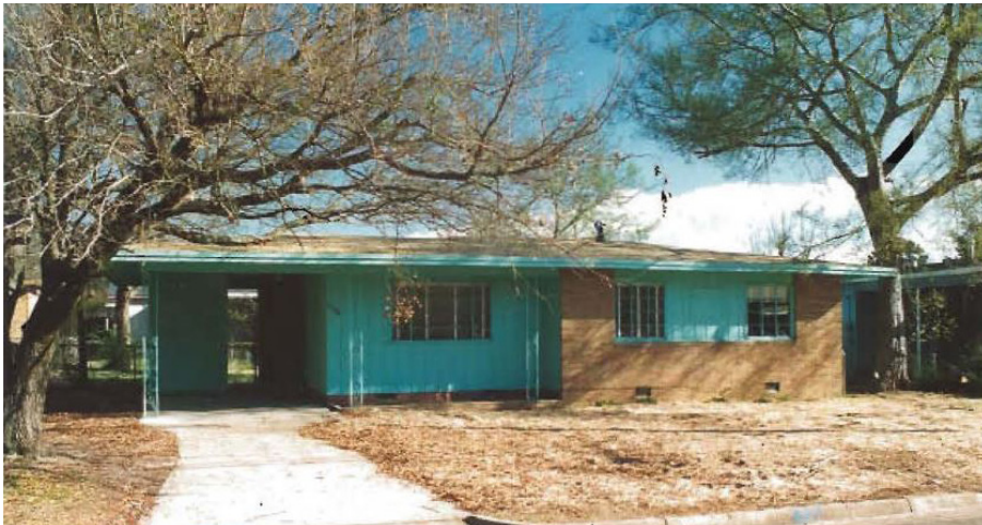
FIGURE 4-31. Mature vegetation, including the live oak before it was transplanted (left), 1996 (source: WFT Architects, 1995 HSR).
