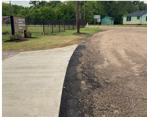
FIGURE 3–27. The concrete apron provides vehicular access to the Missouri Street Lots (source: DHM Design, 2023).
