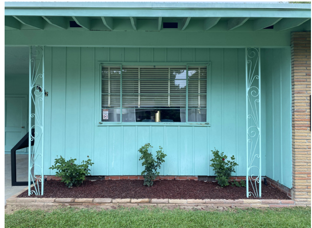
FIGURE 5–5. Decorative wrought iron and brick planters, depicted here at the Medgar and Myrlie Evers House NHL, are prominent character-defining features in the Medgar Evers Historic District (source: DHM Design, 2023).
