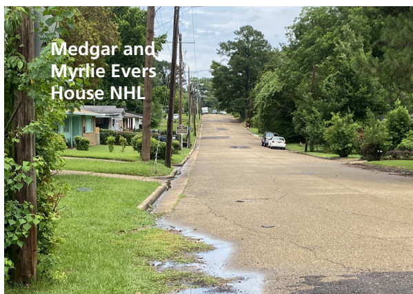
FIGURE 3-8. The road slopes to a low point at the drainage and sewer overflow channel (source: DHM Design, 2023).
