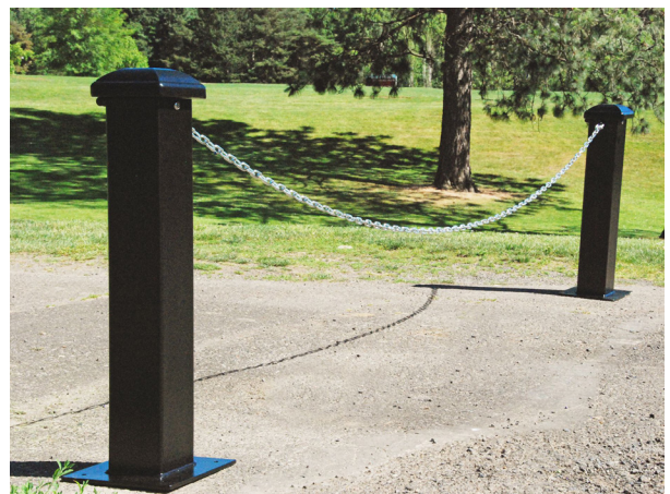
FIGURE 5–9. Example of a non-permanent, compatible post and chain barrier to prevent non-NPS vehicles from entering the driveway (source: drivewaylocker.com ).
