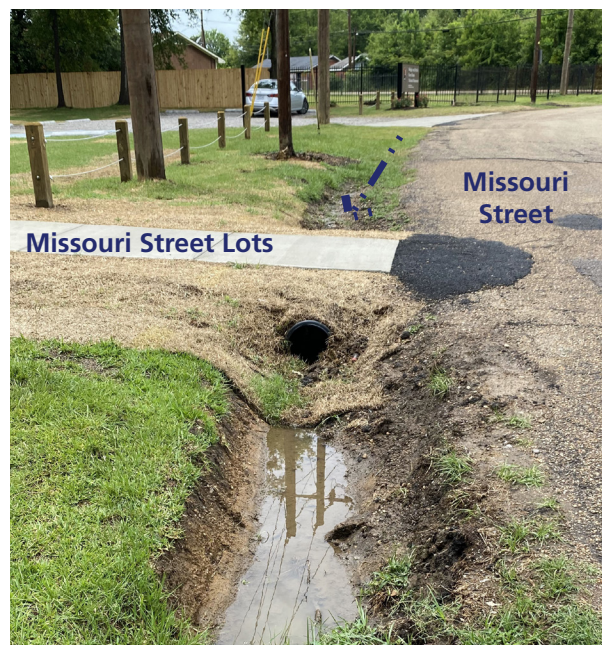
FIGURE 3–13. The constructed grass swale follows the edge of Missouri Street and has connecting culverts at driveway and walkway crossings (source: DHM Design, 2023).
