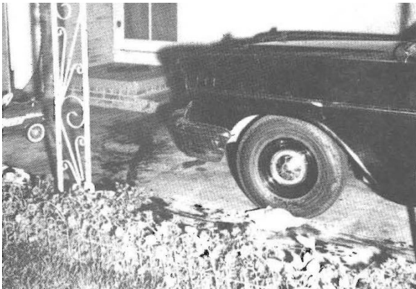
FIGURE 4-21. Fenced perennial bed replaced the medium flowering shrubs at the carport by 1963. Photo taken in 1963 (source: 1995 Historic Structures Report).
