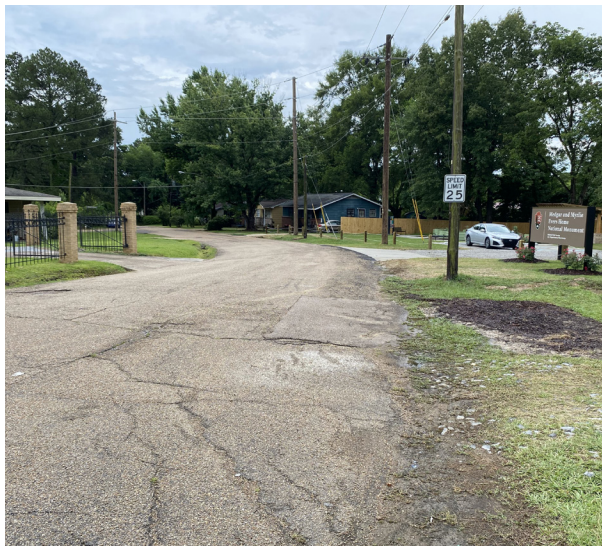
FIGURE 3-21. Missouri Street does not have sidewalks or curbs on either side of the road (source: DHM Design, 2023).
