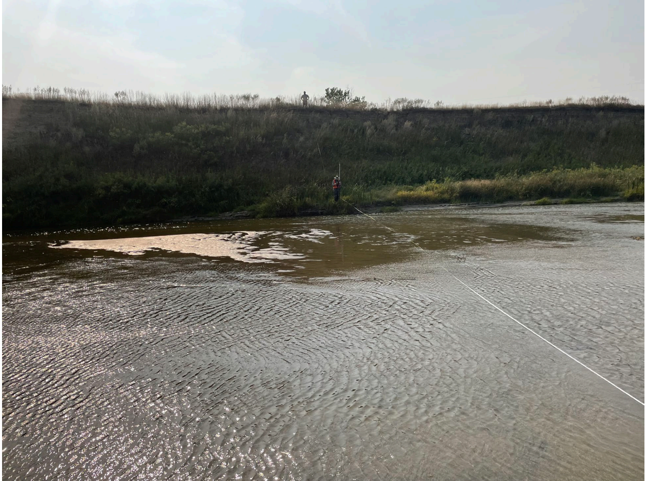
Figure 6. KNRI stream channel monitoring site SCM 001 at T11 (upstream) end. Despite the high banks (8m), the bank is largely covered in vegetation and has a small floodplain forming atop eroded material at the base. It scored a 15 on BSI index for bank instability (“unstable”). Good access to the floodplain is available on the left bank.
