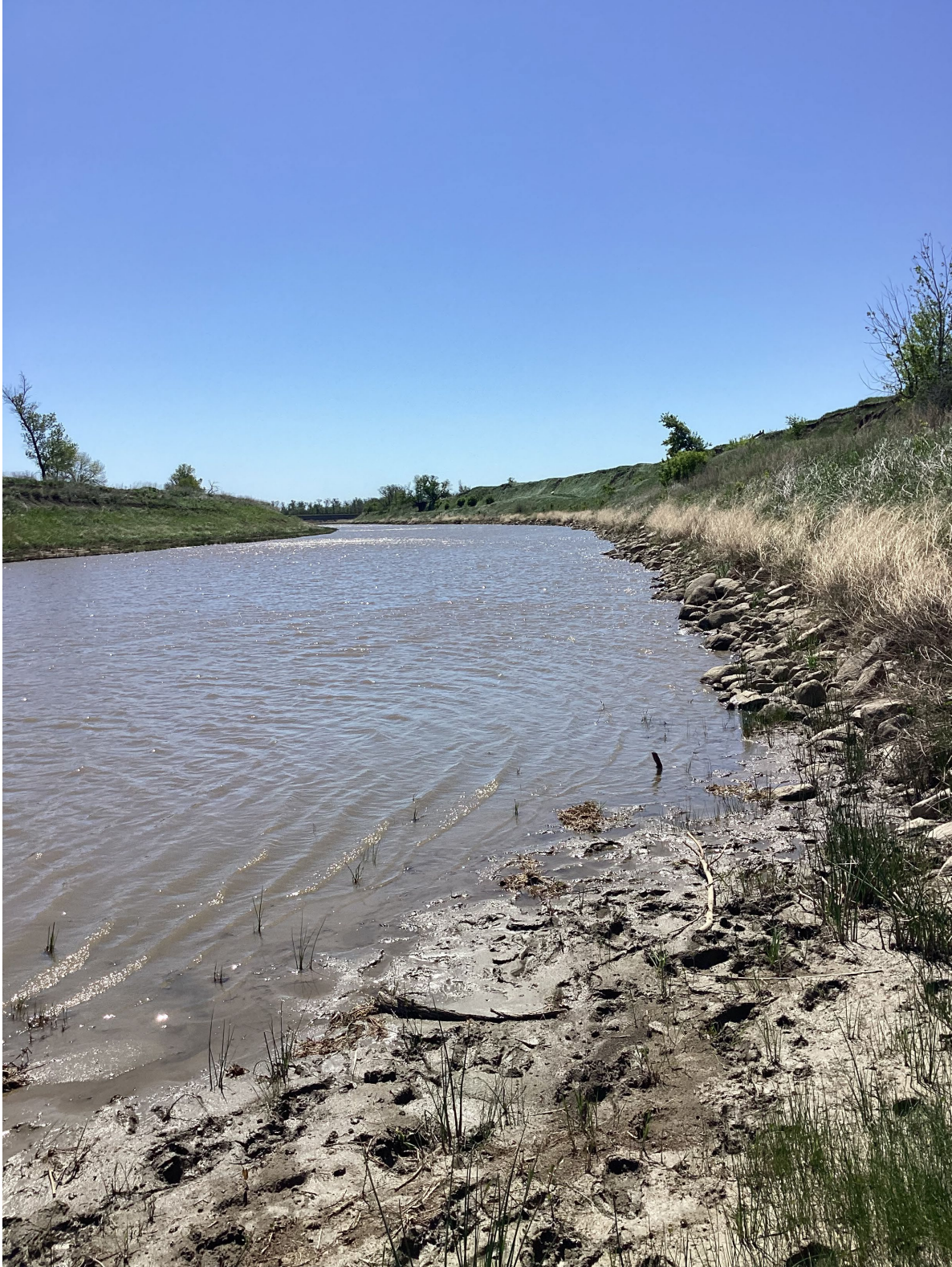
Figure 12. Restabilized base of right bank (outside bend) looking downstream toward T1. Note silt clay substrate, cobble-sized rock and vegetation stabilizing the lower bank.
