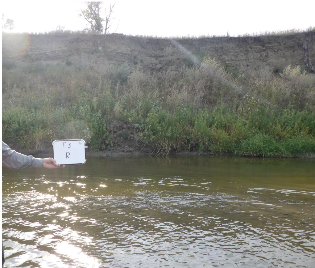
Figure 5. KNRI stream channel monitoring site SCM 001 at T3 (downstream) end. This is one of the fastest eroding banks on Unnamed Bend according to Sexton 2012 while it had a moderate BSI score for bank stability (11.5).
